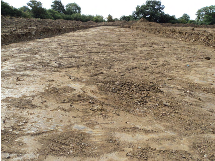
Plate 3. View of Stripped Area. Facing South.
