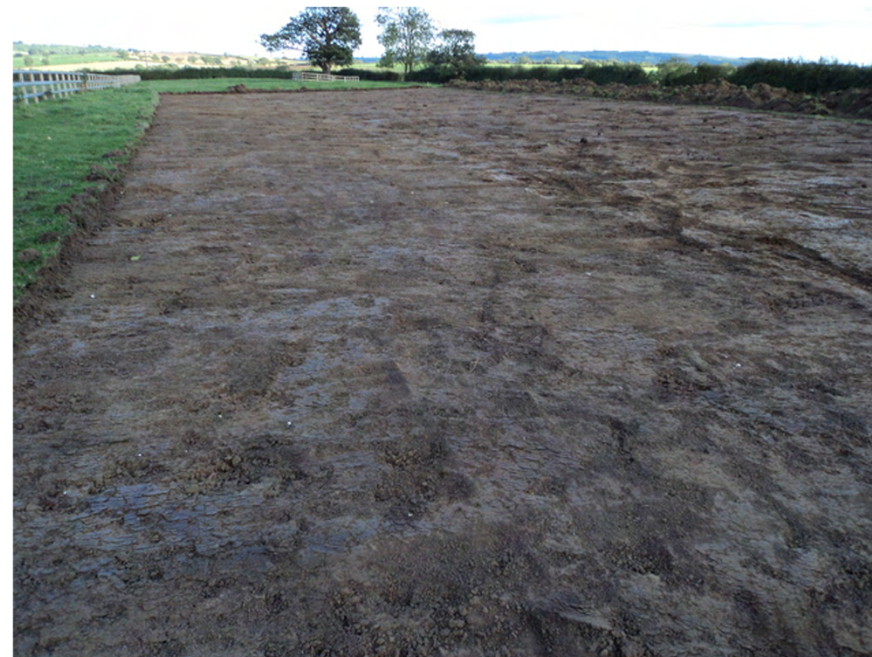
Plate 2. Ménage after Topsoil Strip. Facing East.
