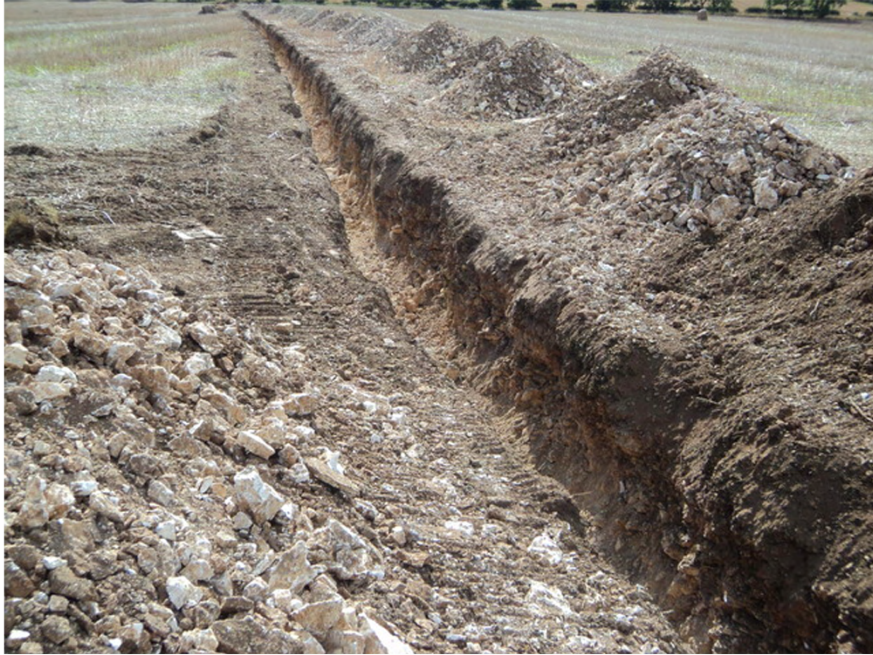
Plate 3. Cable Trench. Facing South-east.
