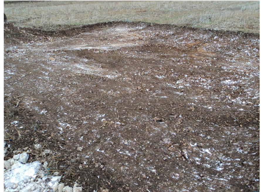
Plate 2. Wind Turbine Base after Topsoil Strip. Facing North-west.
