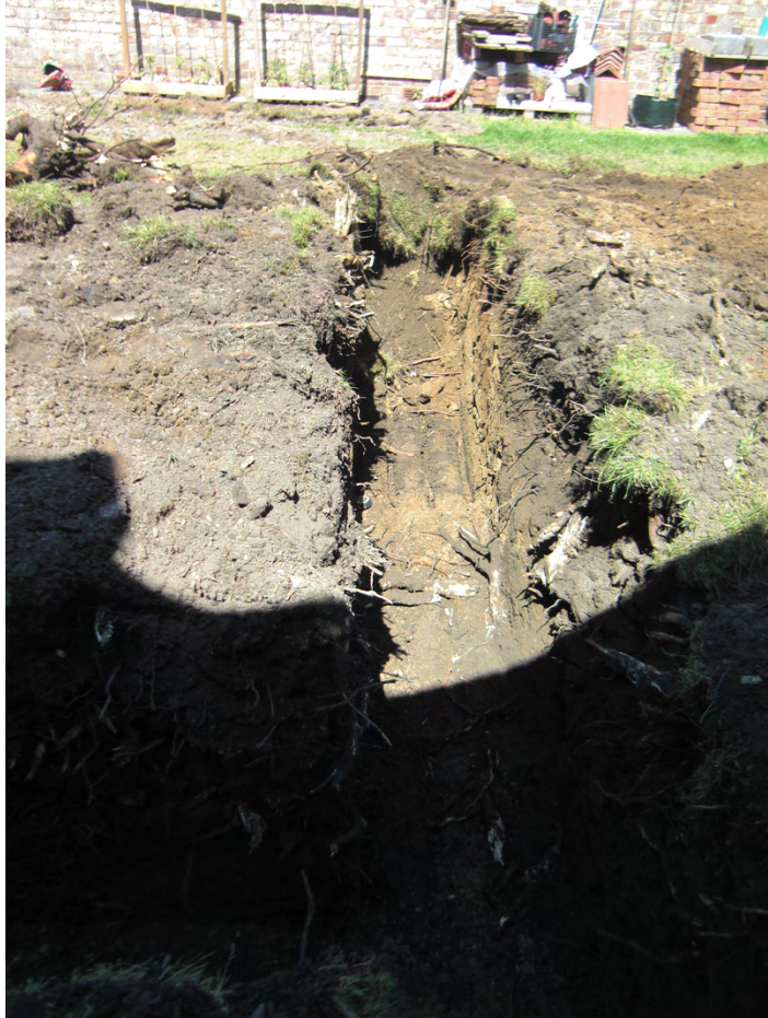
Plate 3. Strip Foundation. Facing South.
