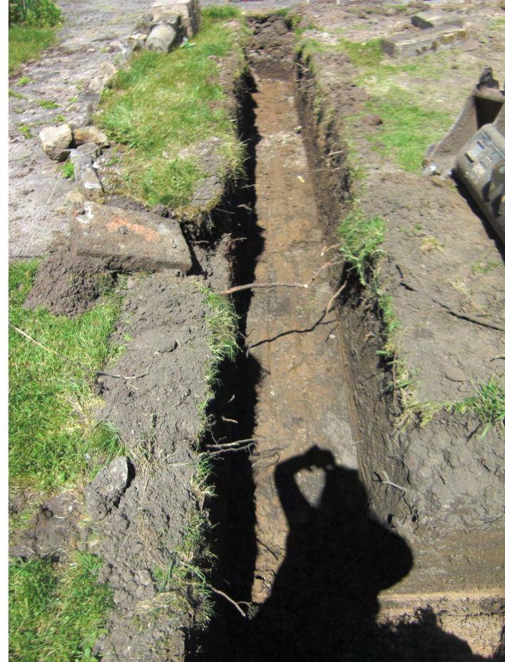
Plate 2. Foundation Trench. Facing East.
