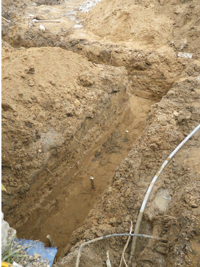
Plate 3. Strip Foundation Trench. Facing North-east.
