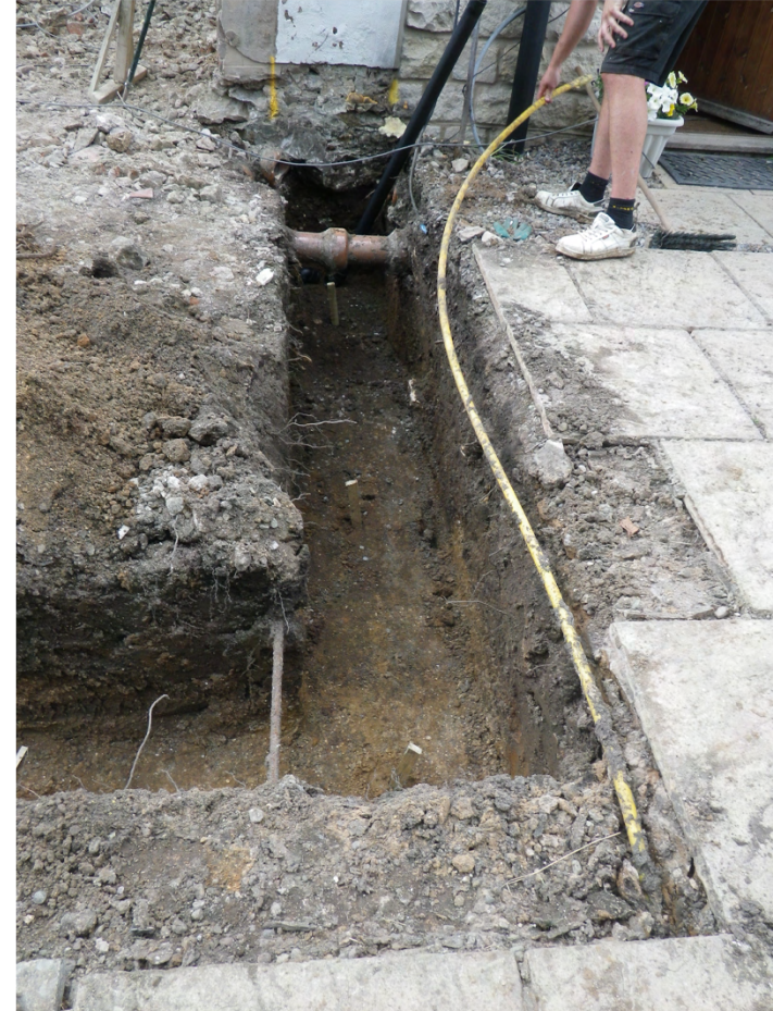
Plate 6. Strip Foundation Trench. Facing West.
