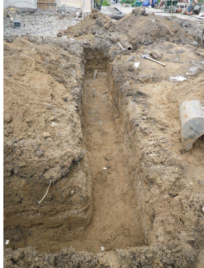
Plate 4. Strip Foundation Trench. Facing North.
