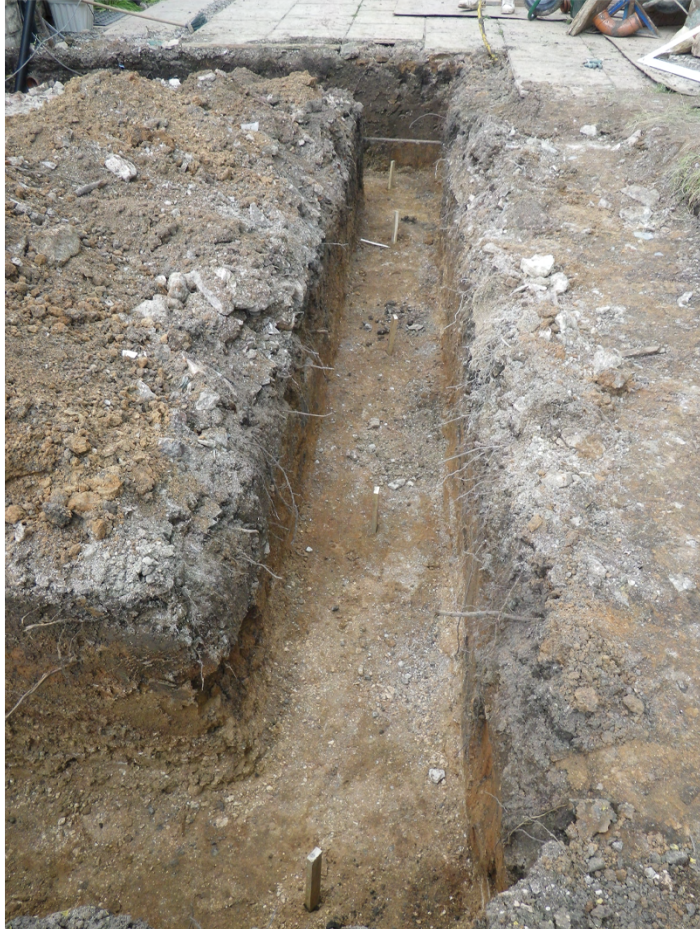
Plate 5. Strip Foundation Trench. Facing North.
