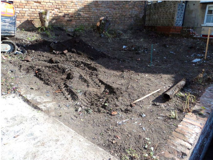
Plate 1. General View of Site. Facing North-east.
