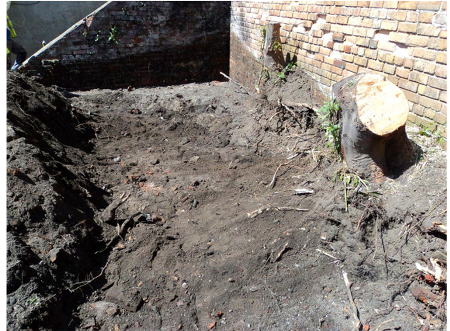
Plate 2. View of Stripped Area for Building Plot. Facing West.
