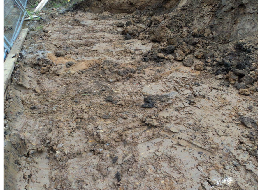
Plate 2. View of Stripped Area for Building Footprint. Facing East.
