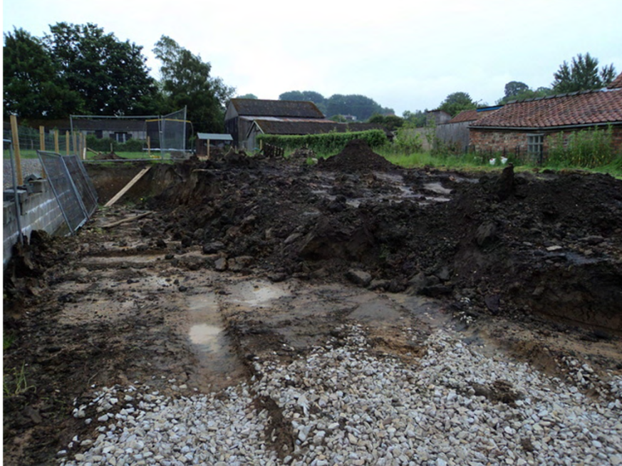
Plate 1. General View of Site. Facing East.
