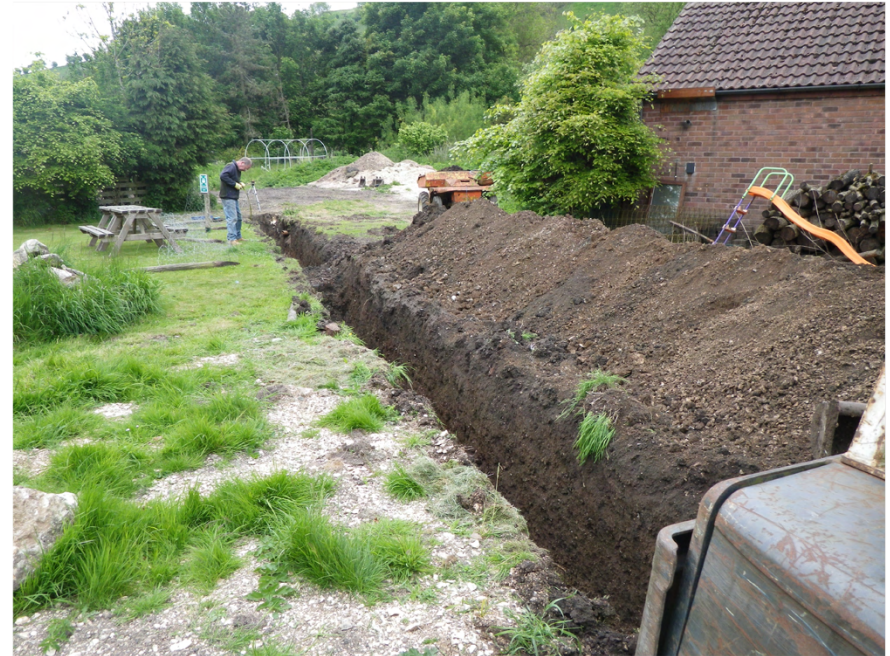
Plate 2. Drainage Trench. Facing South-west.
