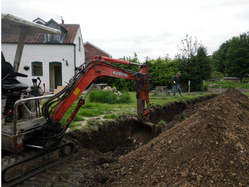
Plate 1. Drainage Trench. Facing North-east.
