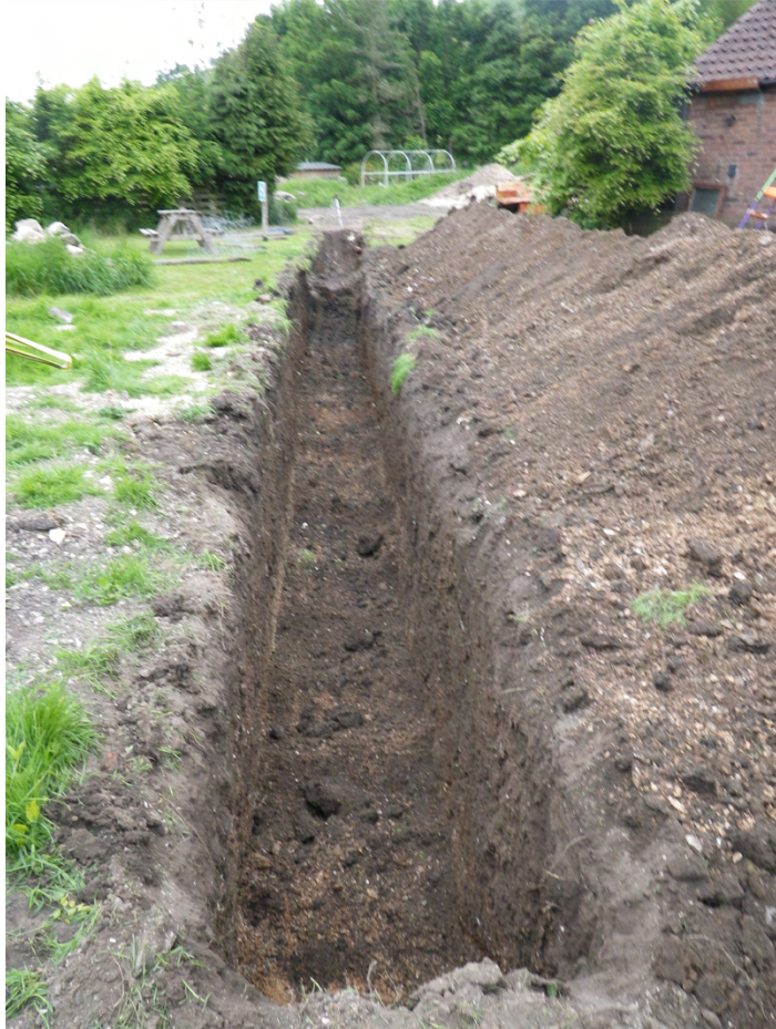
Plate 3. Drainage Trench. Facing South-west.
