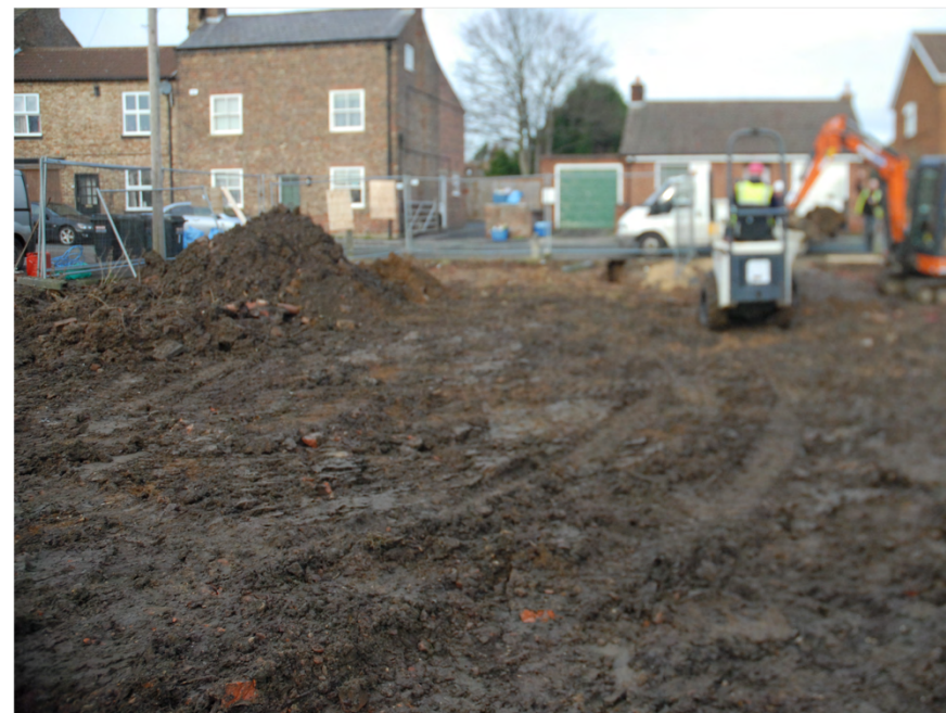
Plate 2. General View. Facing North.
