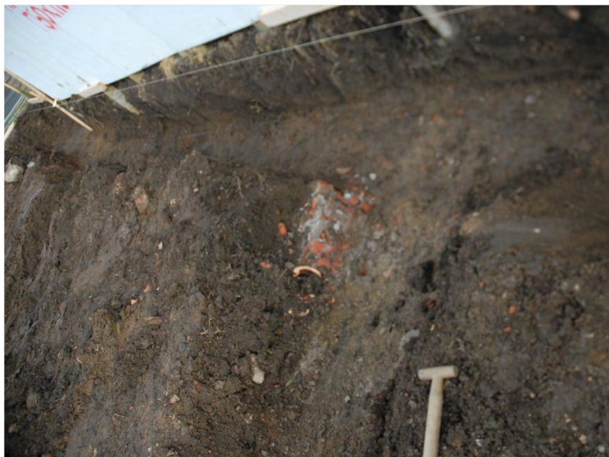
Plate 3. Foundation Trench. Facing South.
