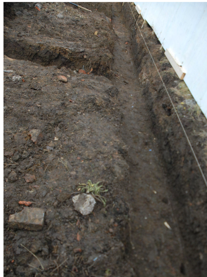
Plate 4. Foundation Trench. Facing South.
