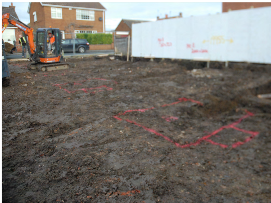
Plate 1. Genberal View of Foundation Trenches. Facing South-west.
