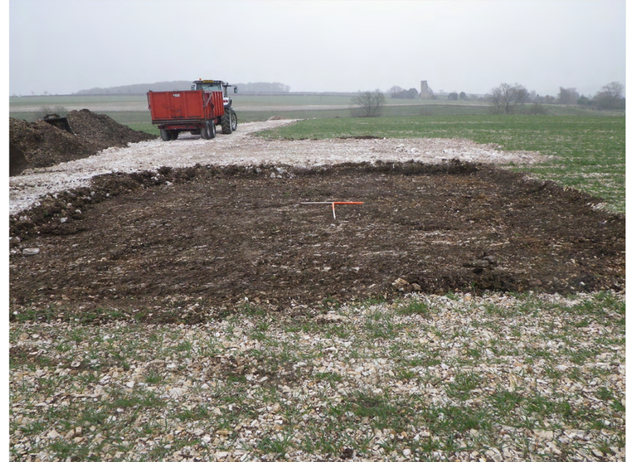
Plate 2. Turbine Base after Topsoil Strip. Facing East.
