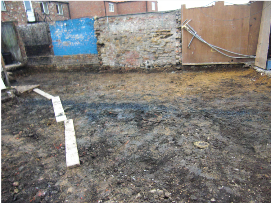
Plate 3. Area of Ground Reduction, Facing East.
