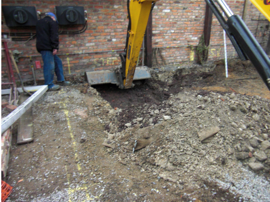
Plate 5. Foundation Trench. Facing North.
