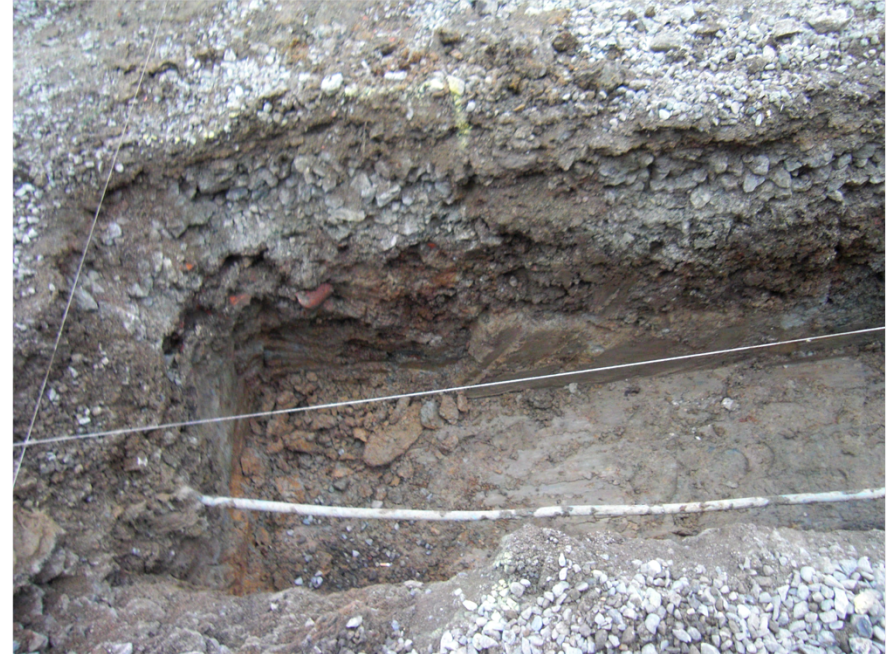
Plate 6. Foundation Trench. Facing East.
