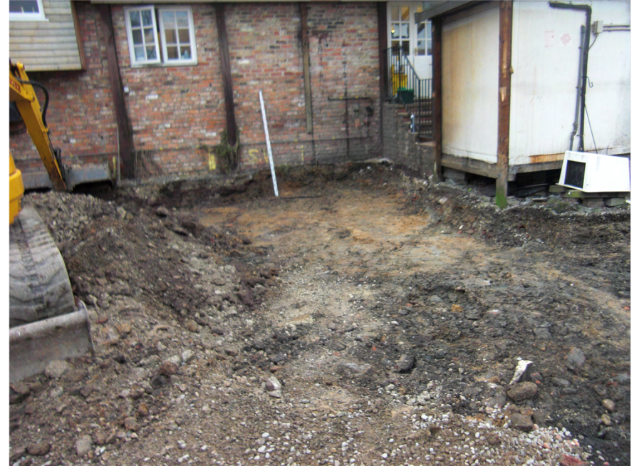
Plate 2. Site during ground reduction. Facing North.
