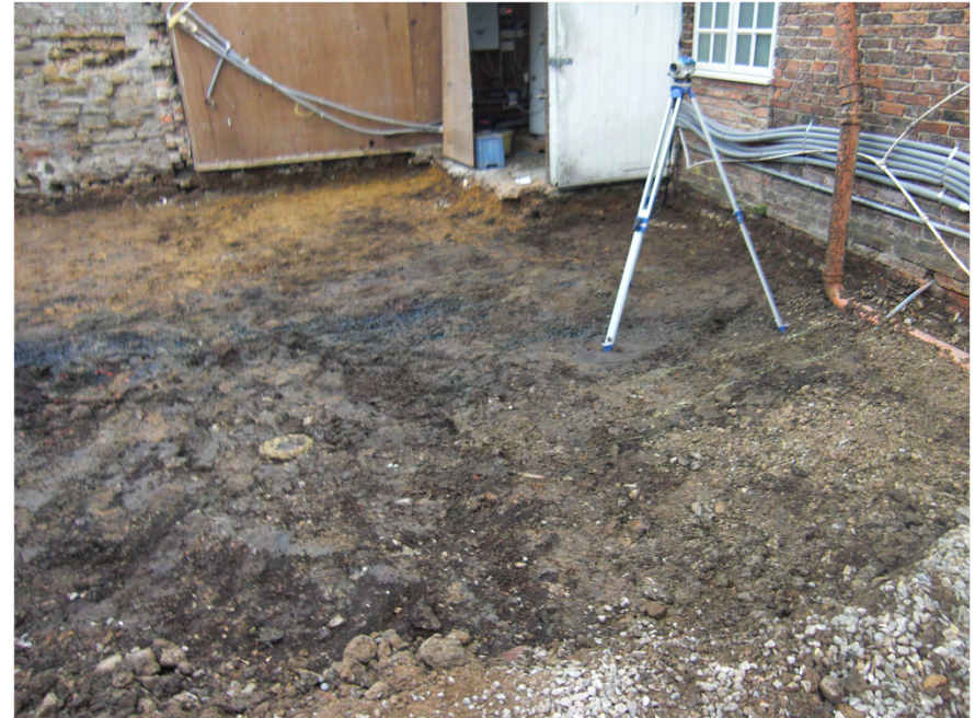
Plate 4. Area of Ground Reduction, Facing East.
