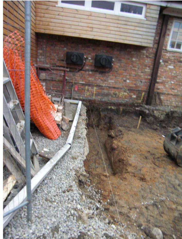
Plate 8. Foundation Trench. Facing North
