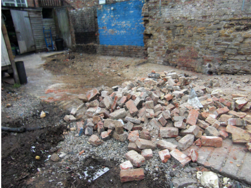
Plate 1 . Site after clearance. Facing North-east.
