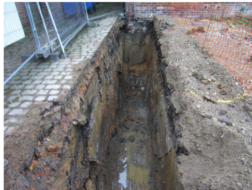
Plate 2. Foundation Trench. Facing North.
