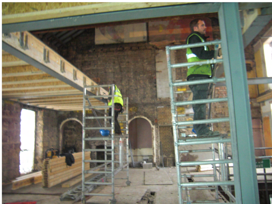
Plate 3. Interior of The West Parl Hotel. Facing North.
