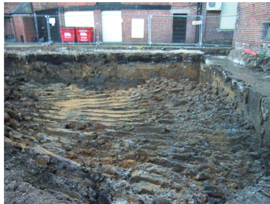
Plate 4. Excavation of Cellar. Facing North.
