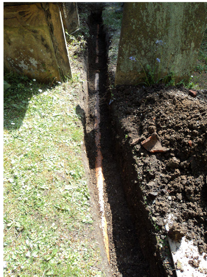
Plate 4. Gas Pipe Excavation Trench (Following Route of Modern Drainage). Facing West
