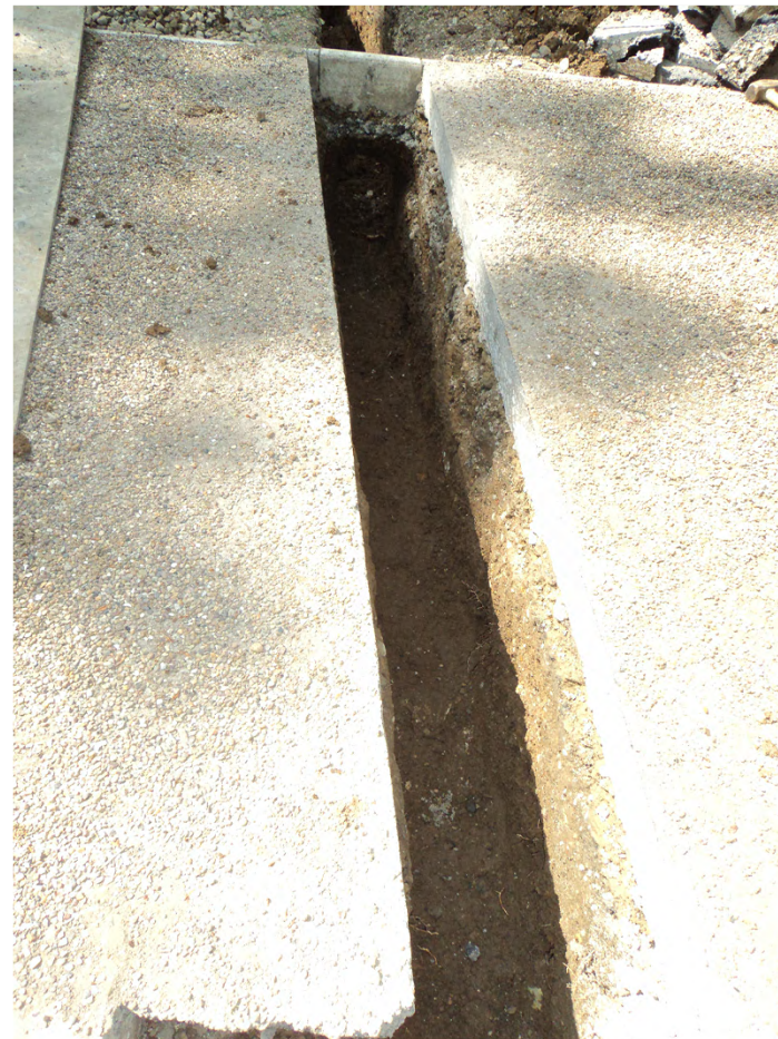
Plate 2. Gas Pipe Excavation Trench. Facing North-west.
