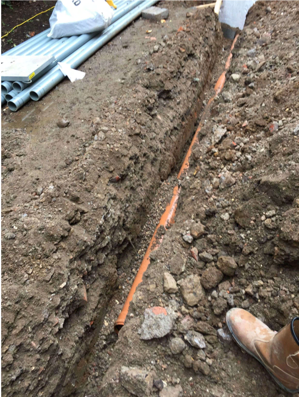
Plate 2. Drainage Trench. Facing North-west.
