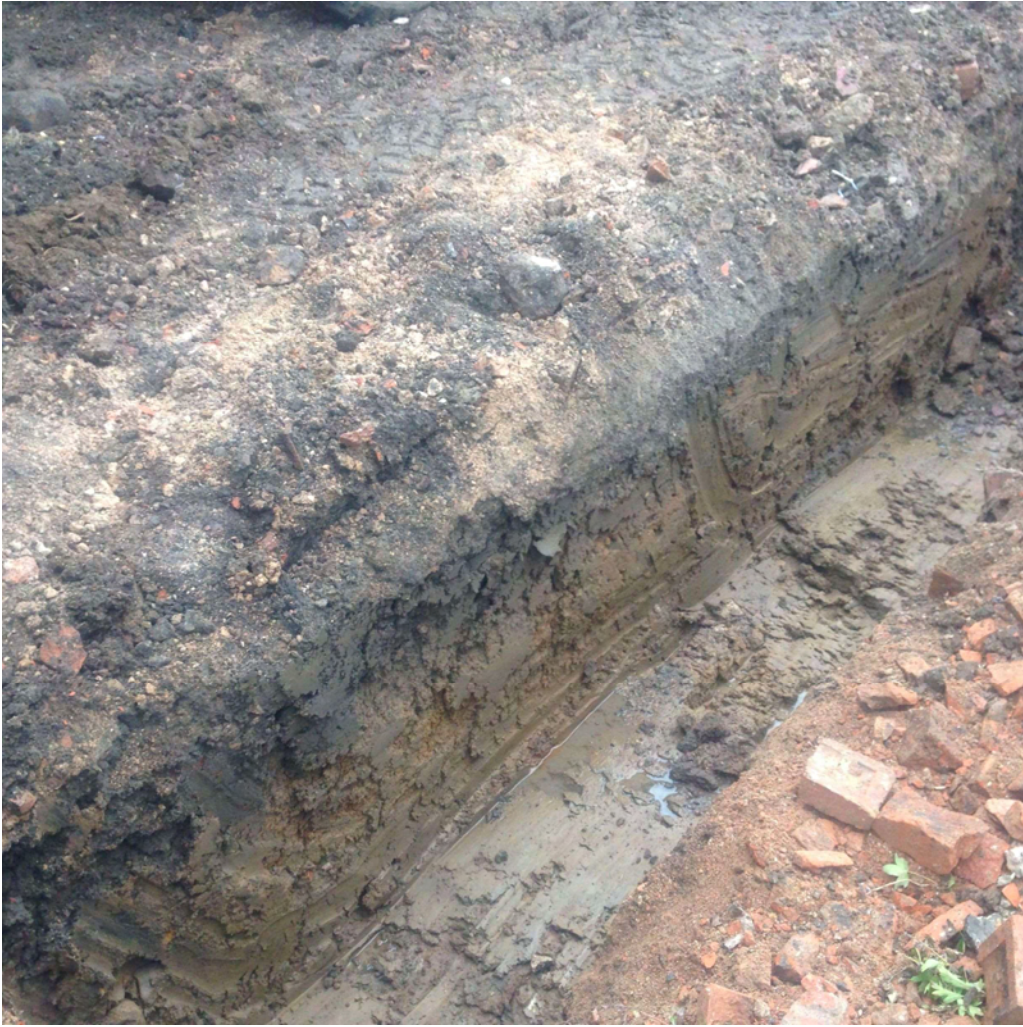
Plate 1. Foundation Trench. Facing North-west.
