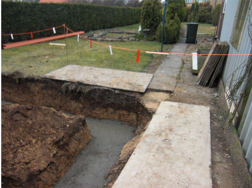
Plate 3. Foundation Trench. Facing North.
