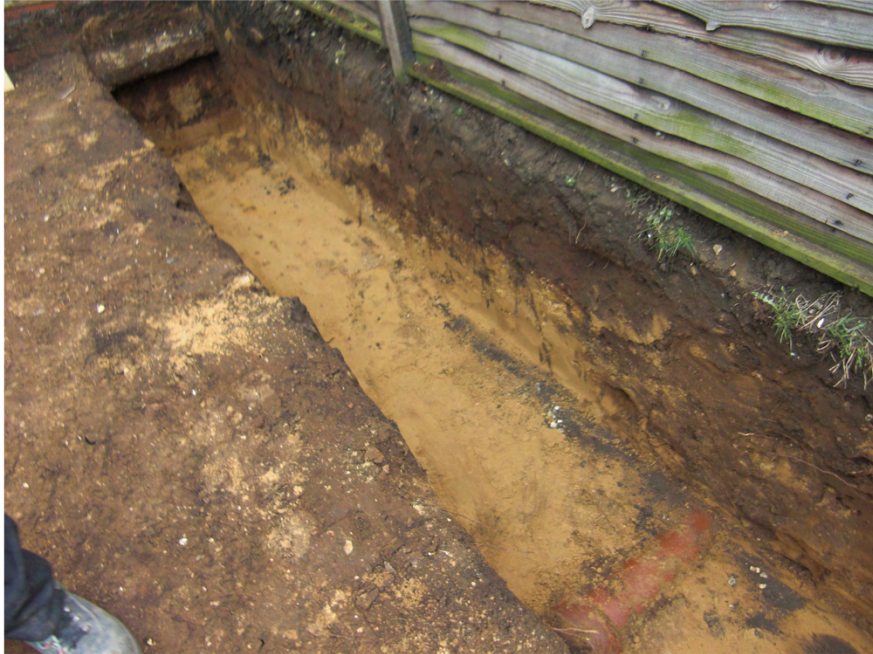
Plate 1. Founsdation Trench with Drain. Facing South-west.
