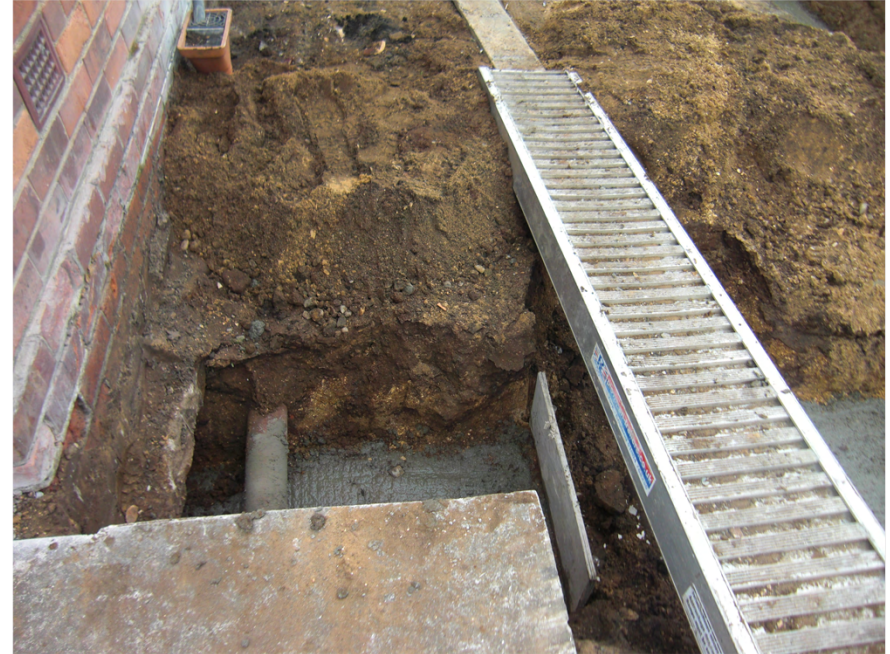
Plate 4. Services in Foundation Trench. Facing West.
