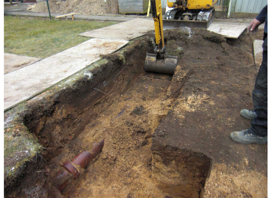
Plate 2. Foundation Trench with Drain. Facing North-east.
