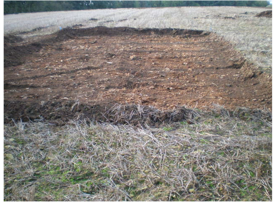
Plate 4. Garage Boundary after Topsoil Strip. Facing South-west.
