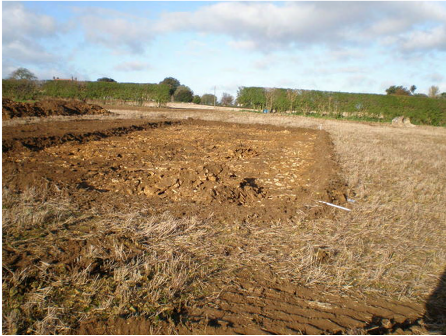
Plate 2. Plot Boundary after Topsoil Strip. Facing North-west.
