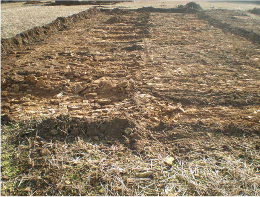
Plate 3. Plot Boundary after Topsoil Strip. Facing South-east.
