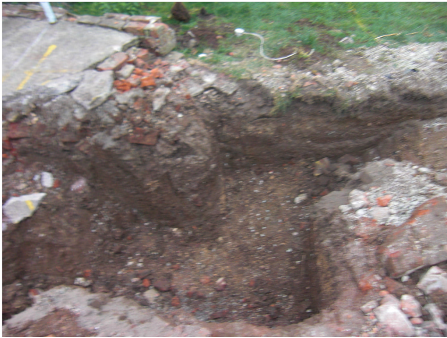
Plate 6. View of Footings.
