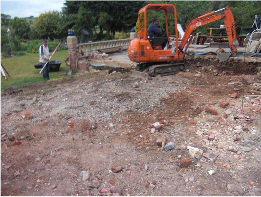
Plate 1. General View of Site. Facing South-west.
