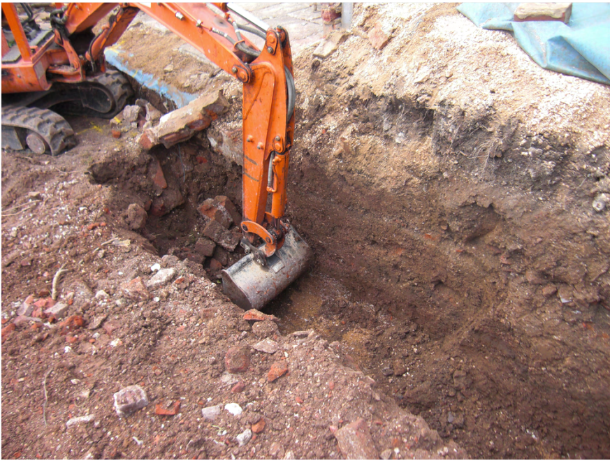
Plate 5. View of Footings.
