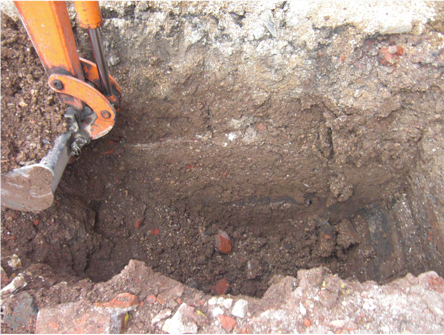
Plate 2. View of Footings.
