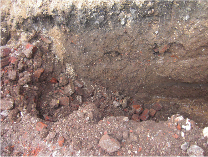
Plate 3. View of Footings.
