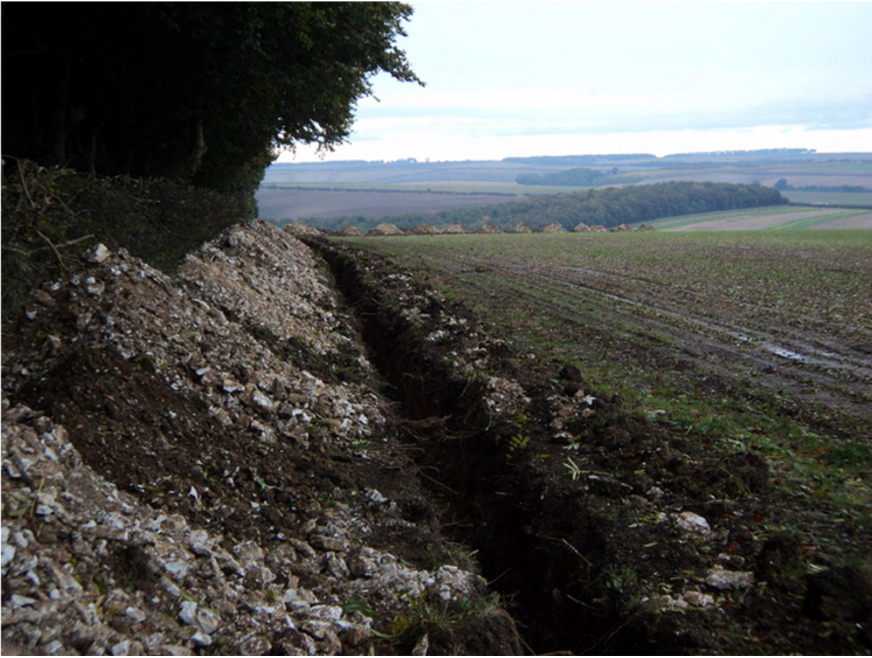
Plate 4. Cable Trench Route. Facing North.
