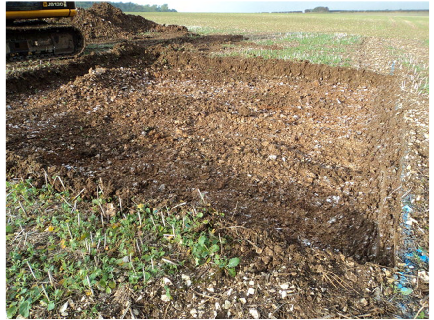
Plate 2. Wind Turbine Base after Topsoil Strip. Facing South-west.
