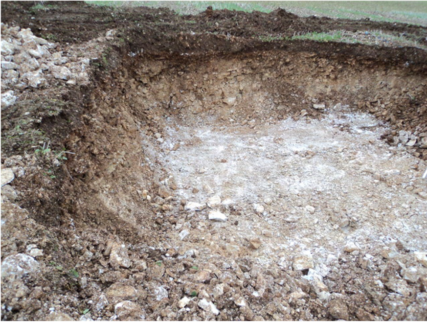
Plate 3. Wind Turbine Base excavated to Formation Level. Facing North-west.
