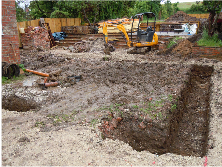
Plate 4. Site Post-excavation. Facing North-west.
