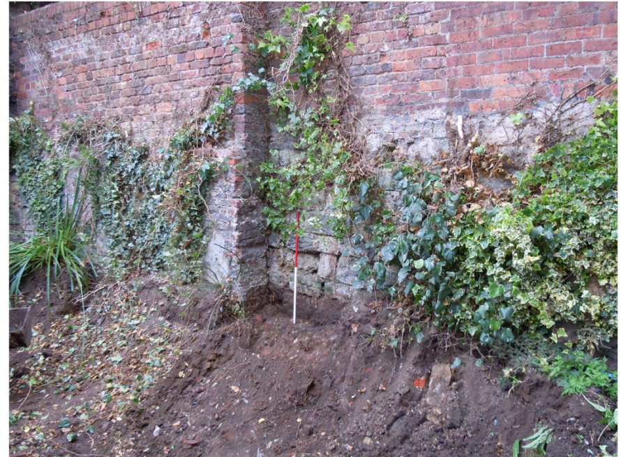
Plate 2. Northern Boundary Wall. Facing North West.
