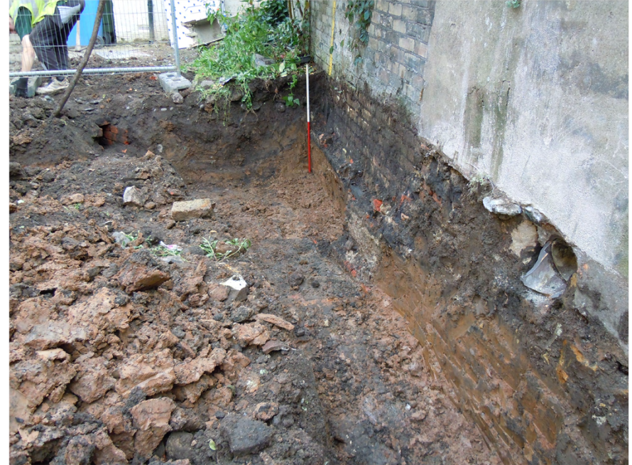
Plate 4. Western foundation Trench. Facing South West.
