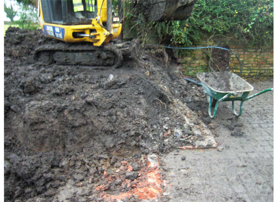
Plate 2. Area during ground reduction. Facing North.
