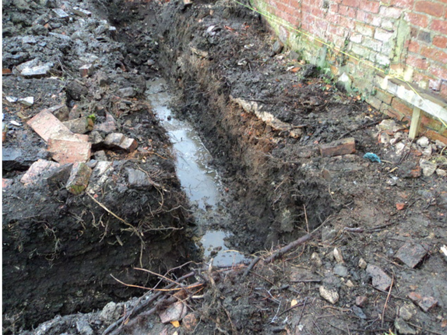
Plate 3. Section of Southern Foundation. Facing East.
