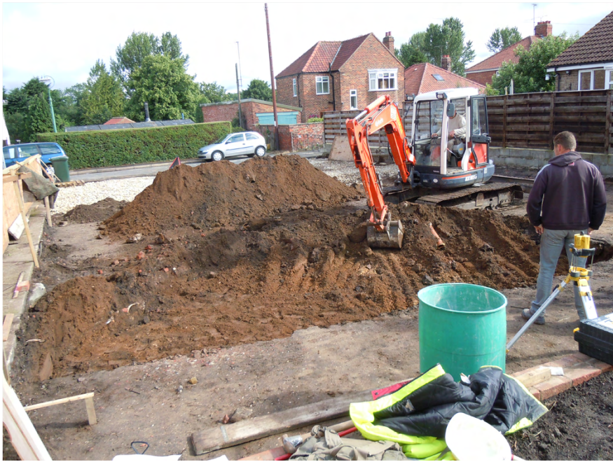
Plate 1. General View of Site Pre-excitation. Facing North-east.
