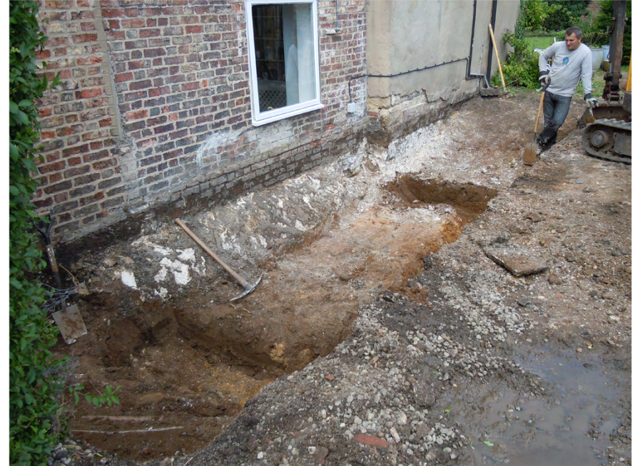
Plate 4. Completed site. Facing North-east.
