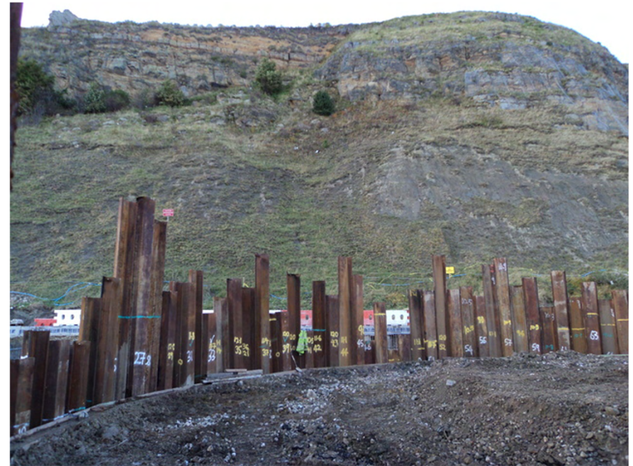
Plate 6. General View of Toll House Pumping Station. Facing North-west.
