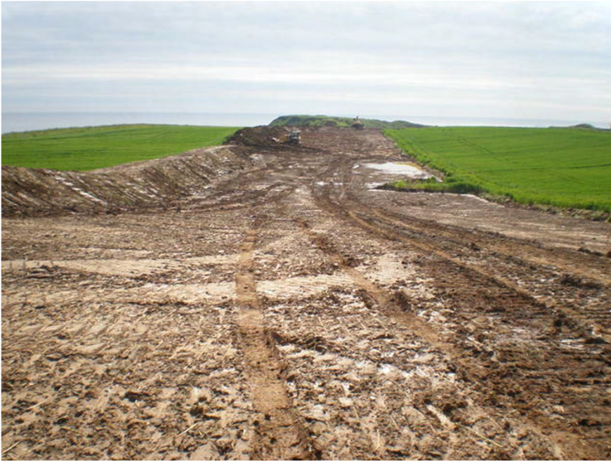
Plate 1. General View of Scarborough WwTW. Facing South.
