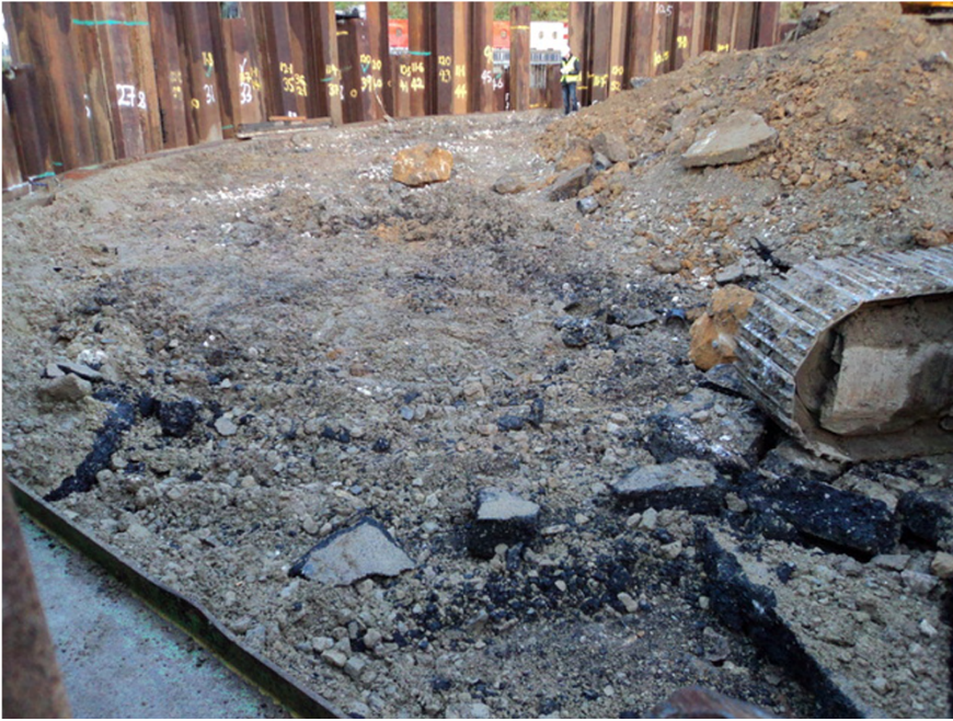
Plate 7. Underground Storage Tank during Stripping. Facing North-west.
