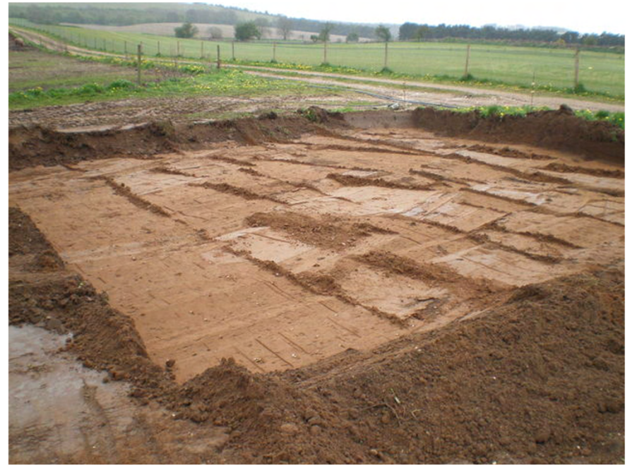
Plate 2. Wind Turbine Base after Topsoil removal. Facing South-west.
