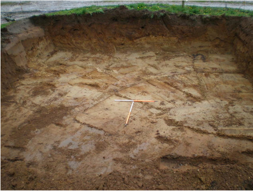
Plate 3. Wind Turbine Base at Formation Level. Facing West.
