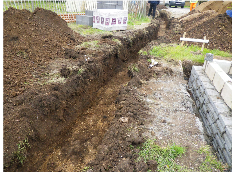
Plate 6. View of Service Trench. Facing South.
