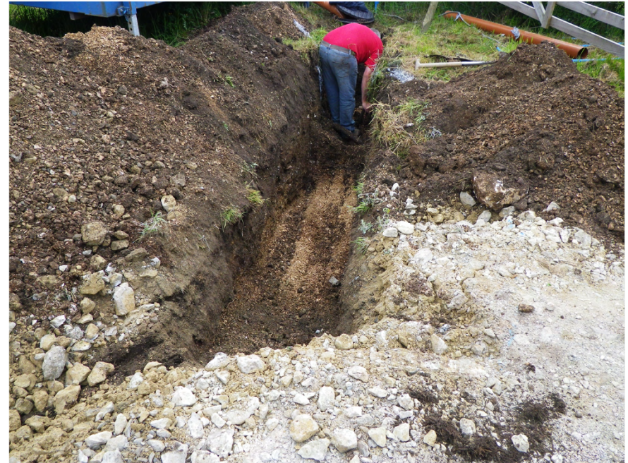
Plate 4. View of Garage Plot, Facing South-east.
