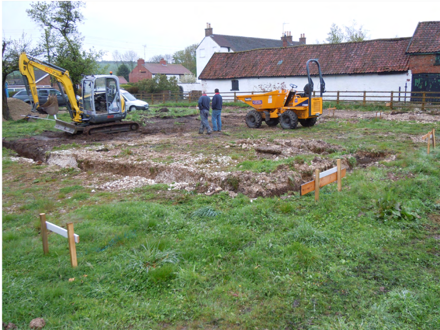
Plate 1. View of Site. Facing South-west.
