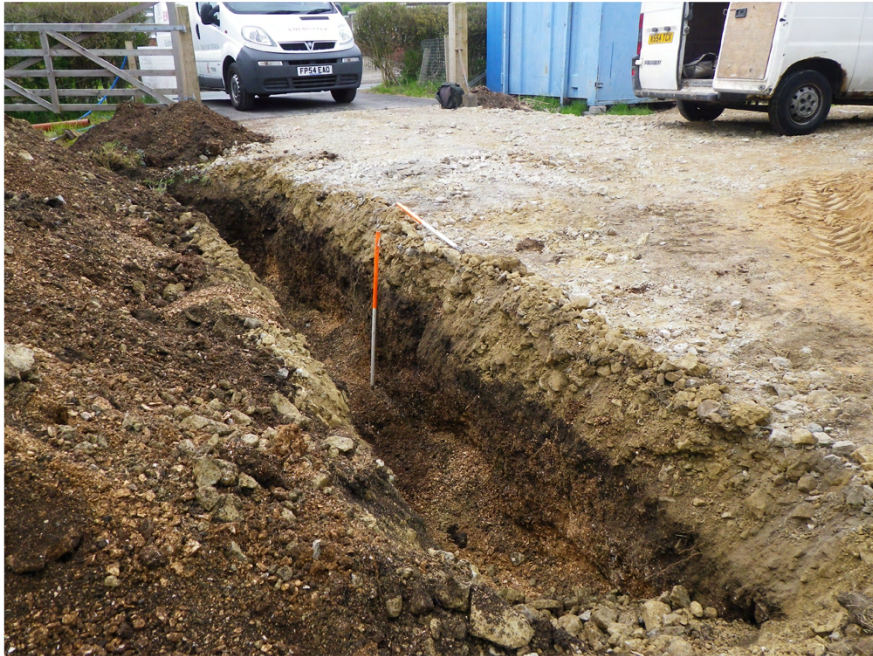
Plate 5. View of Tree Bowl in Service Trench. Facing South.
