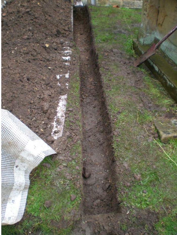
Plate 3. Drainage Gully Excavation. Facing East.
