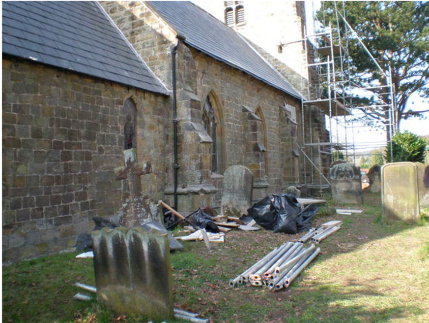
Plate 1. General View of Site. Facing South-west.
