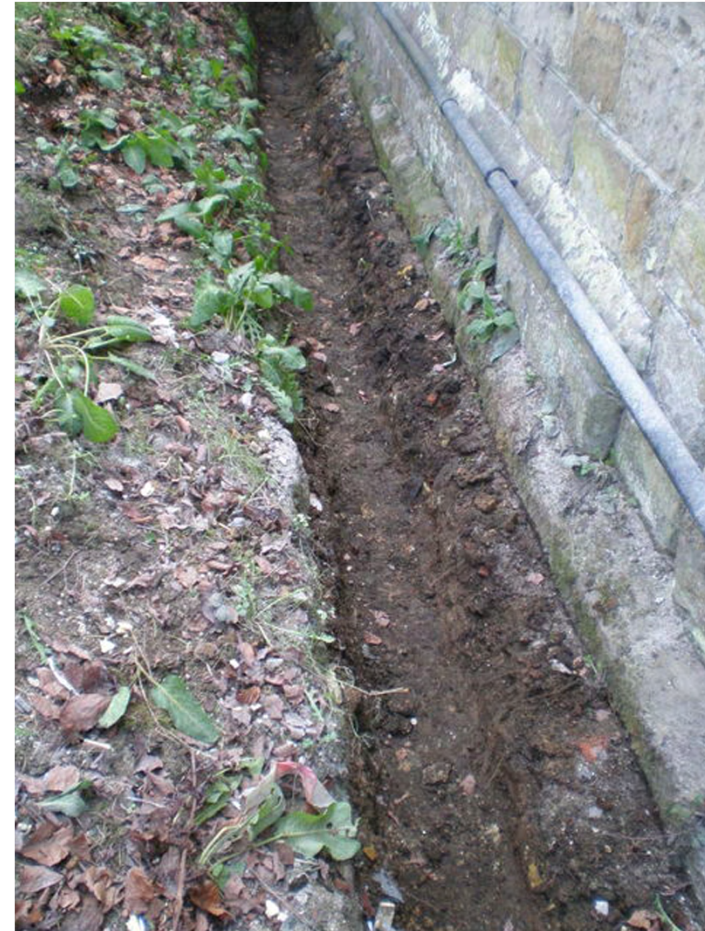
Plate 2. Drainage Gully Excavation. Facing East.
