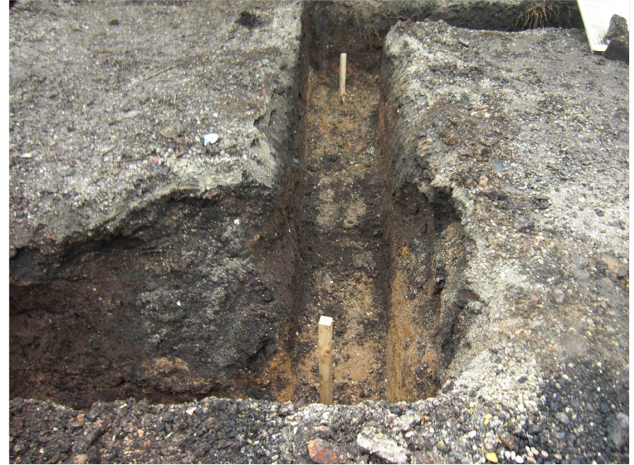
Plate 2. View of Foundation Trench. Facing South.
