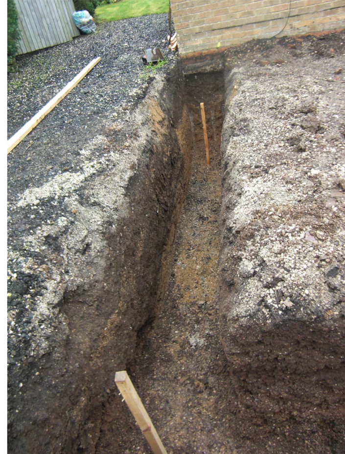
Plate 4. View of Foundation Trench. Facing South.
