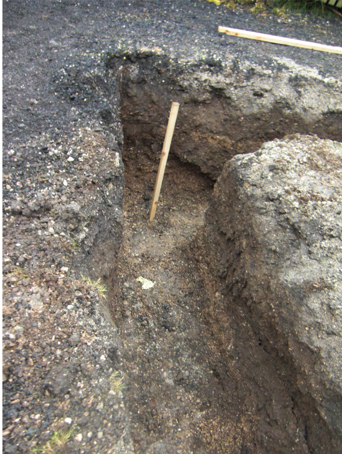
Plate 3. View of Foundation Trench. Facing West.
