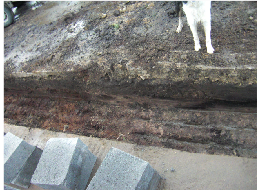
Plate 4. View of Foundation Trench. Facing North-West,
