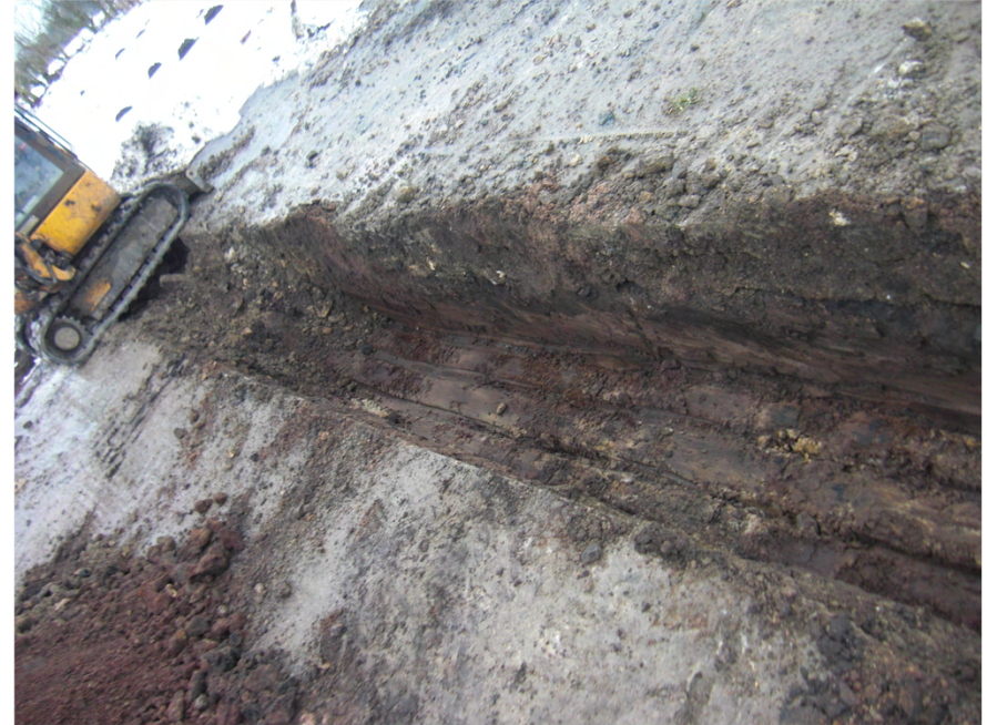
Plate 2. View of Foundation Trench. Facing South-west.
