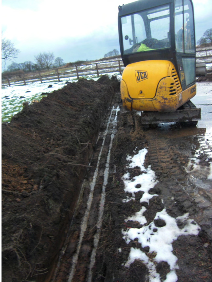
Plate 3. View of Foundation Trench. Facing South-east.
