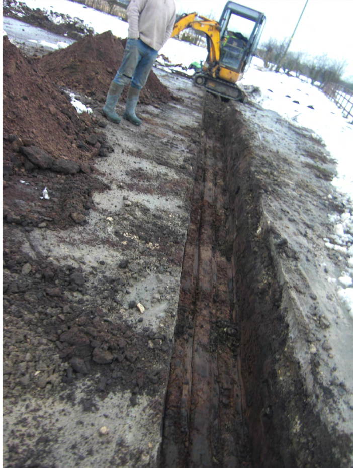
Plate 1. View of Foundation Trench. Facing South-west.
