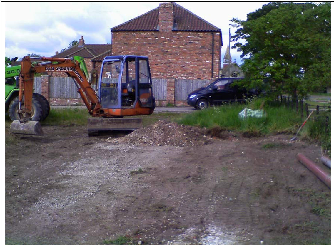
Plate 2. Proposed Development Area. Facing South-west.
