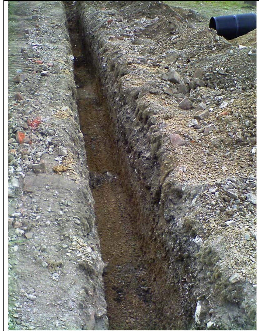
Plate 4. Drainage Trench. Facing North-west.
