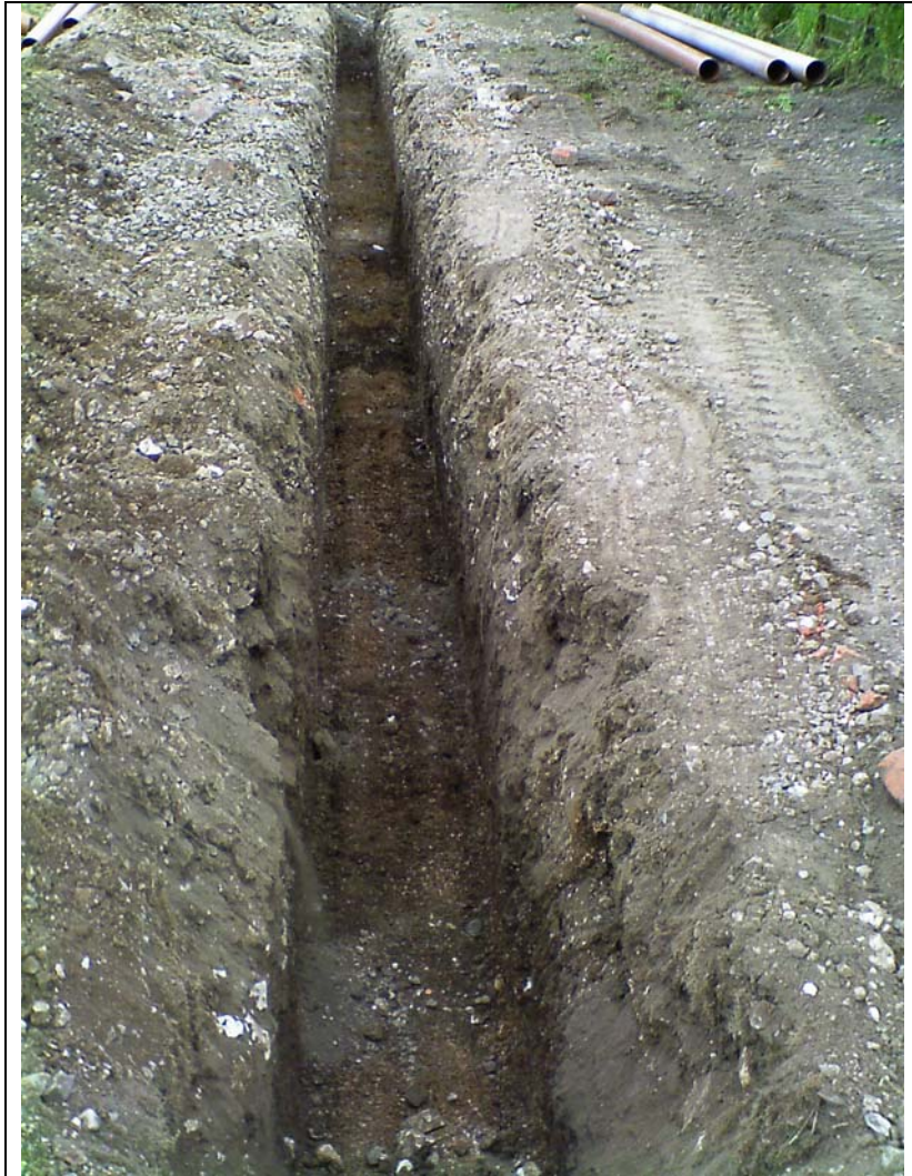
Plate 3. Drainage Trench. Facing South-west.
