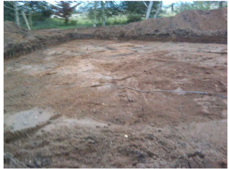
Plate 4. Area after Stripping. Facing North.
