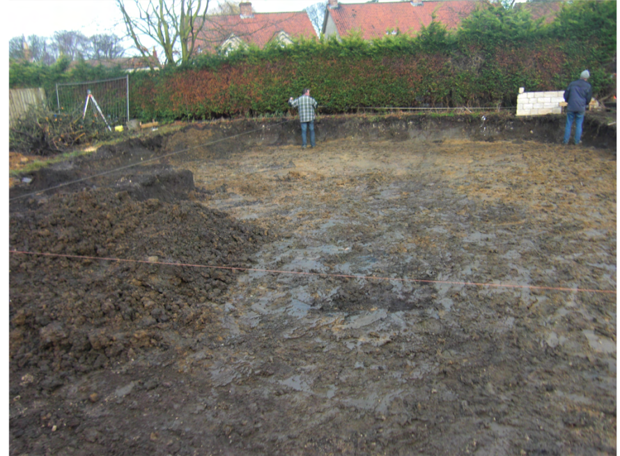
Plate 4. View of Site after Reduced Level Dig. Facing South-west.
