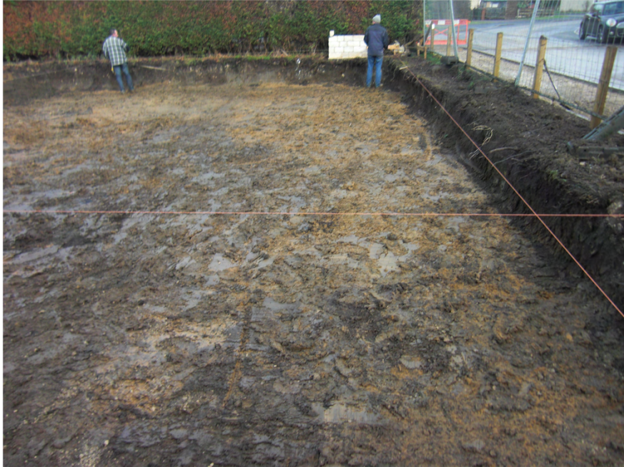
Plate 3. View of Site after Reduced Level Dig. Facing West.
