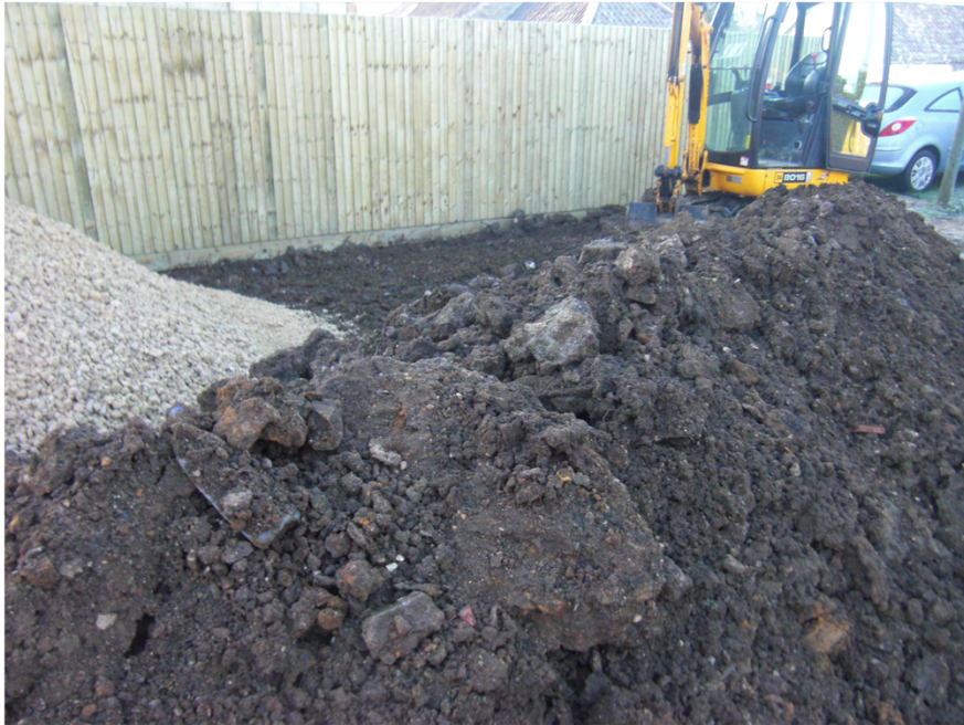
Plate 1. View of Site during Topsoil Stripping. Facing South.
