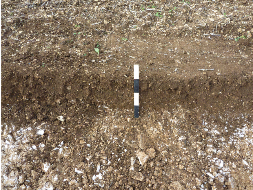
Plate 11. East facing section of stripped turbine base. Facing West.
