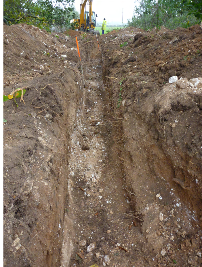
Plate. 14. Turbine 2 cable route through woodland belt after excavation. Facing East.
