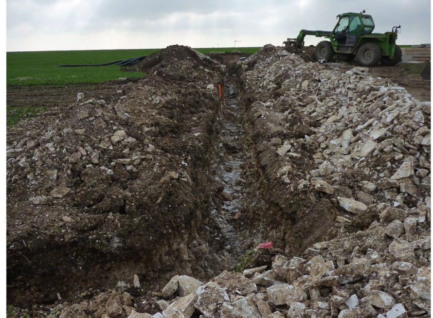
Plate 4. Turbine 1 cable run from turbine base after excavation. Facing South.
