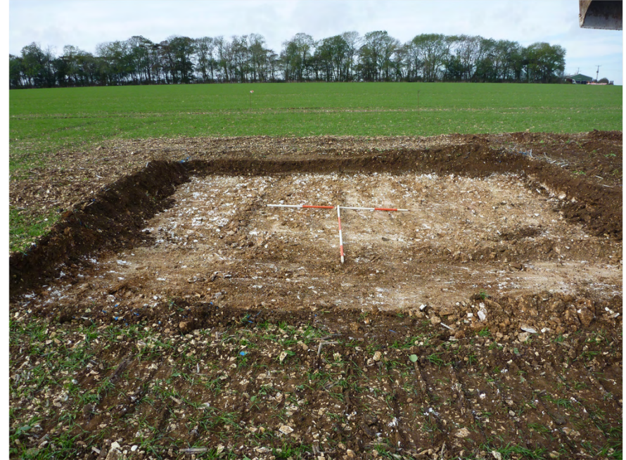
Plate 10. Site of Turbine 2 after topsoil strip. Facing West.
