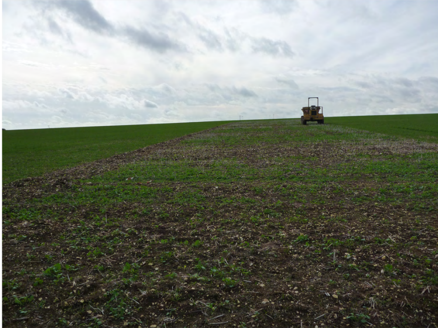
Plate 1. General location of Turbine 1 prior to excavation. Facing South.
