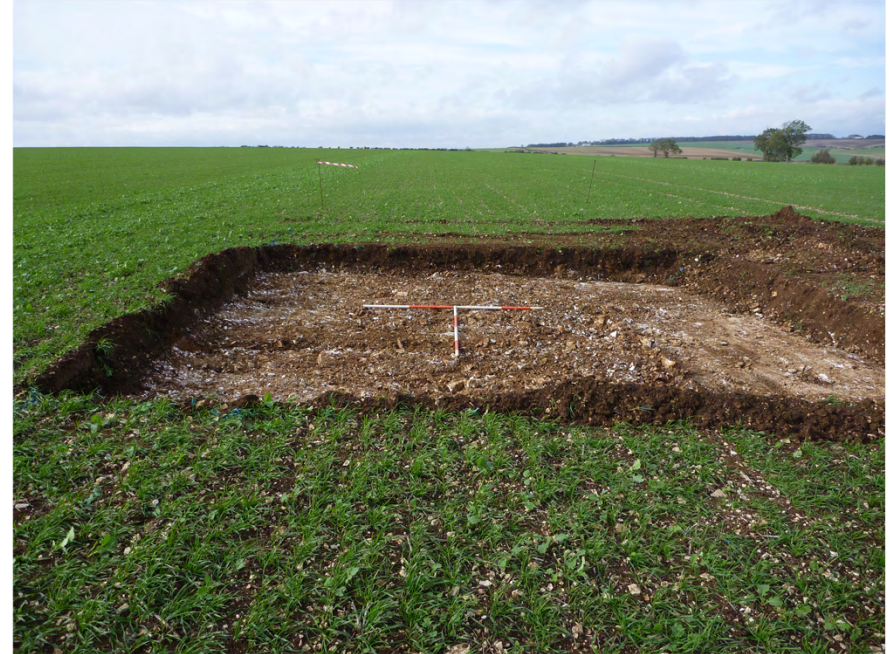
Plate 2. Site of Turbine 1 after topsoil strip. Facing South.
