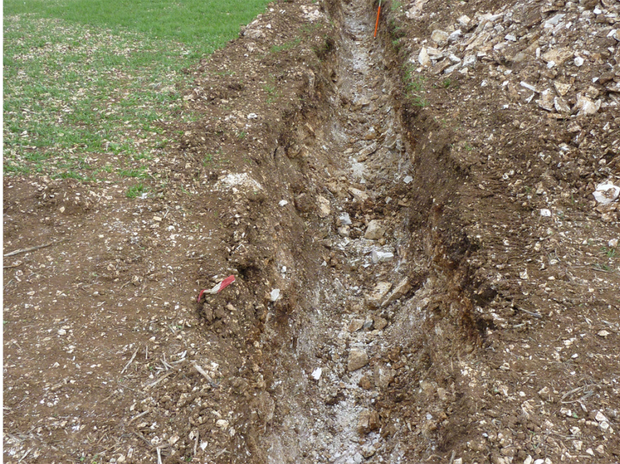
Plate 5. Turbine 1 cable run after excavation. Facing North-east.
