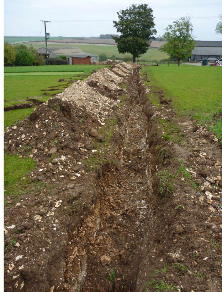
Plate 16. Turbine 2 cable route to transformer after excavation. Facing North.
