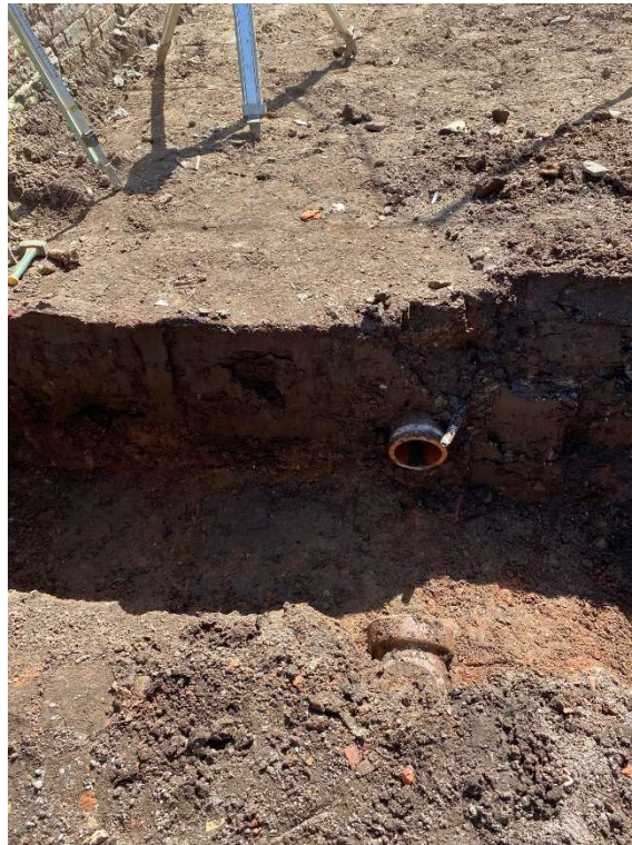
Plate 7: Modern drain in the foundation trench. Facing north.
