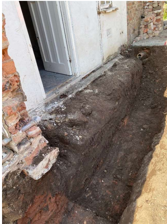
Plate 5: Foundation trench (0.50m deep). Facing south-west.
