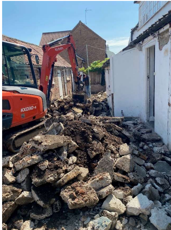
Plate 1: Removal of existing concrete slab. Facing east.
