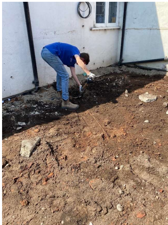
Plate 2: Area of extension after removal of the concrete. Facing south-west.
