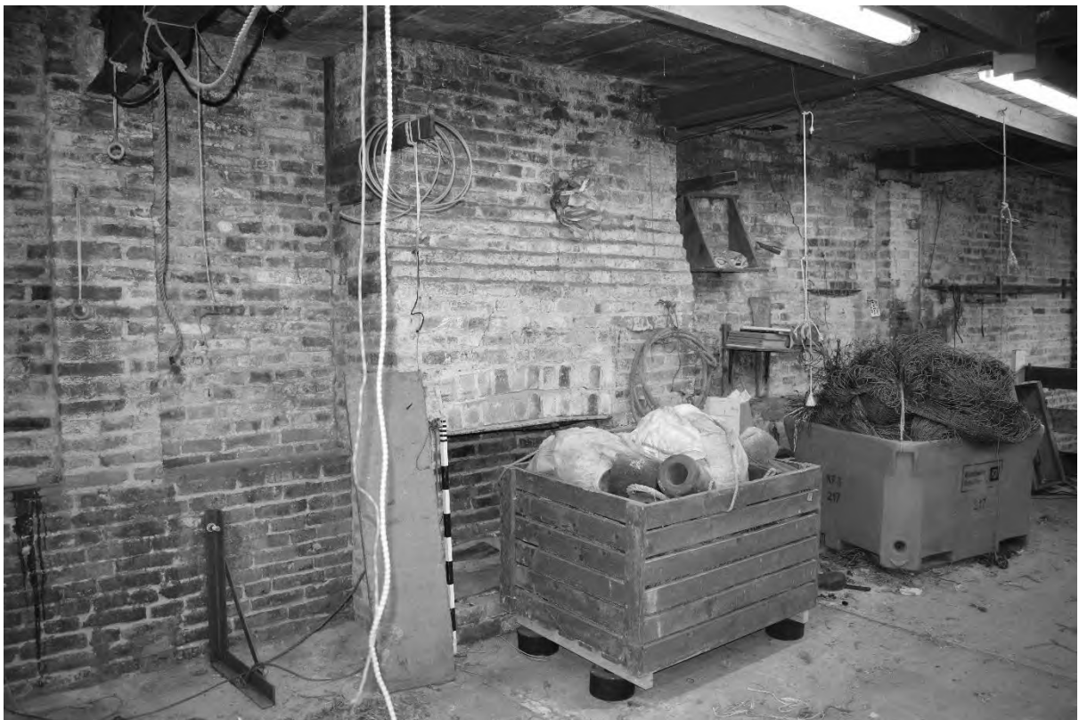
Plate 34. Interior First Floor Workshop: Disused Forge (DSC_0633). Facing South-east.
