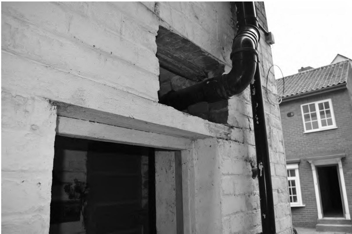
Plate 28. Outside Toilet on Ground Floor (DSC_0701). Facing South-east.
