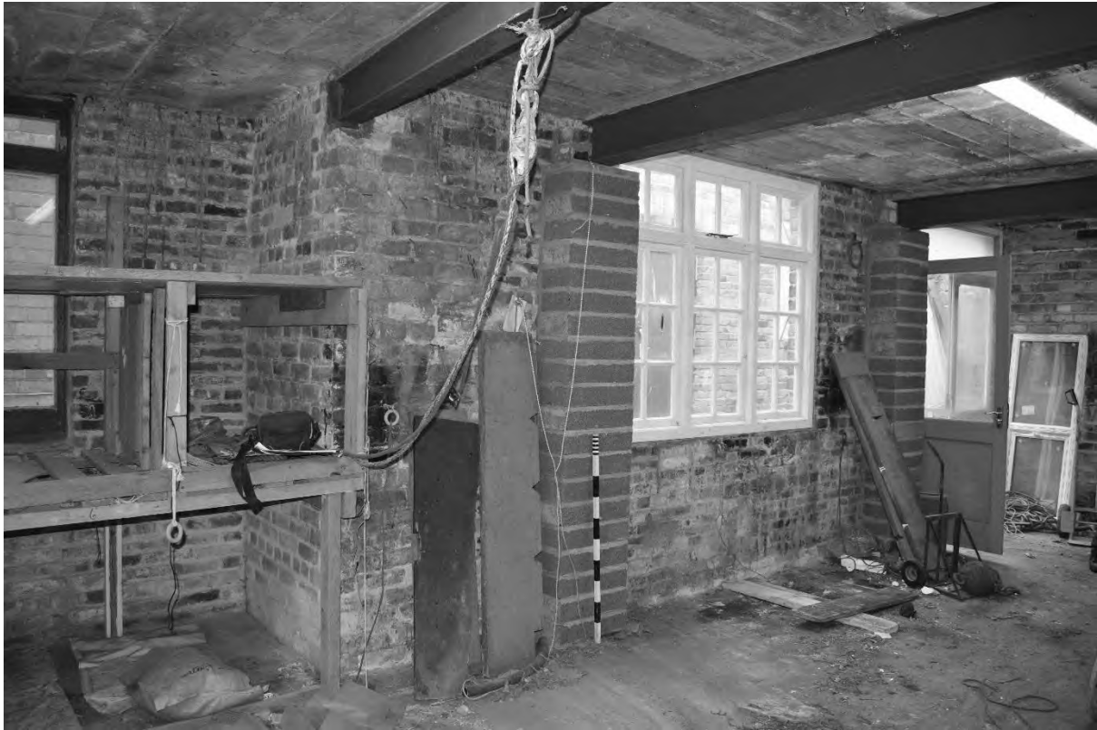
Plate 41. Interior First Floor Workshop (DSC_0645). Facing South-west.
