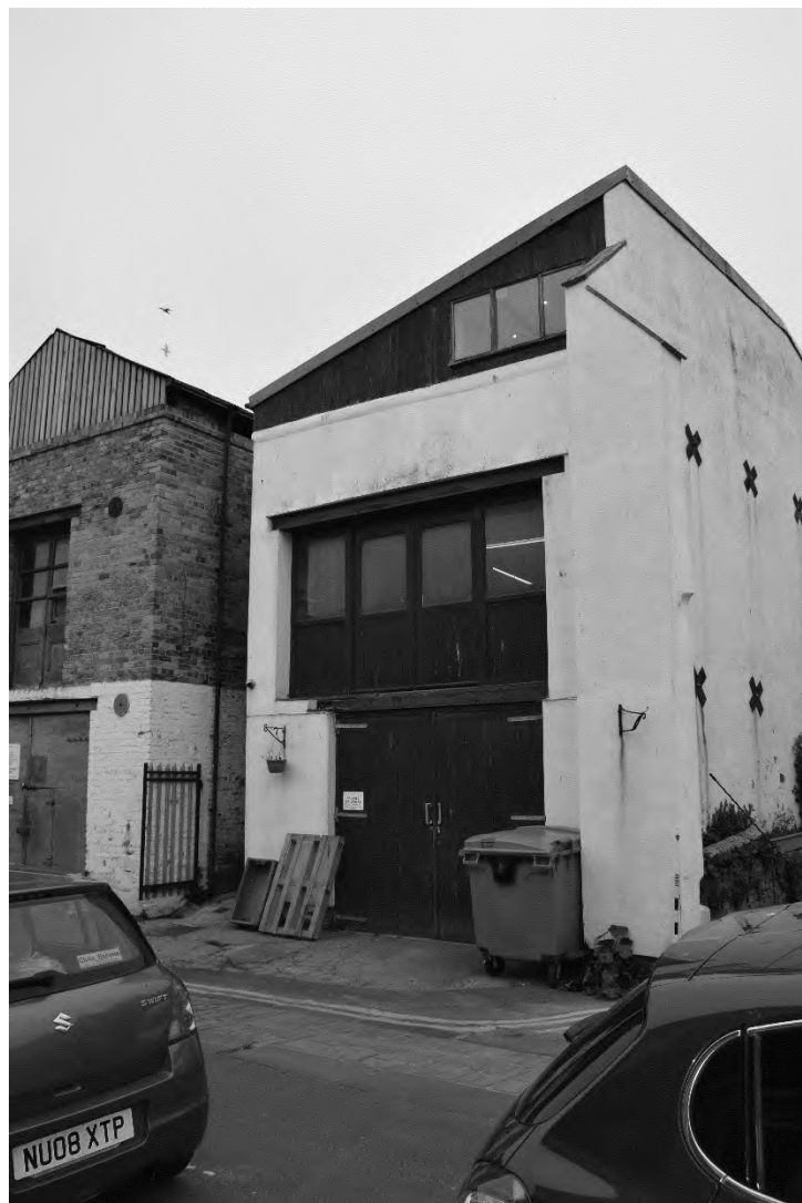
Plate 4: Exterior South & East Elevations (DSC_674). Facing North-west.
