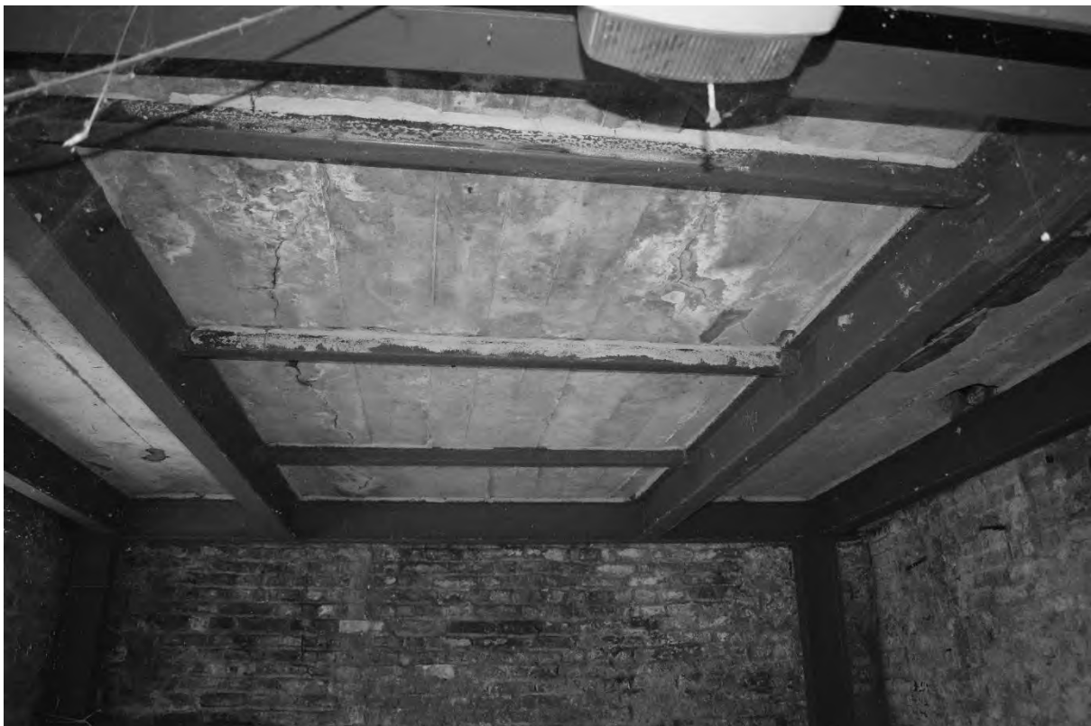
Plate 48. Interior First Floor Store Ceiling (DSC_0653). Facing North.
