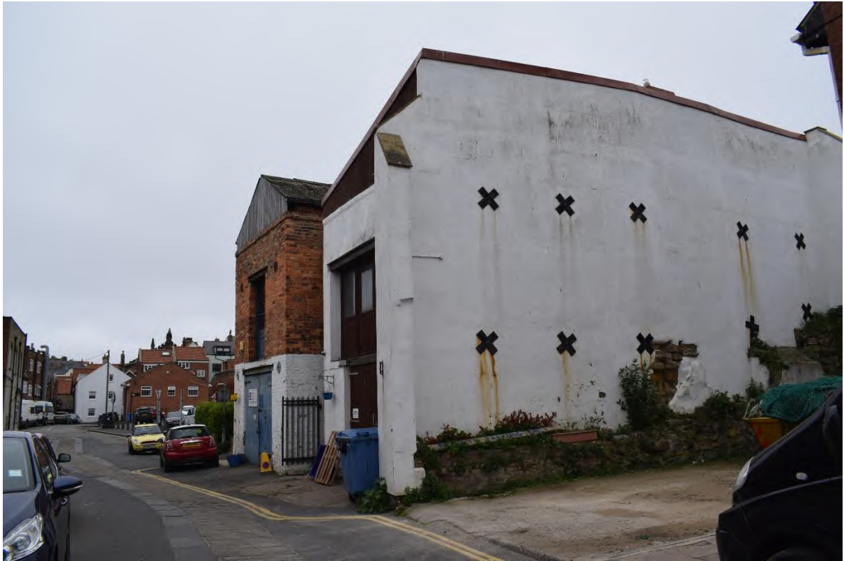
Plate 1. 22a Quay Street (DSC_0695). Facing West.
