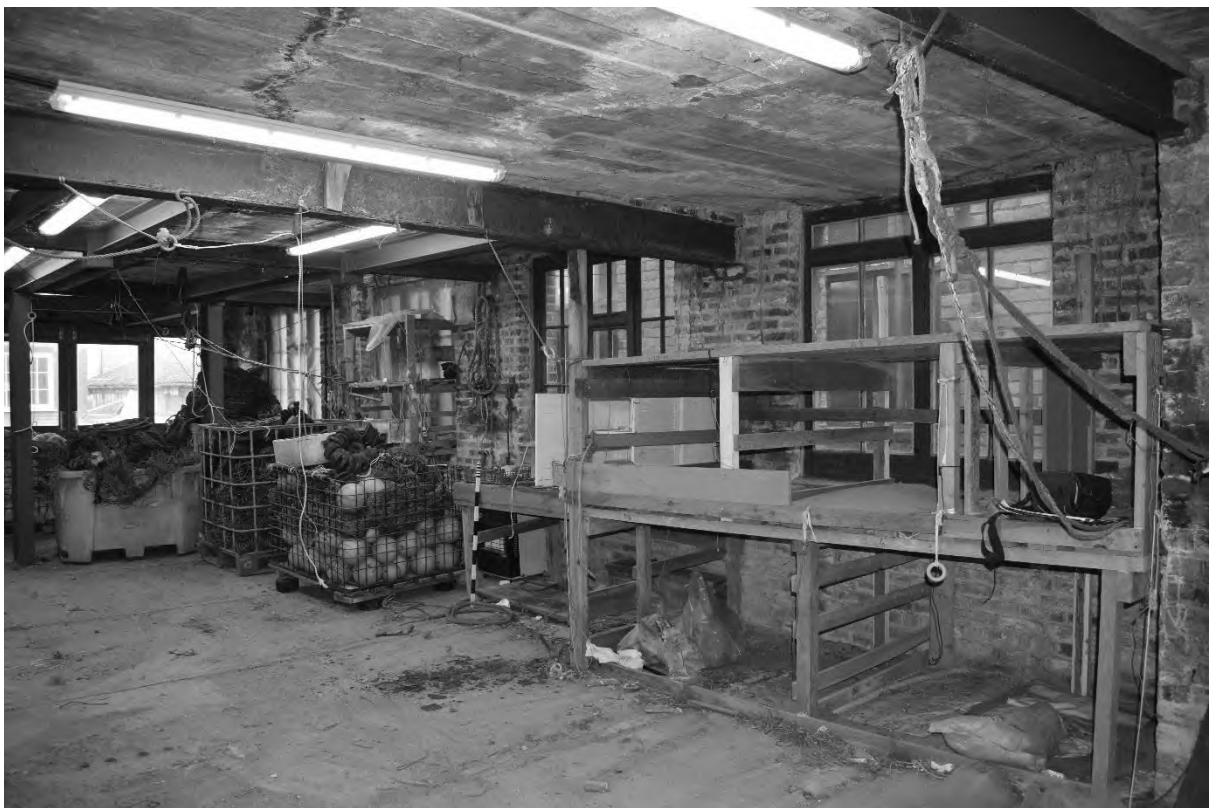
Plate 38. Interior First Floor Workshop (DSC_0641). Facing South-west.
