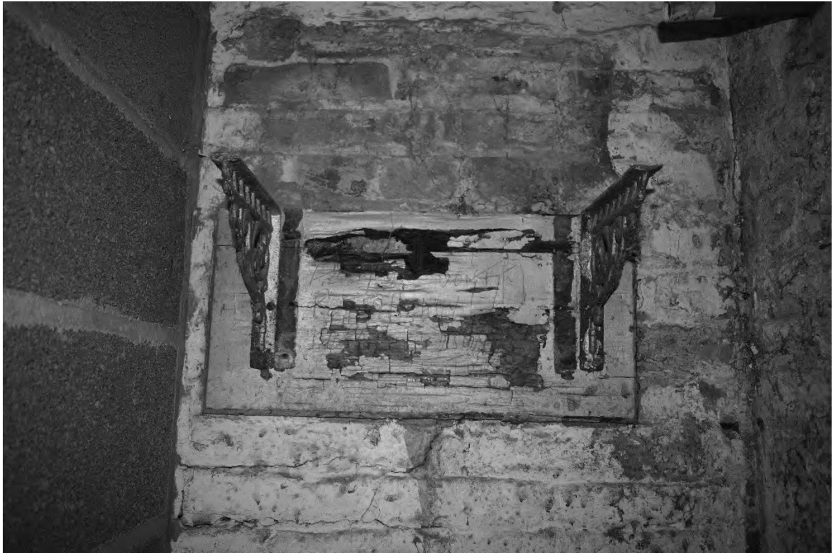
Plate 29. Disused Cistern Brackets (DSC_0702). Facing South.
