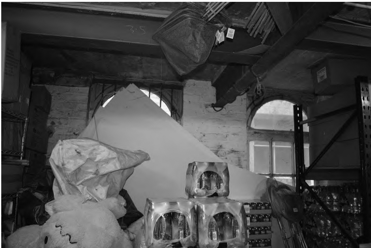
Plate 26, Interior Ground Floor (DSC_0632). Facing West.
