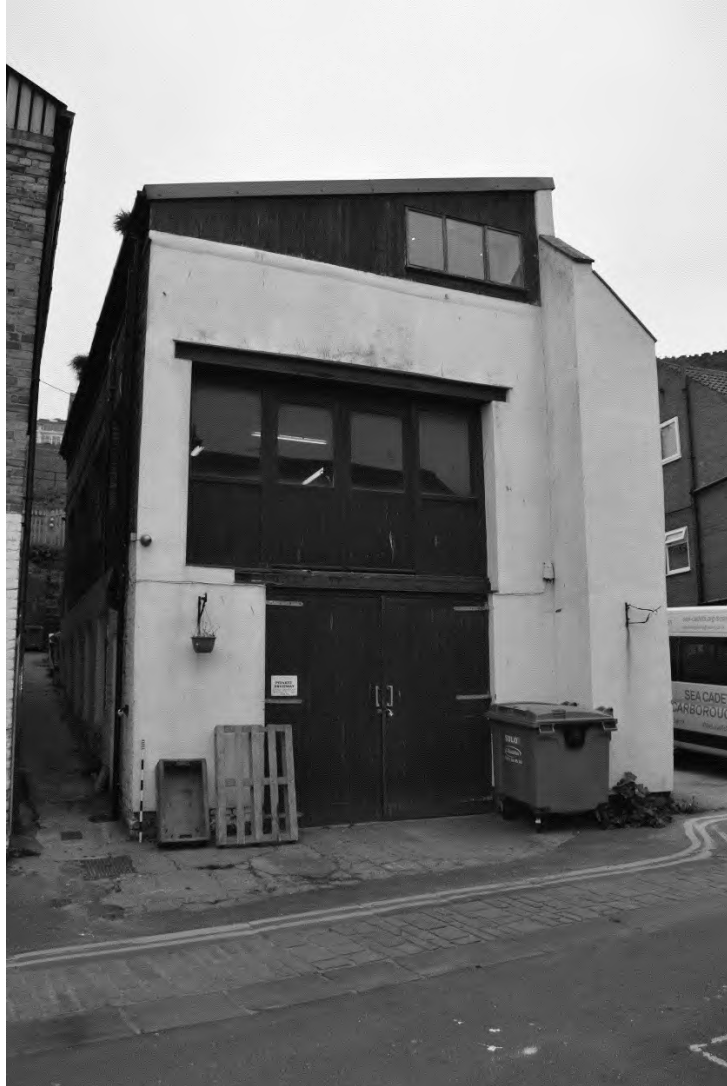
Plate 5. Exterior West & South Elevations (DSC_0670). Facing North-east.
