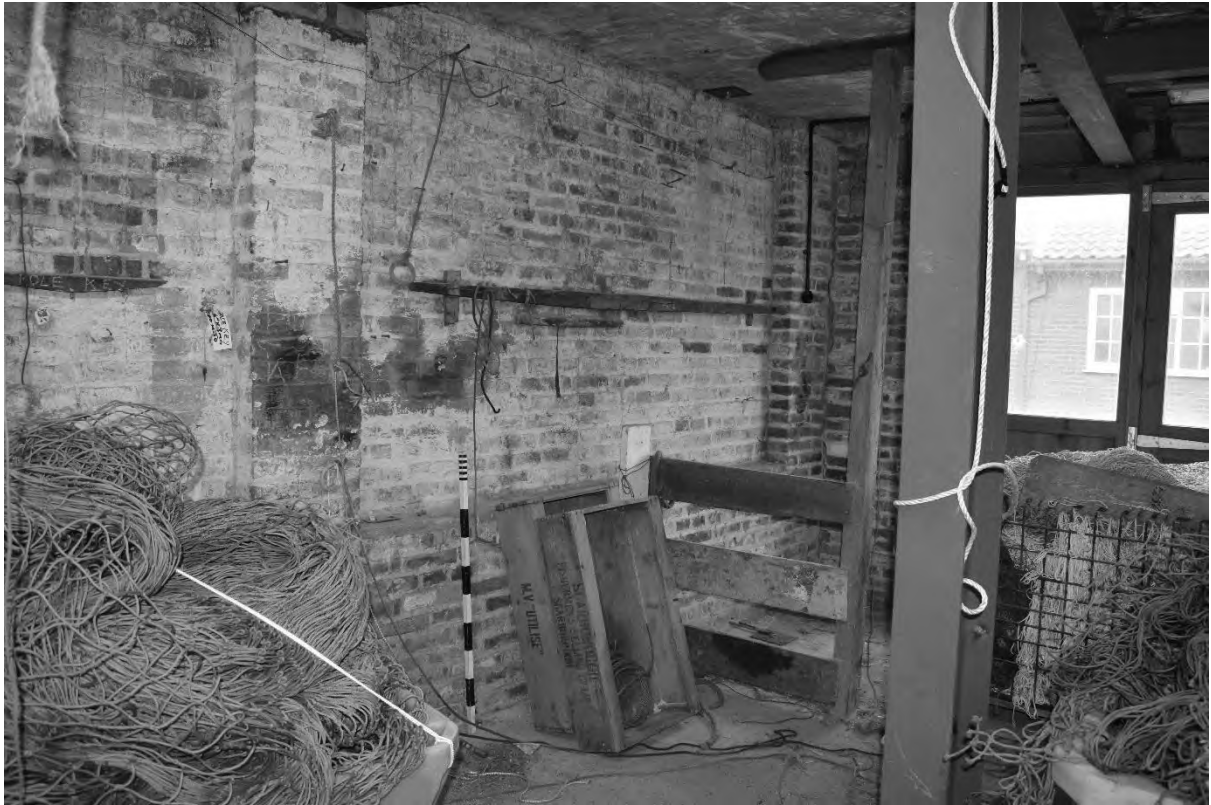
Plate 33. Interior First Floor Workshop (DSC_0636). Facing South-east.
