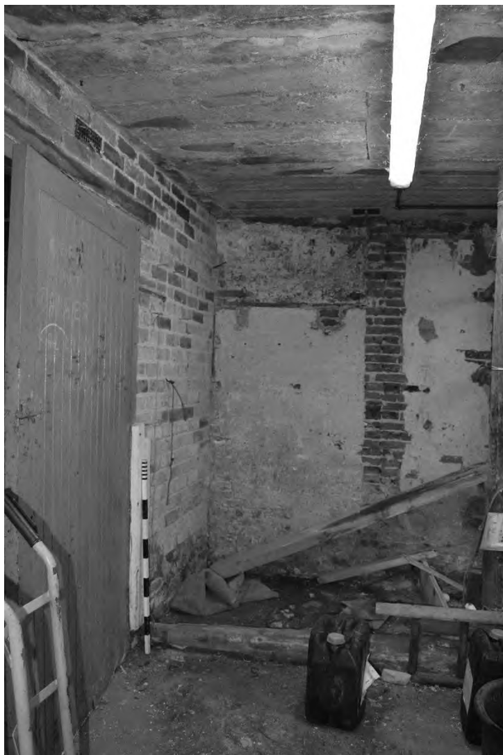
Plate 43. Interior First Floor Workshop: wall scar (DSC_0655). Facing North-east.
