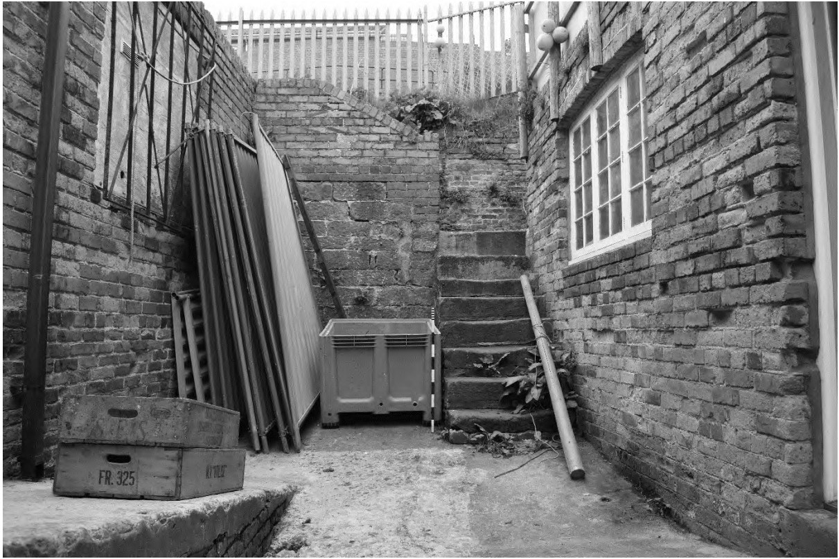
Plate 13. Exterior West Elevation Rear Steps (DSC_0718). Facing North.
