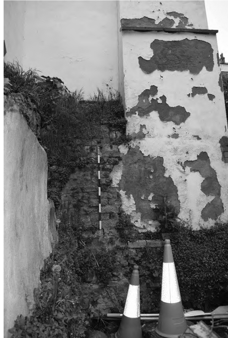
Plate 16. Exterior Buttress (DSC_0678). Facing North.
