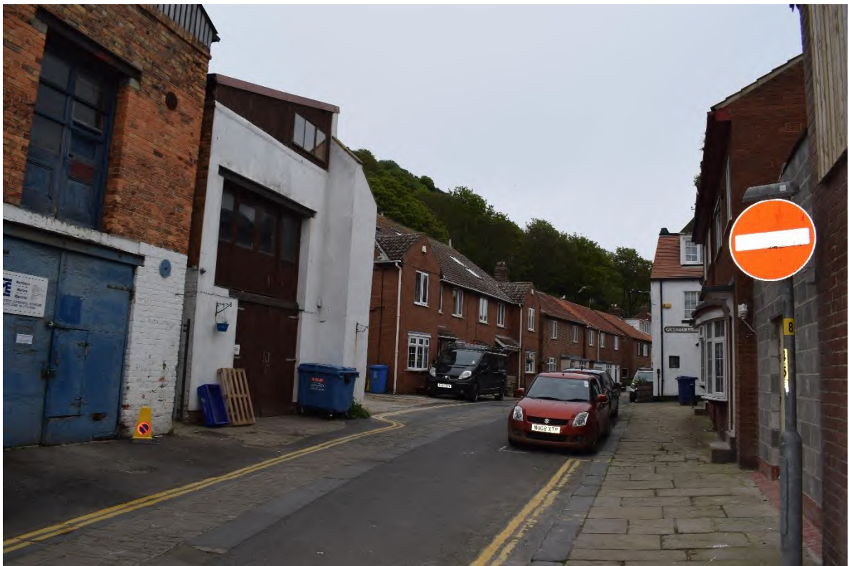
Plate 2. 22a Quay Street (DSC_0697). Facing East.
