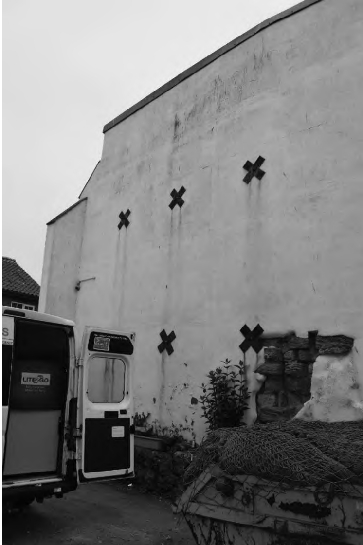
Plate 15. Exterior East Elevation (DSC_0677). Facing South-west.
