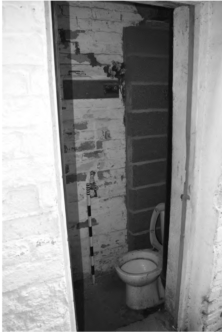
Plate 27. Outside Toilet on Ground Floor (DSC_0698). Facing South-east.
