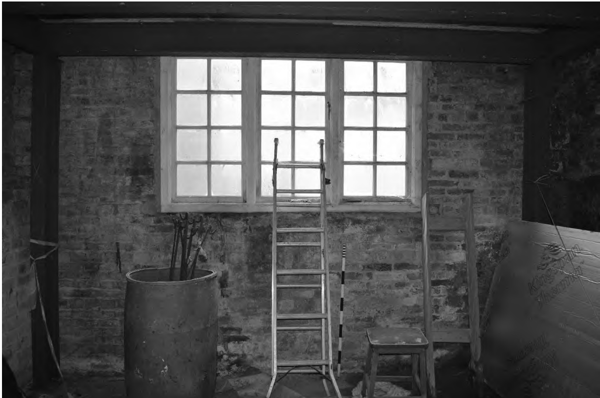
Plate 46. Interior First Floor Store (DSC_0649). Facing West.
