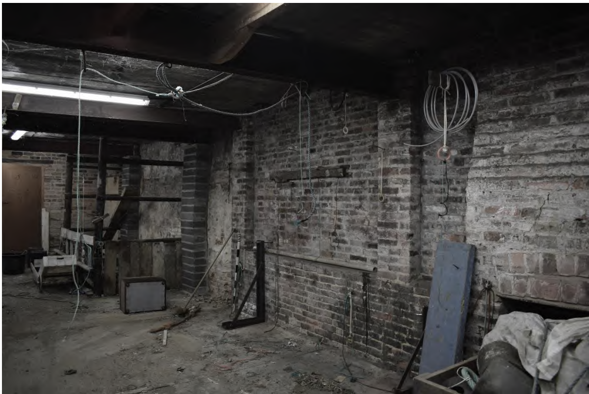
Plate 36. Interior First Floor Workshop (DSC_0642). Facing North-east.
