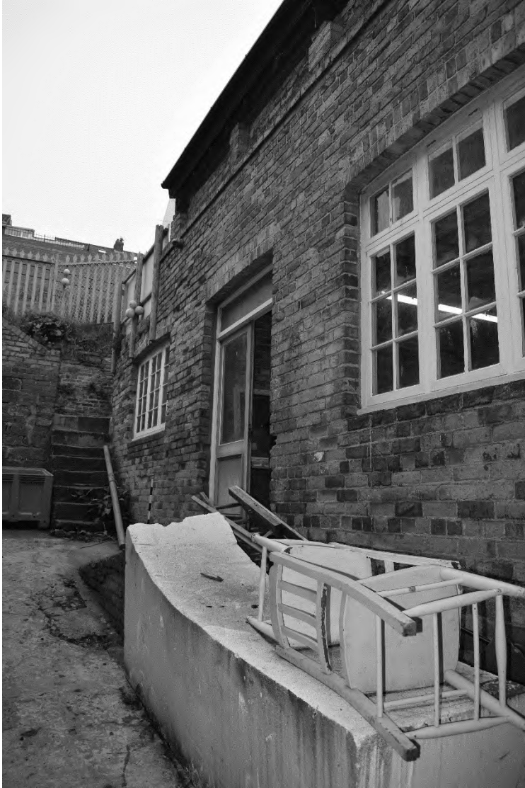
Plate 9. Exterior West Elevation (DSC-656), facing North-east.
