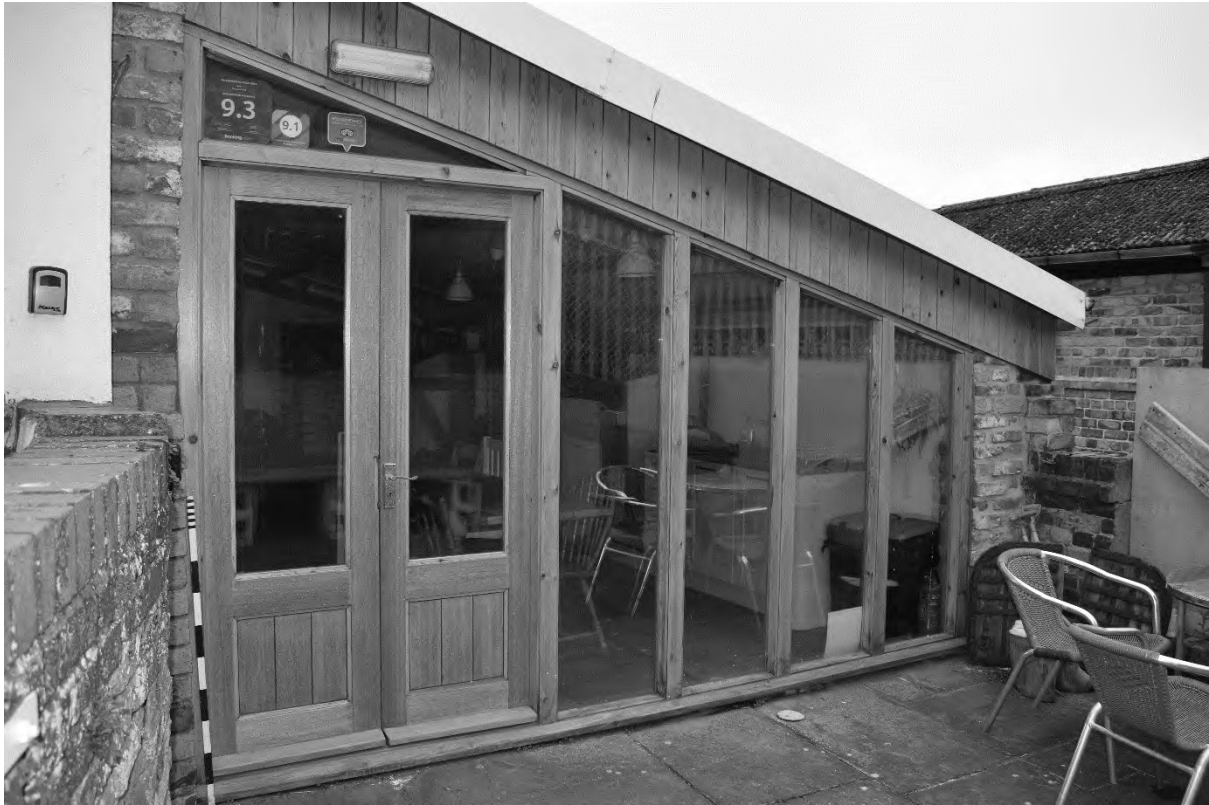
Plate 19. Exterior North Elevation (DSC_0692). Facing North-east.
