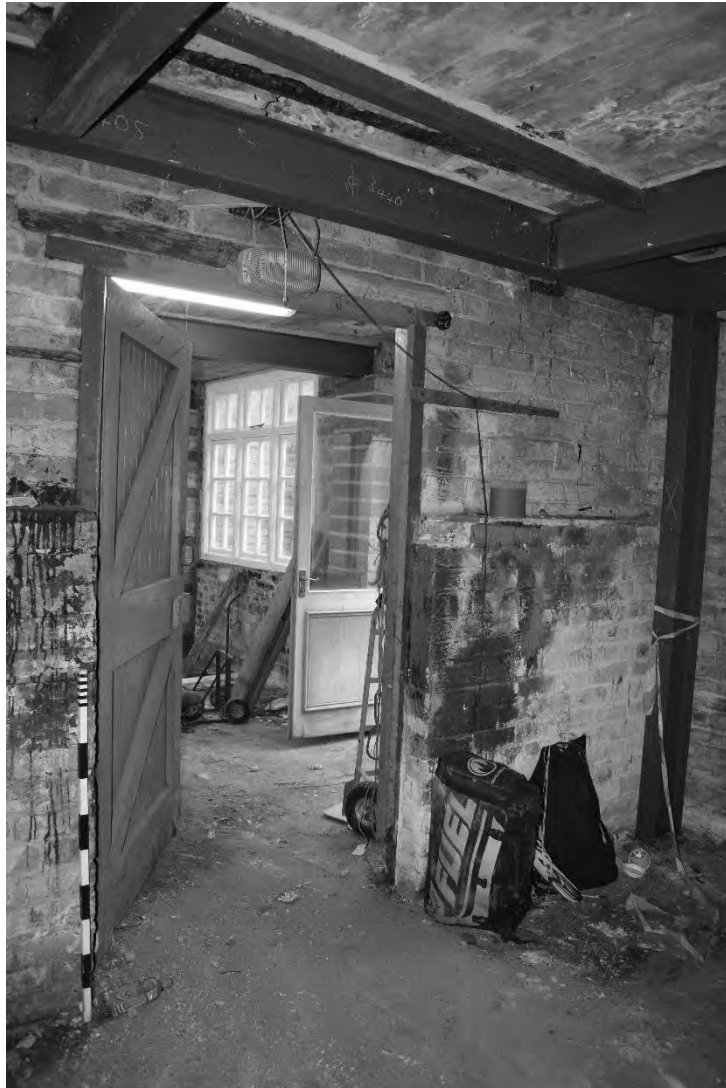
Plate 47. Interior First Floor Store (DSC_0651). Facing South-west.
