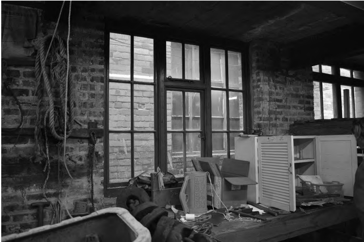
Plate 39. Interior First Floor Workshop (DSC_0717). Facing North-west.
