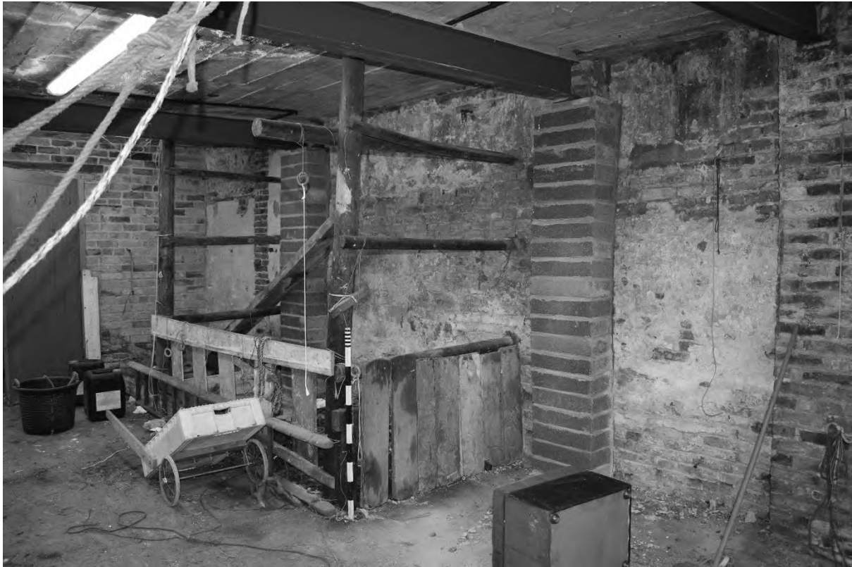
Plate 37. Interior First Floor Workshop (DSC_0644). Facing North-east.
