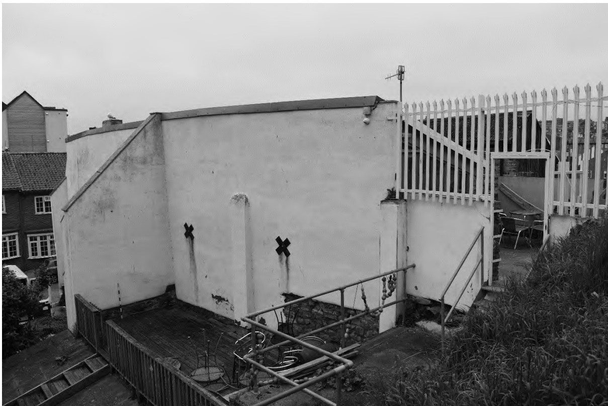
Plate 18. Exterior East Elevation (DSC_0680). Facing South-west.
