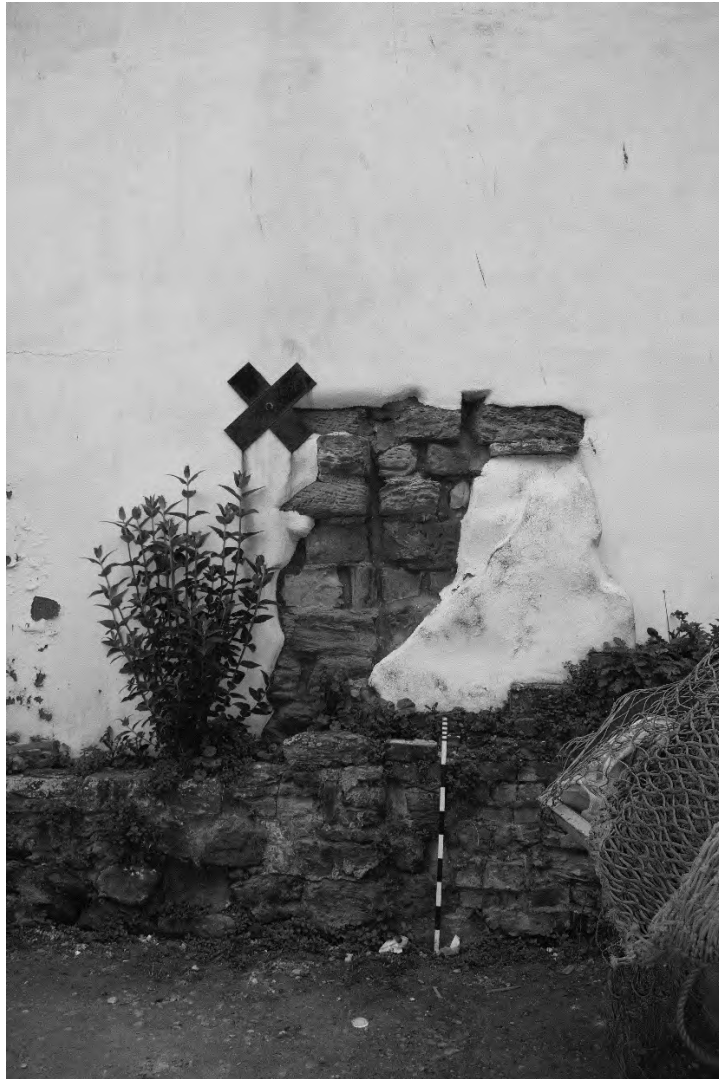
Plate 17. Exterior East Elevation Exposed Stone (DSC_0676). Facing West.
