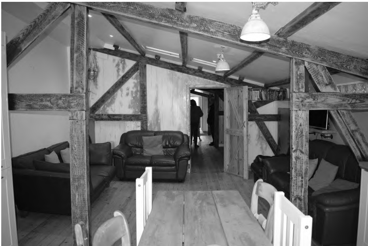
Plate 50. Interior Second Floor Surfer's Hostel (DSC_0707). Facing South.
