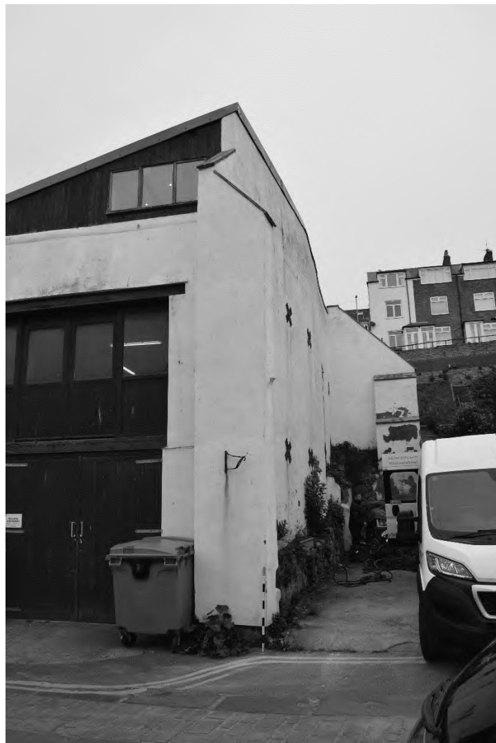
Plate 14. Exterior South & east Elevations (DSC_0673). Facing North-west.
