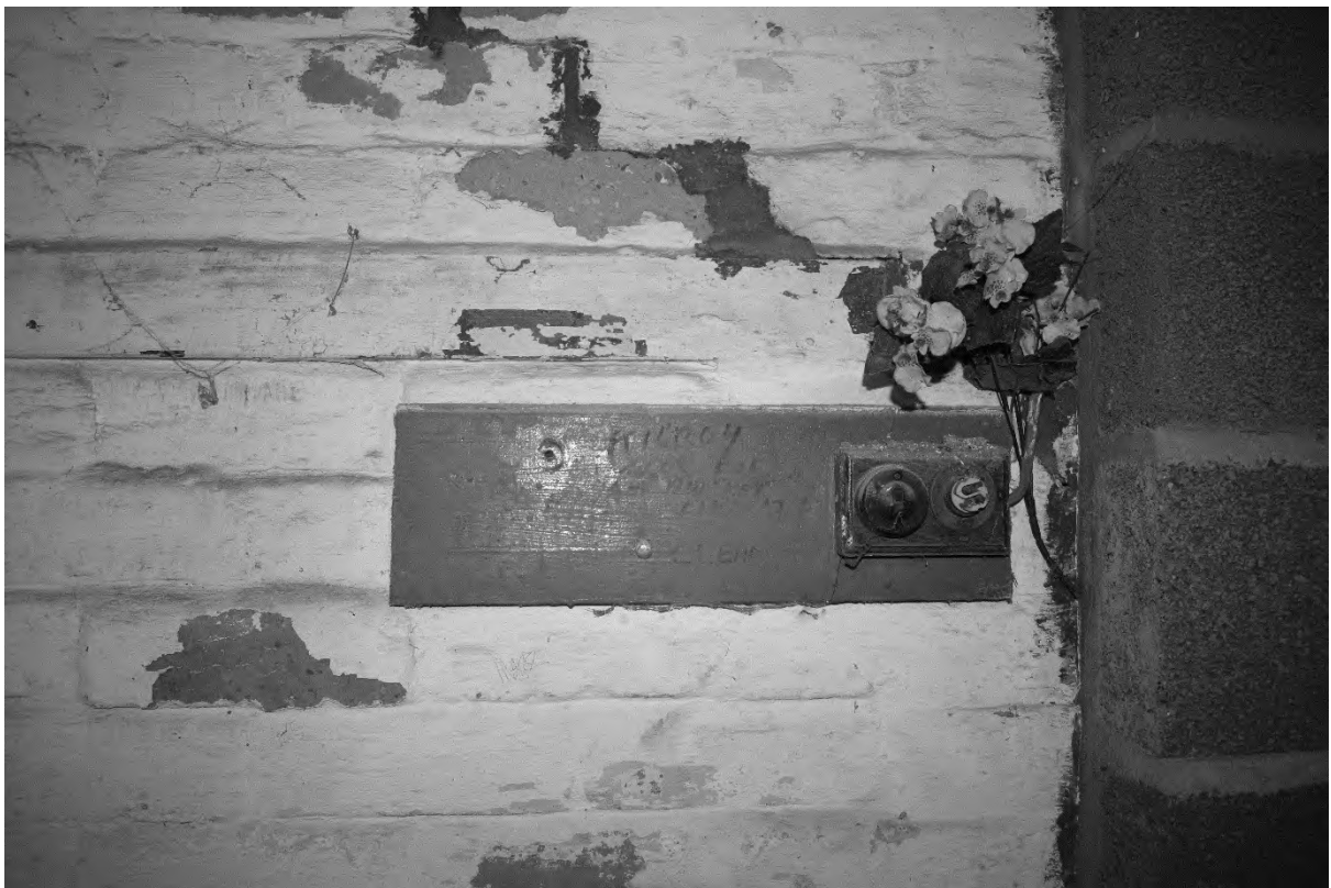
Plate 30. Bakelite Light switch & Socket (DSC_703). Facing East.
