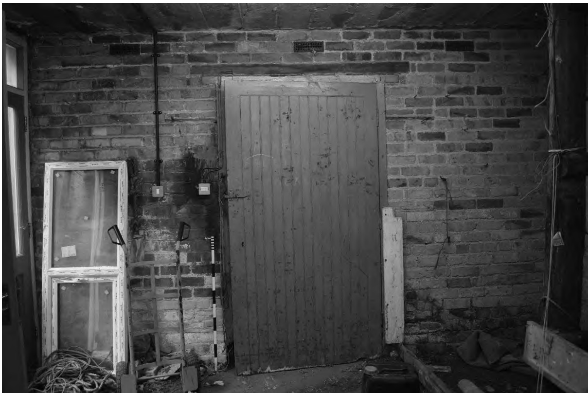
Plate 42. Interior First Floor Workshop Door to Rear Store (DSC_0645). Facing North.
