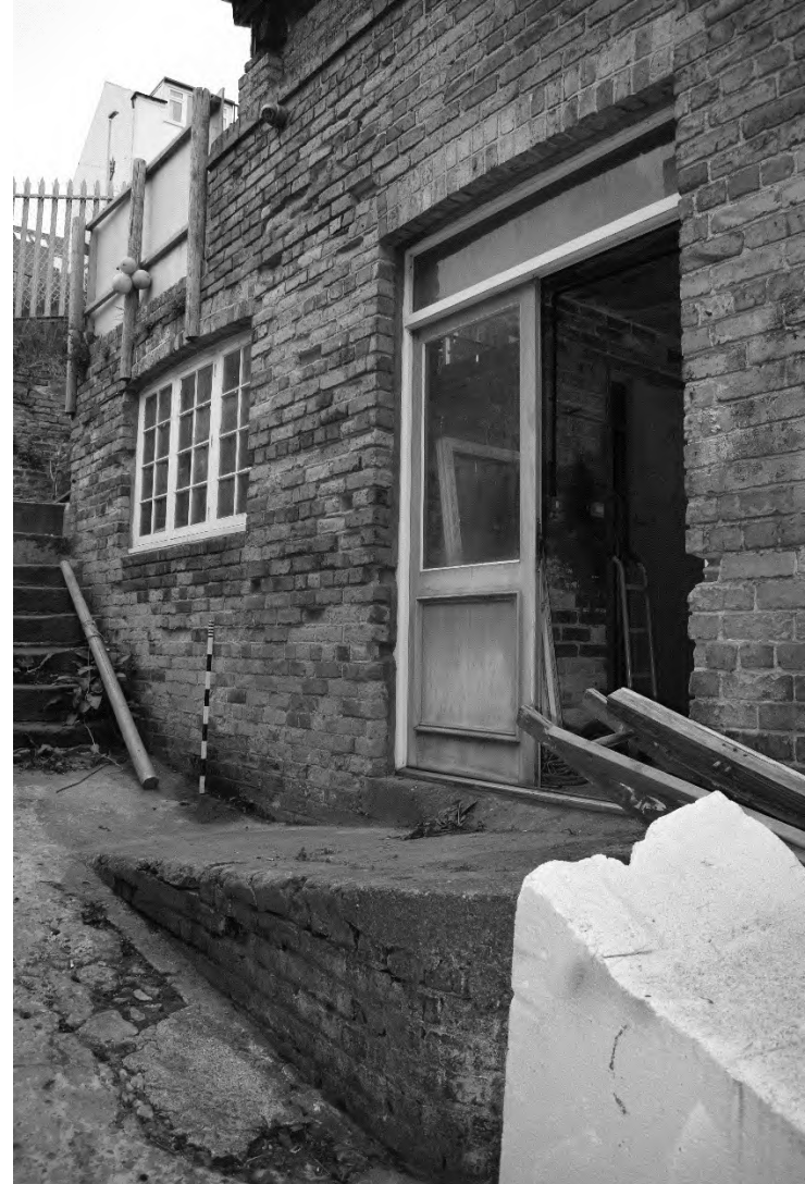
Plate 12. Exterior West Elevation Access (DSC_0657). Facing North-east.
