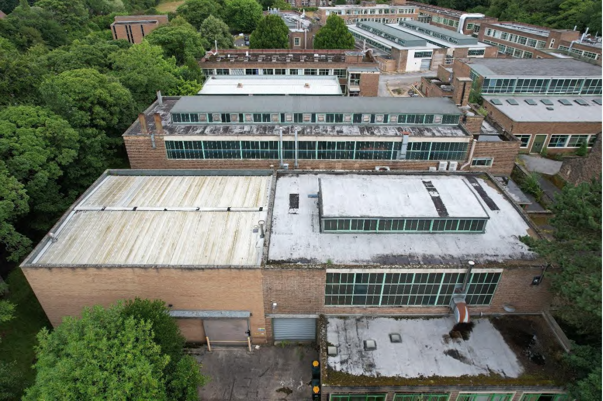
Plate 41. Blocks G & F from Drone (DJI_0219). Facing East.
