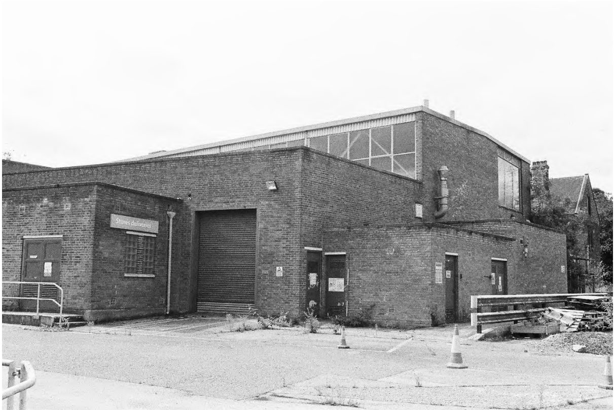
Plate 65. Block L: Exterior North & West Elevations (Swinden11_25). Facing South-west.
