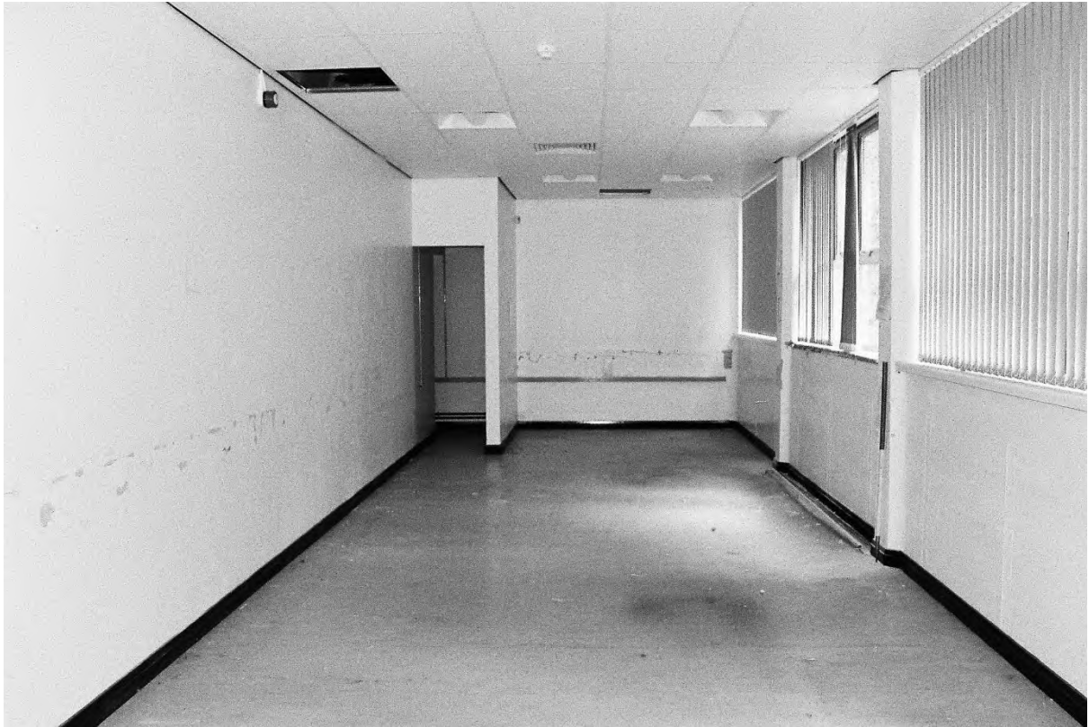
Plate 209. Block K: Interior Ground Floor Room K9 (Swinden8_07). Facing East.
