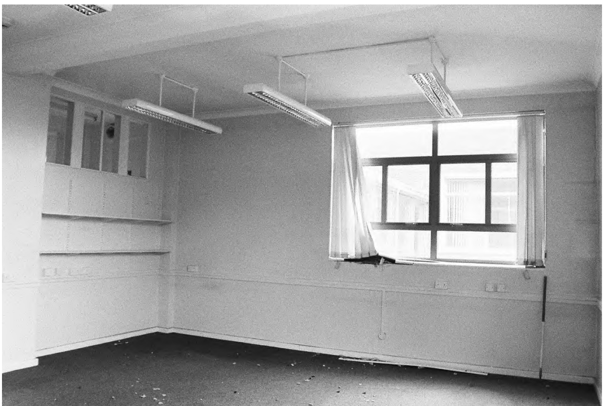
Plate 120. Block A: Interior First Floor Room A54 (Swinden2_23). Facing West.
