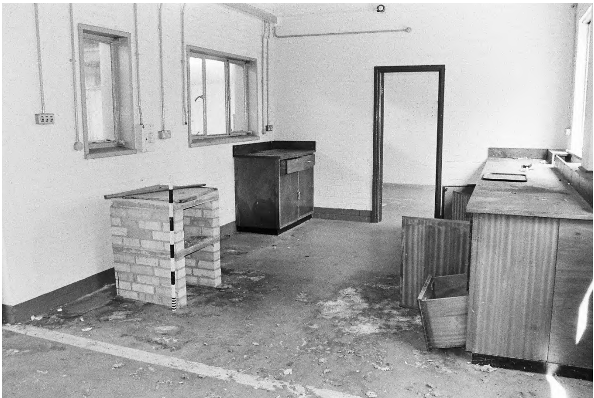
Plate 170. Block D: Interior Room D214 (Swinden6_04). Facing East.
