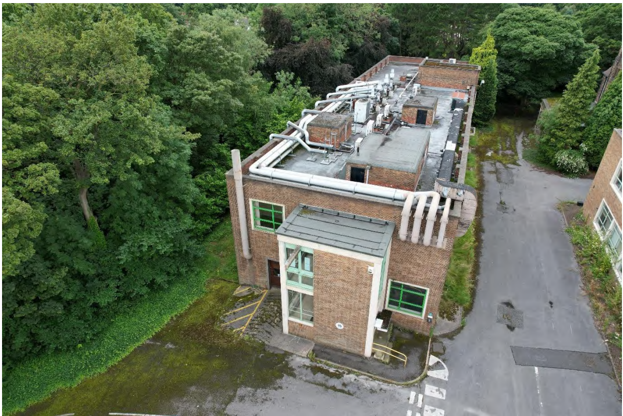
Plate 52. Block K from Drone (DJI_0166). Facing West.
