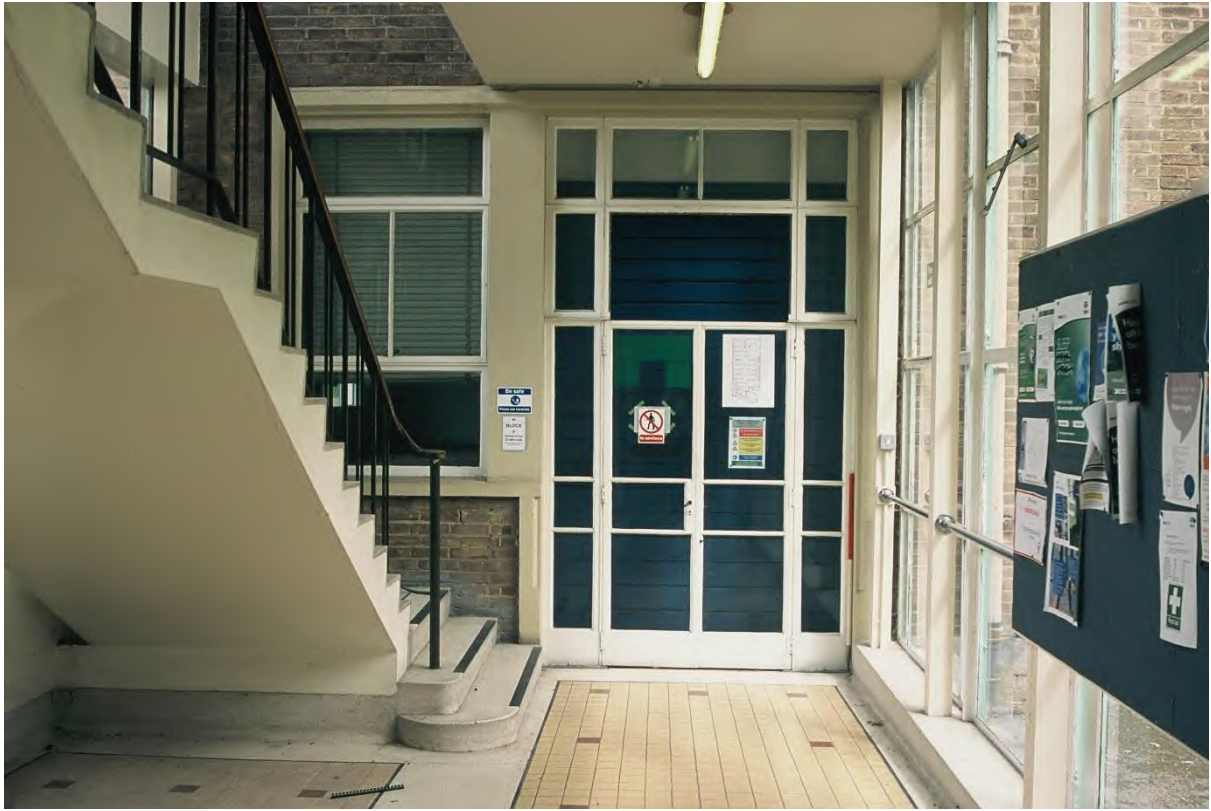
Plate 113. Blocked Entrance to Block A South (Swinden5_01). Facing North.
