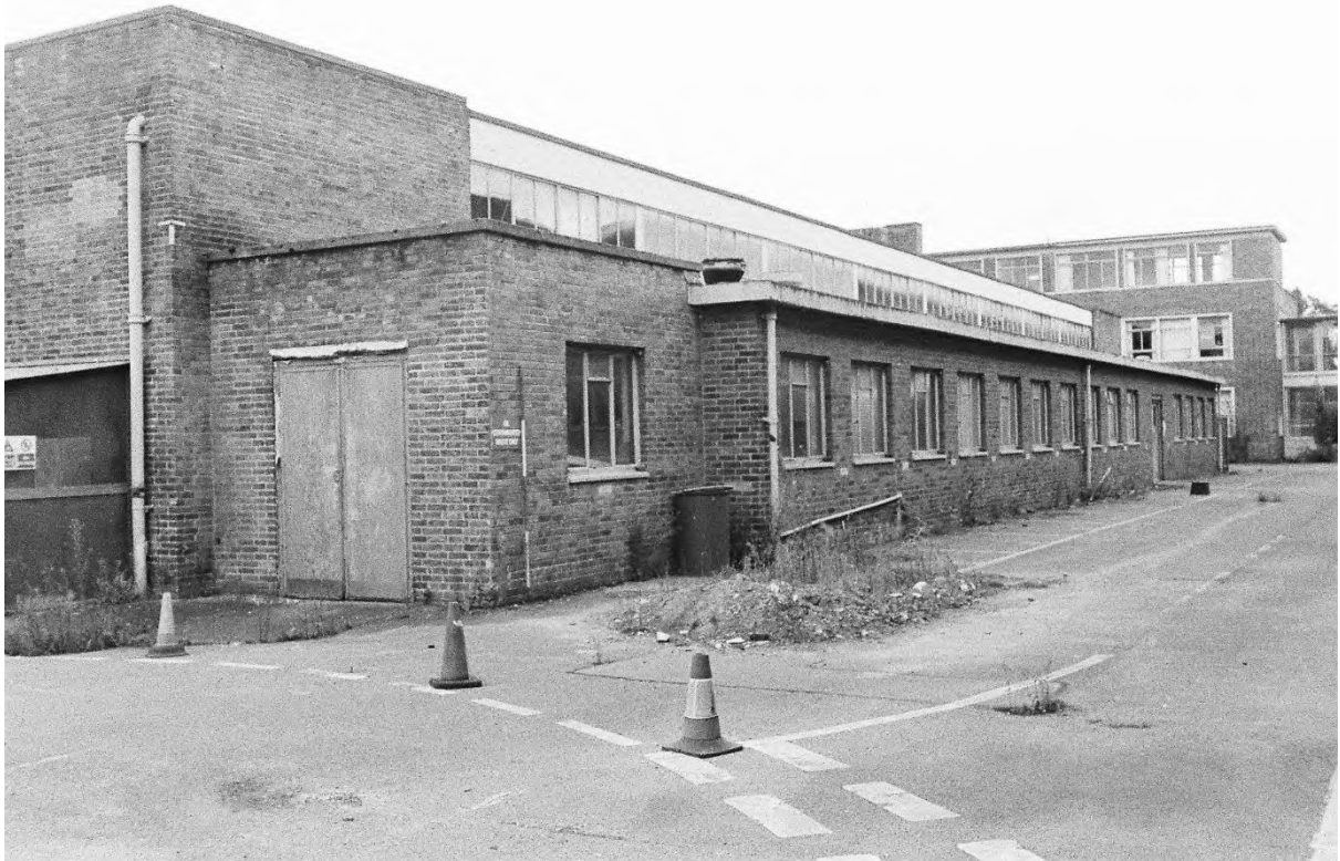
Plate 33. Block D: Exterior South Elevation (Swinden9_35). Facing North-east.
