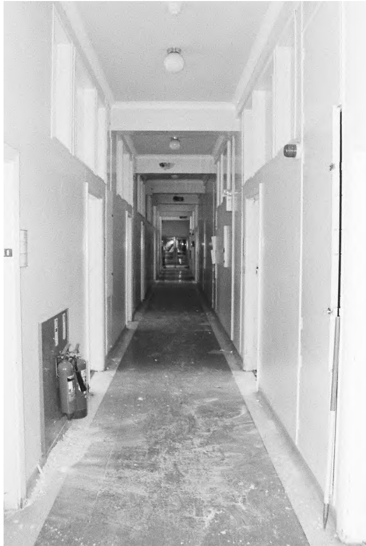
Plate 123. Block H: Interior Ground Floor Corridor (Swinden2_27). Facing West.
