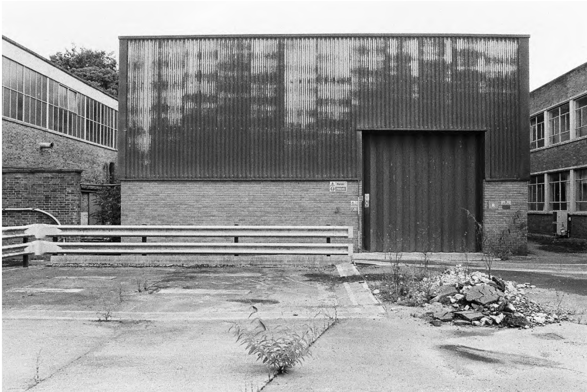
Plate 73. Block R: Exterior South Elevation (Swinden11_10). Facing North.
