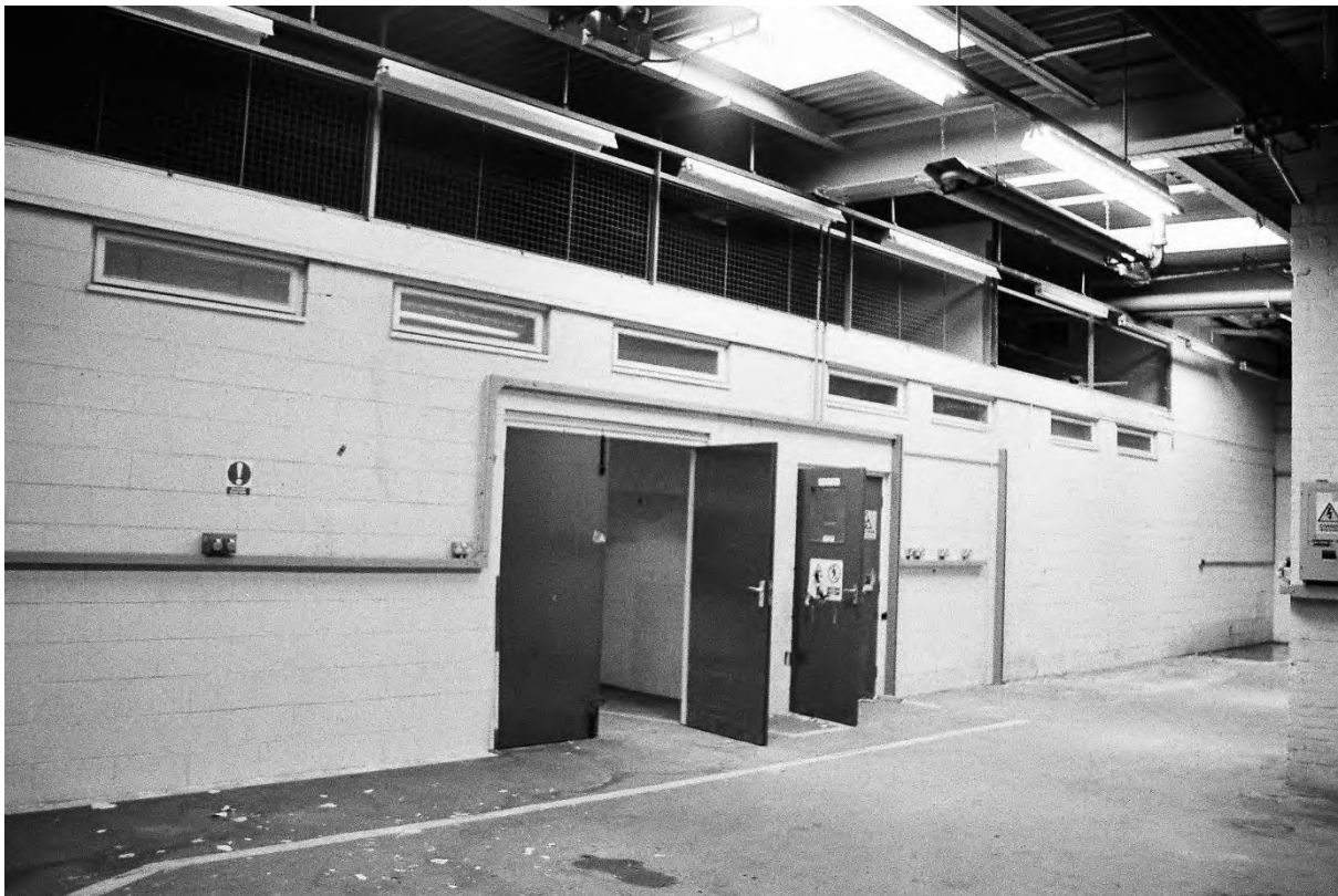
Plate 238. Block L: Interior Ground Floor Room L18 (Swinden8_32). Facing North-west.
