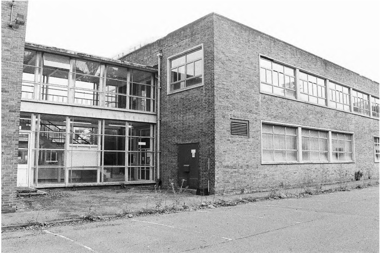
Plate 13. Block A: Exterior West & South Elevations (Swinden9_21). Facing North-east.
