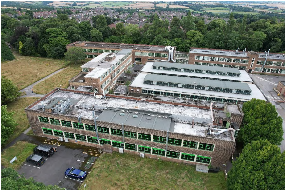
Plate 19. Block B from Drone (DJI_0072). Facing South.
