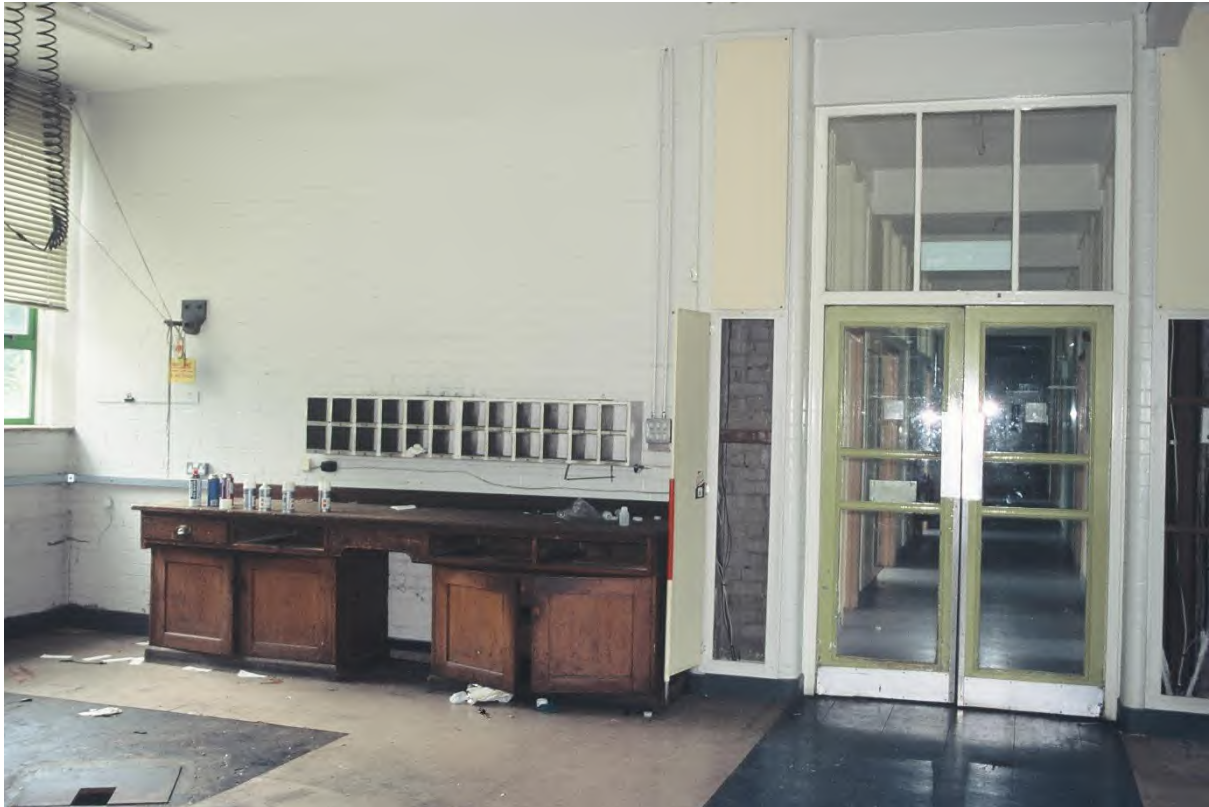
Plate 107. Block A: Interior Ground Floor Room A2 (Swinden5_09). Facing South-west.
