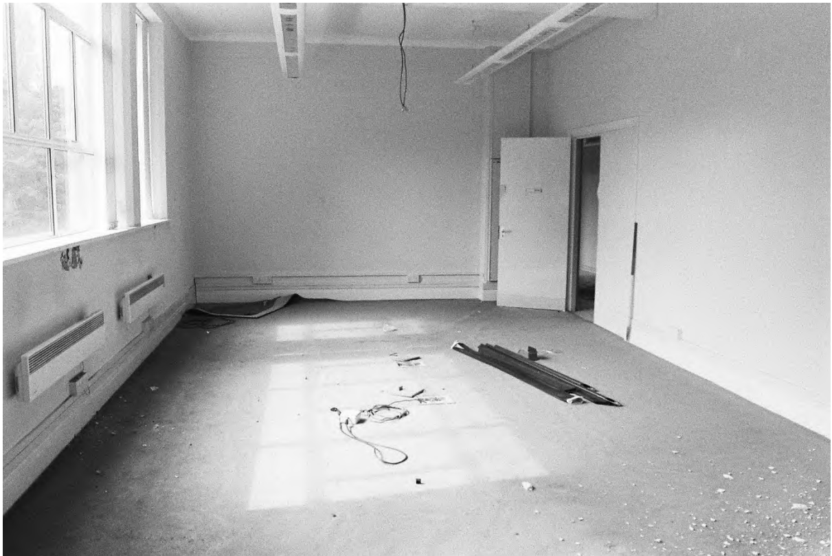
Plate 119. Block A: Interior First Floor Room A27 (Swinden2_16). Facing West.
