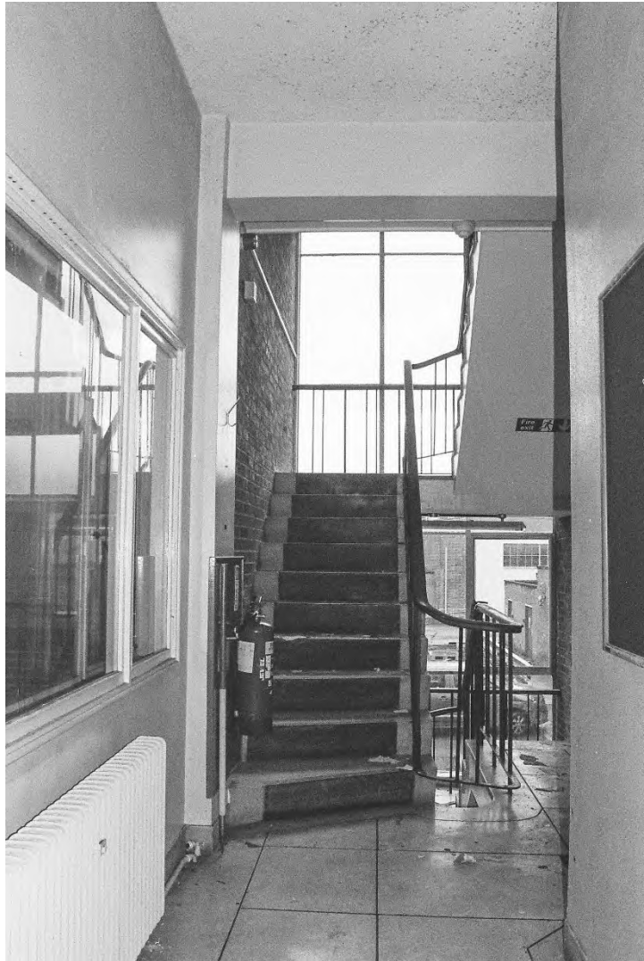
Plate 177. Block F: Interior First Floor Room F4 (Swinden6_21). Facing East.
