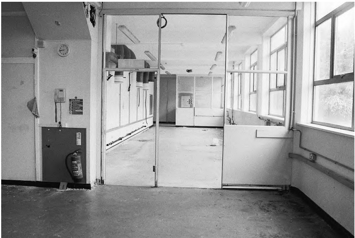
Plate 210. Block K: Interior Ground Floor Room K2/K8/K10 (Swinden7_37). Facing West.
