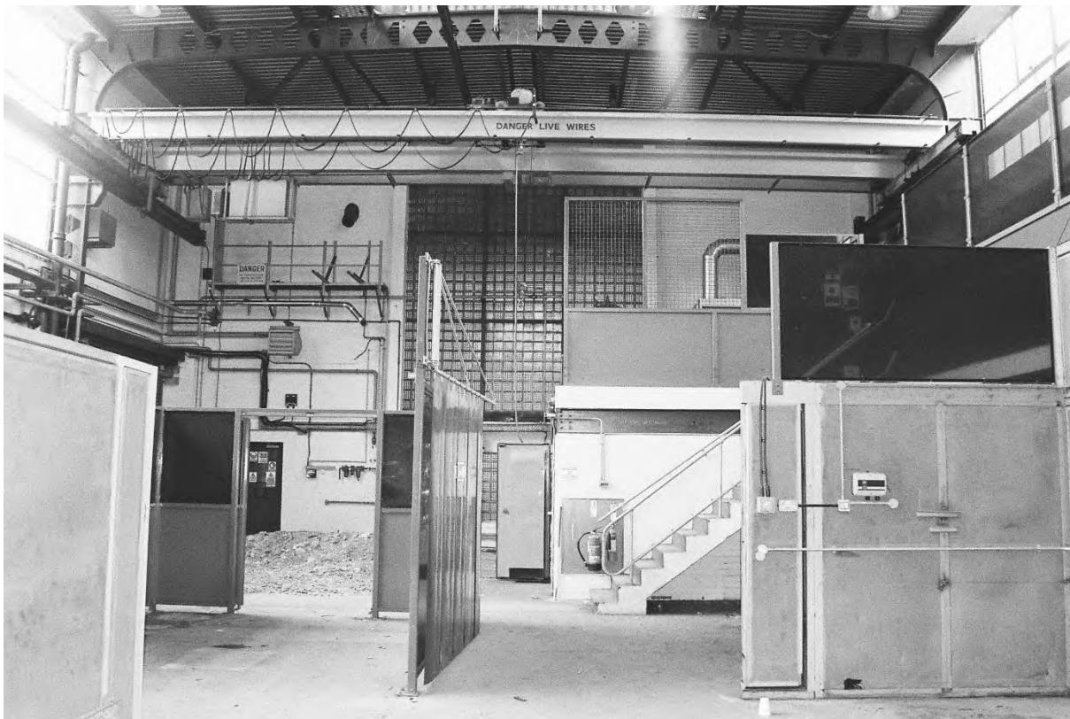
Plate 186. Block G: Interior Room G1 (Swinden6_32). Facing North.
