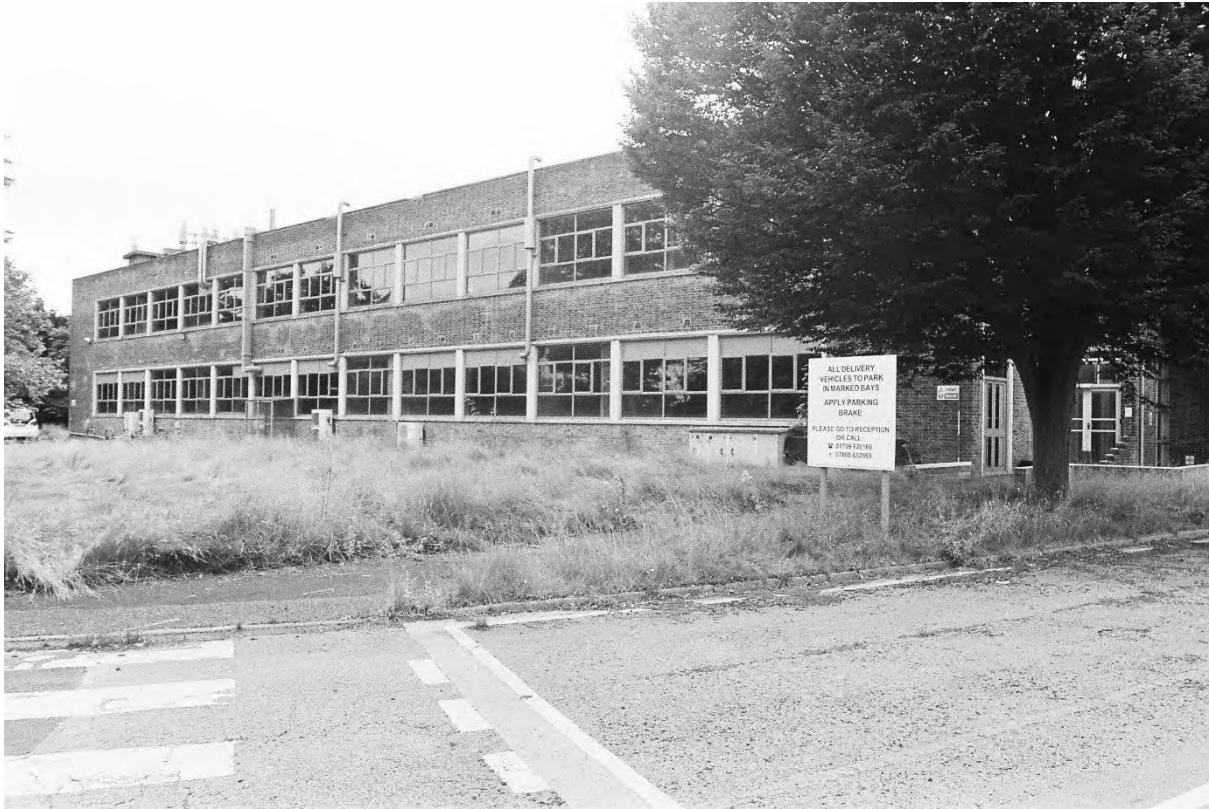
Plate 23. Block B: Exterior North Elevation (Swinden10_07). Facing South-east.
