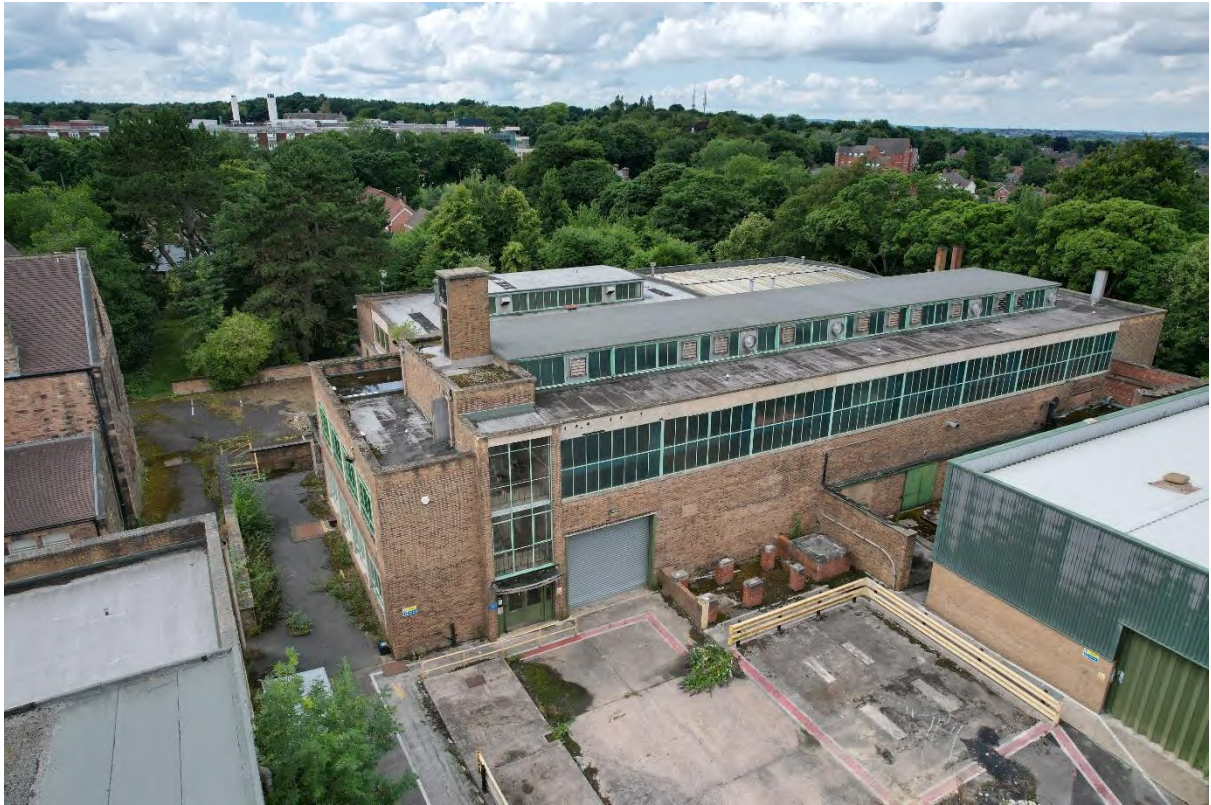
Plate 35. Block F from Drone (DJI_0213). Facing West.
