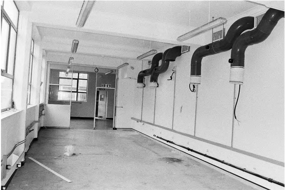
Plate 211. Block K: Interior Ground Floor Room K2/K8 (Swinden8_03). Facing East.
