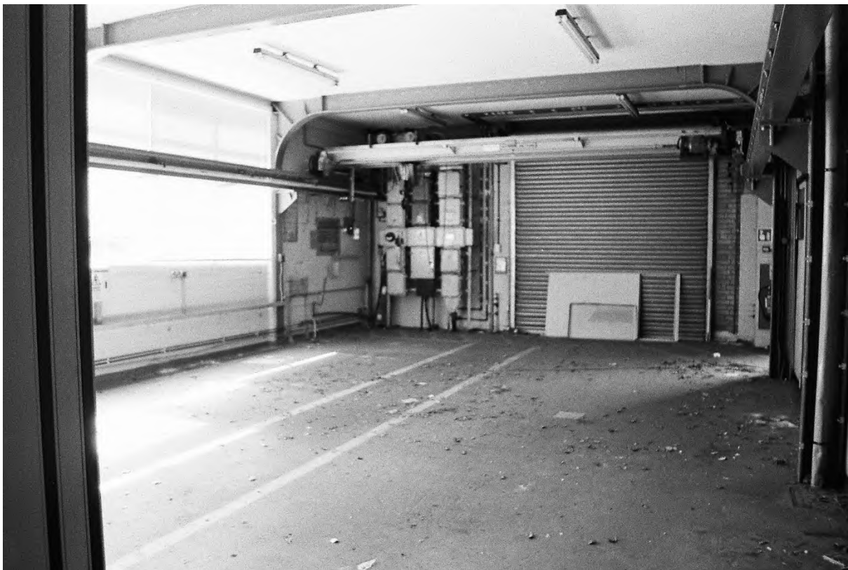
Plate 132. Block H: Interior Ground Floor Room H12 (Swinden3_06). Facing West.
