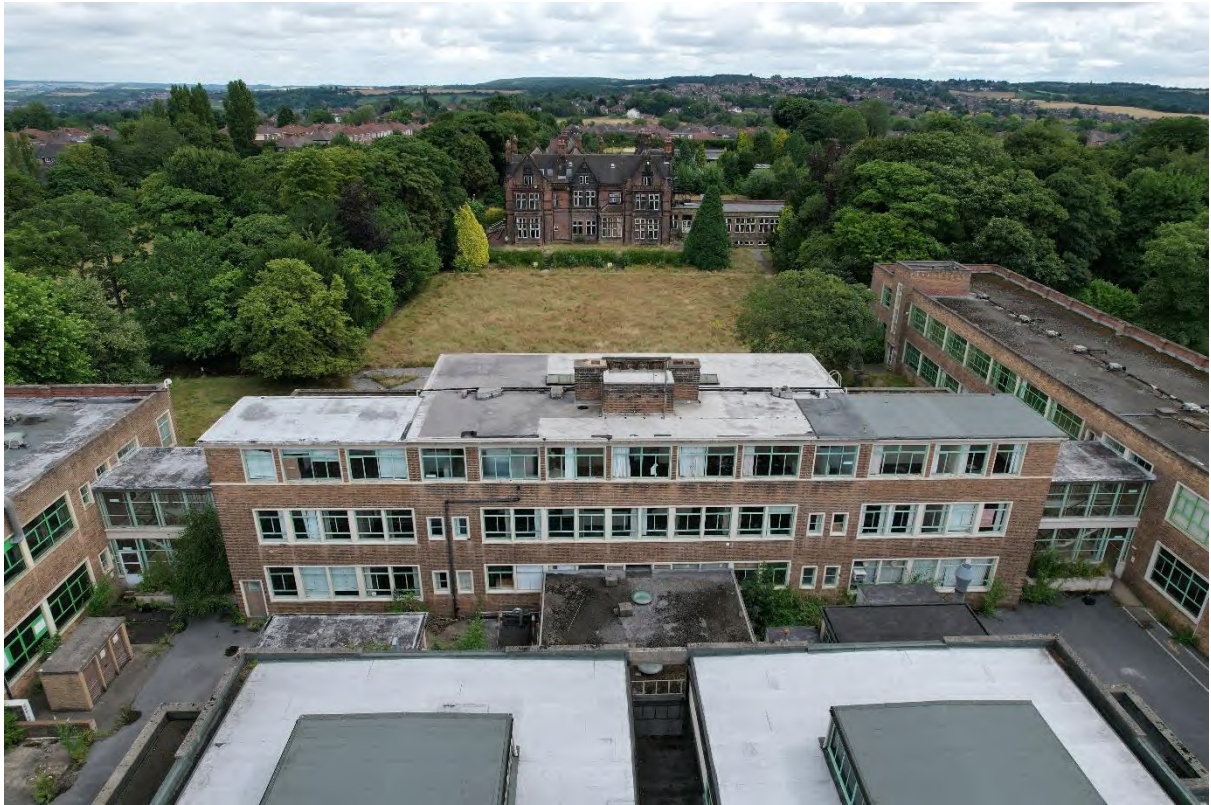
Plate 3. Block C from Drone (DJI_0075). Facing East.
