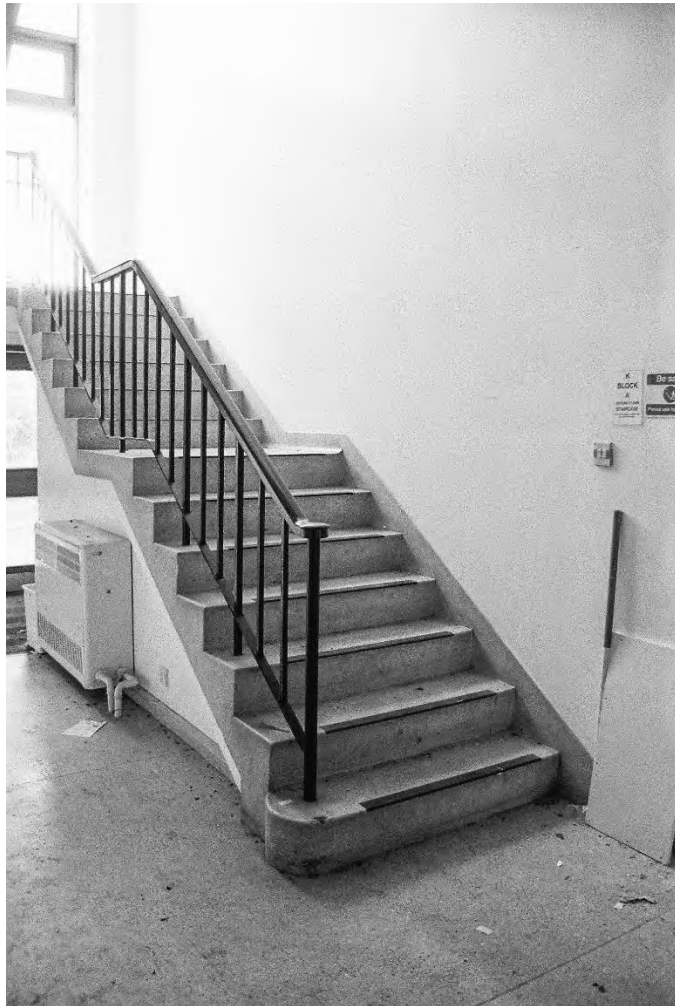
Plate 205. Block K: Interior Ground Floor Corridor (Swinden7_30). Facing North-east.
