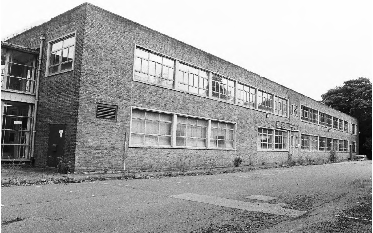
Plate 12. Block A: Exterior South Elevation (Swinden9_19). Facing North-east.
