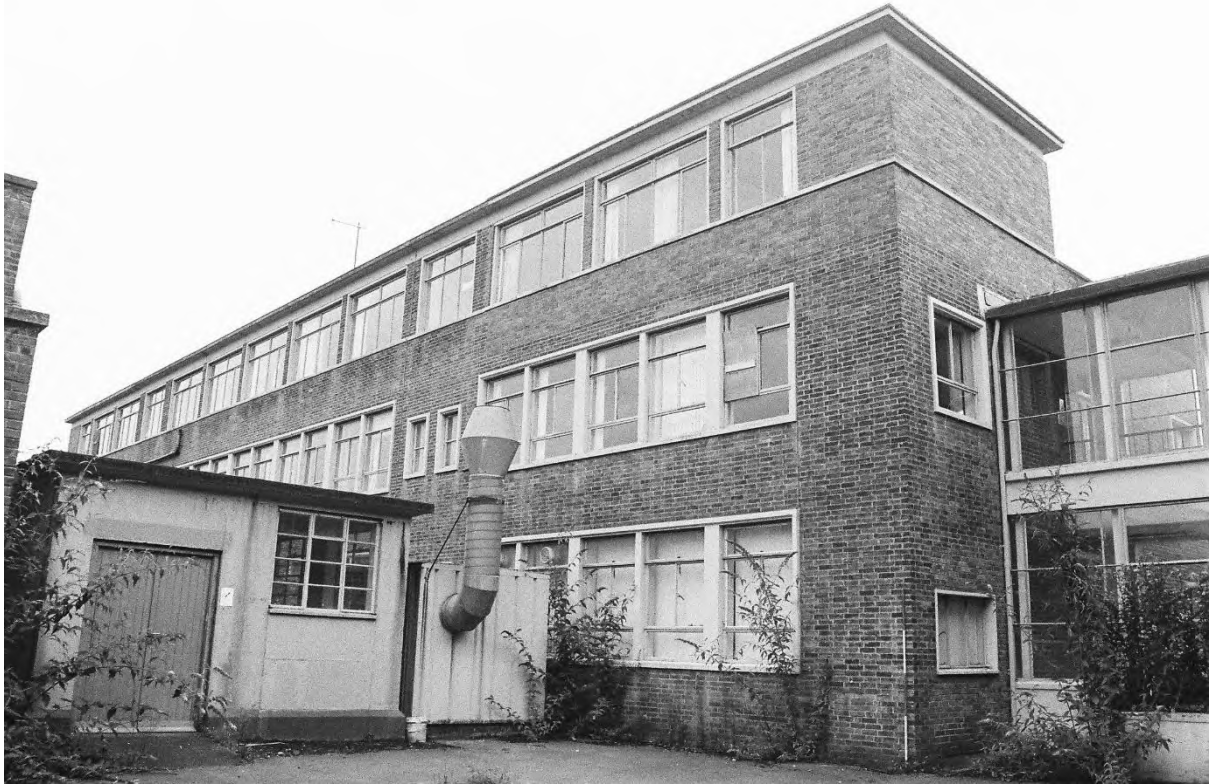
Plate 7. Block C: Exterior West Elevation (Swinden9_33). Facing North-east.
