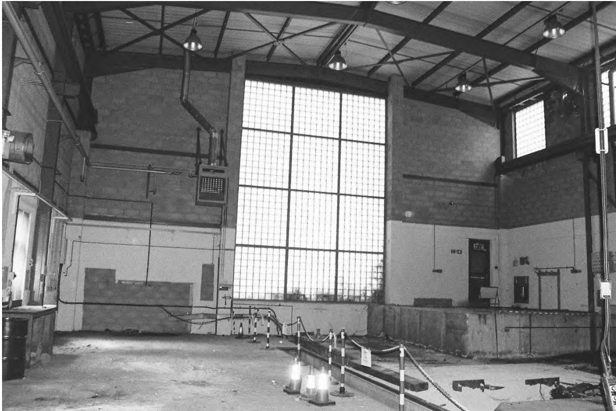
Plate 187. Block G Extension: Room G15 (Swinden6_35). Facing North.
