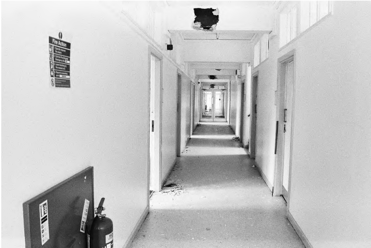
Plate 89. Block C: Interior First Floor Corridor (Swinden11_25). Facing South.
