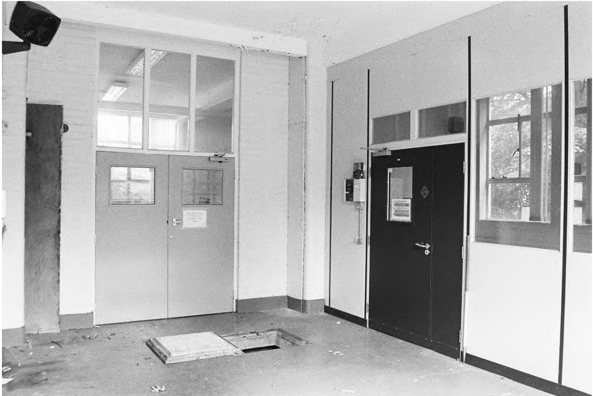
Plate 105. Block A: Interior Ground Floor Room A1 (Swinden2_08). Facing North-east.
