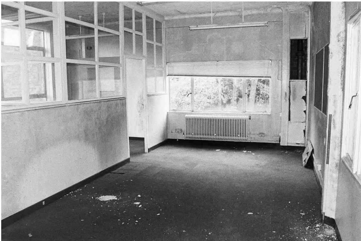
Plate 178. Block F: Interior First Floor Room F3 (Swinden6_22). Facing West.
