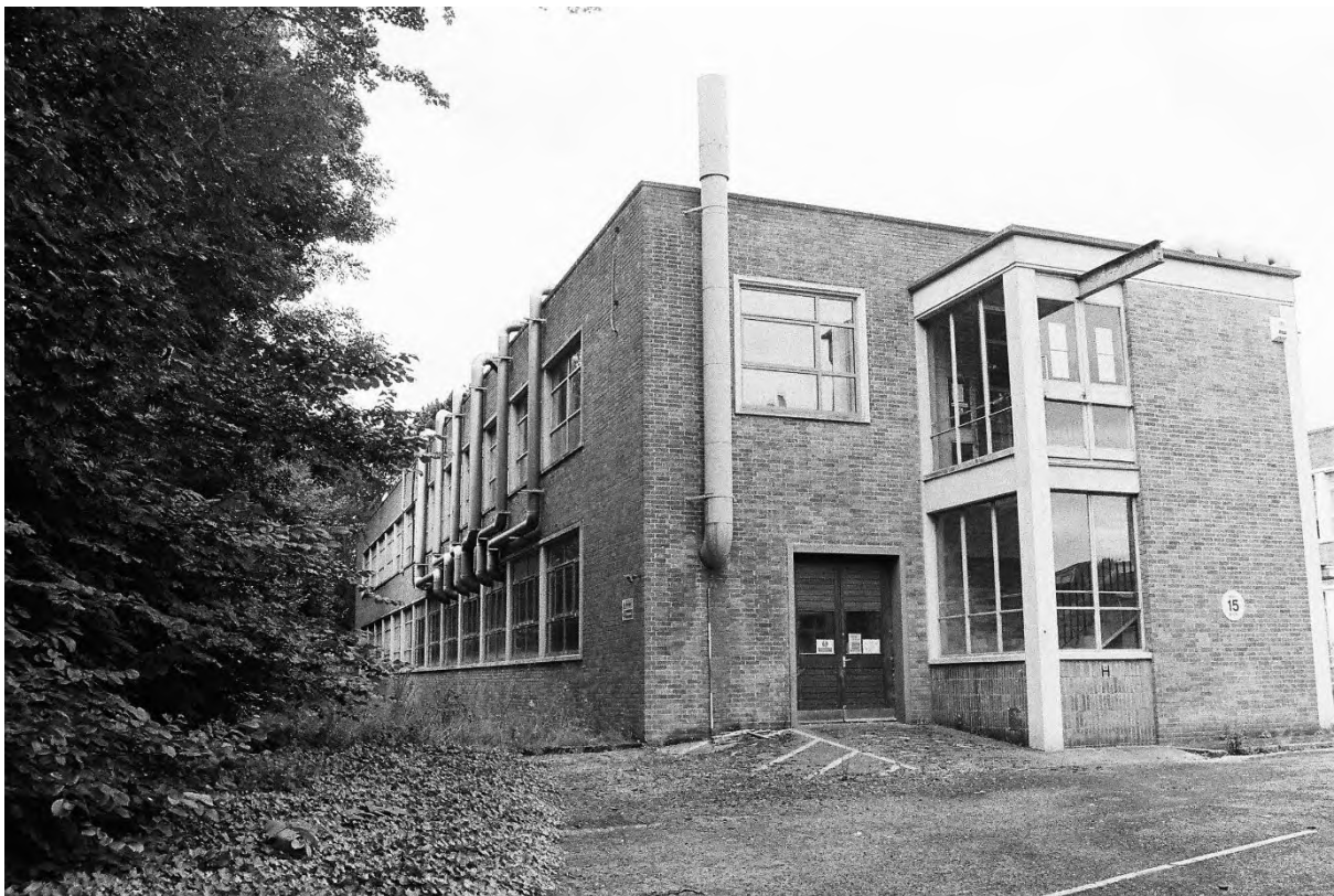
Plate 56. Block K: Exterior East & South Elevations (Swinden11_15). Facing West.
