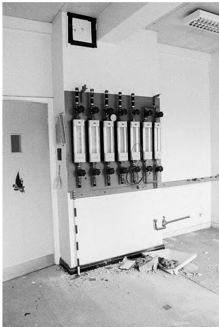
Plate 194. Block J: Interior Ground Floor Room J14 (Swinden7_16). Facing North-west.
