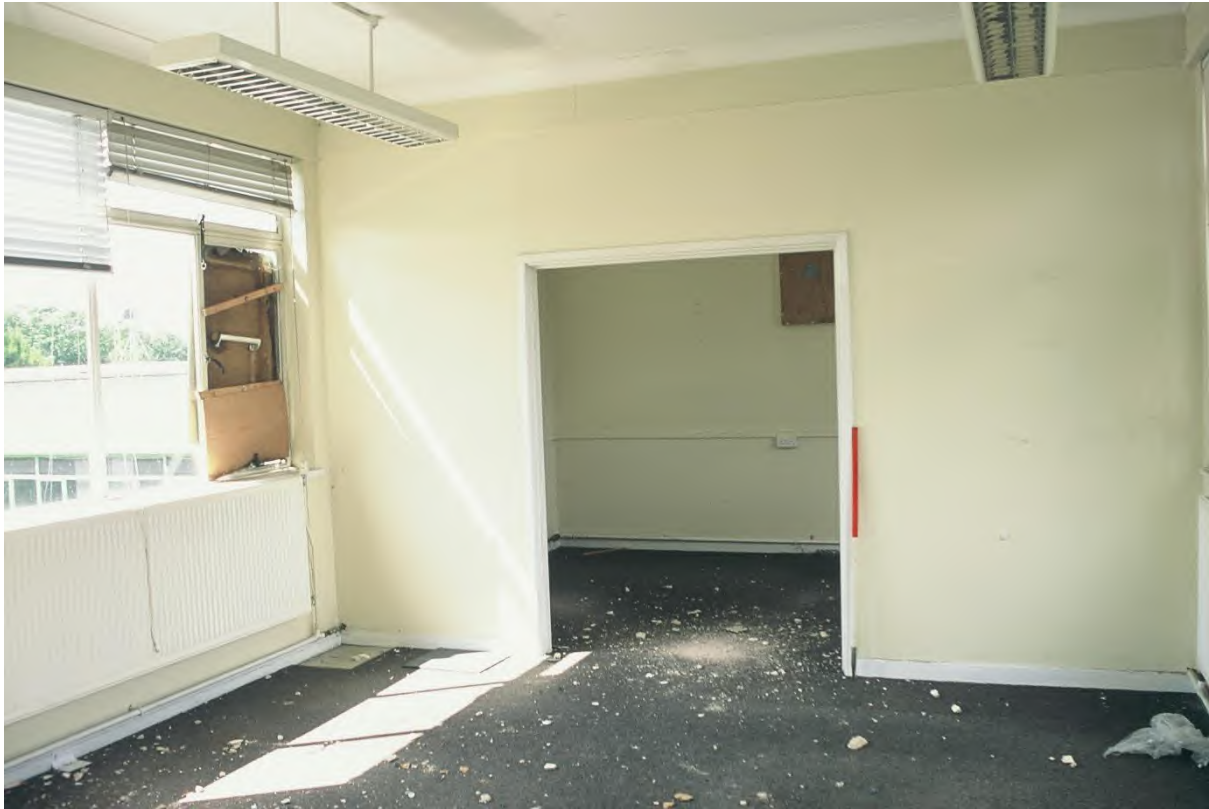
Plate 101. Block C: Interior Second Floor Room 152/152A (Swinden5_17). Facing North.
