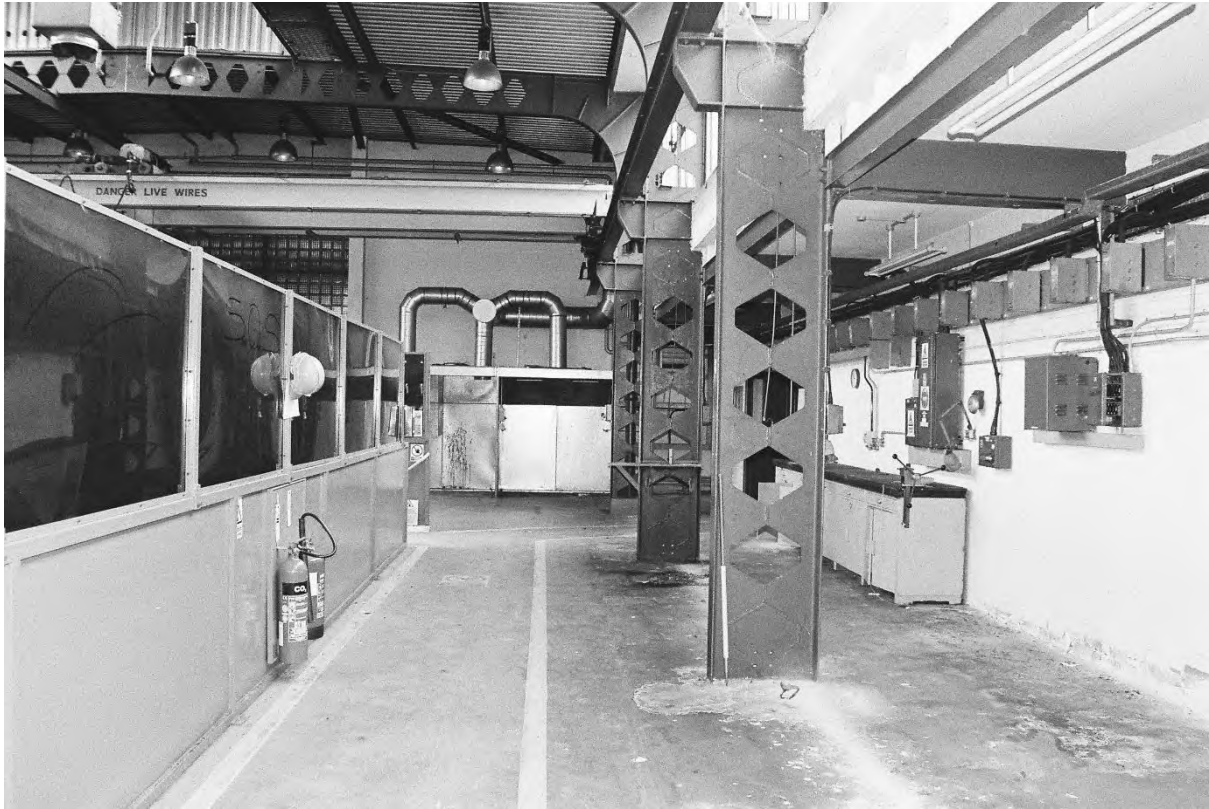
Plate 181. Block G: Interior Mezzanine (Swinden6_25). Facing North.
