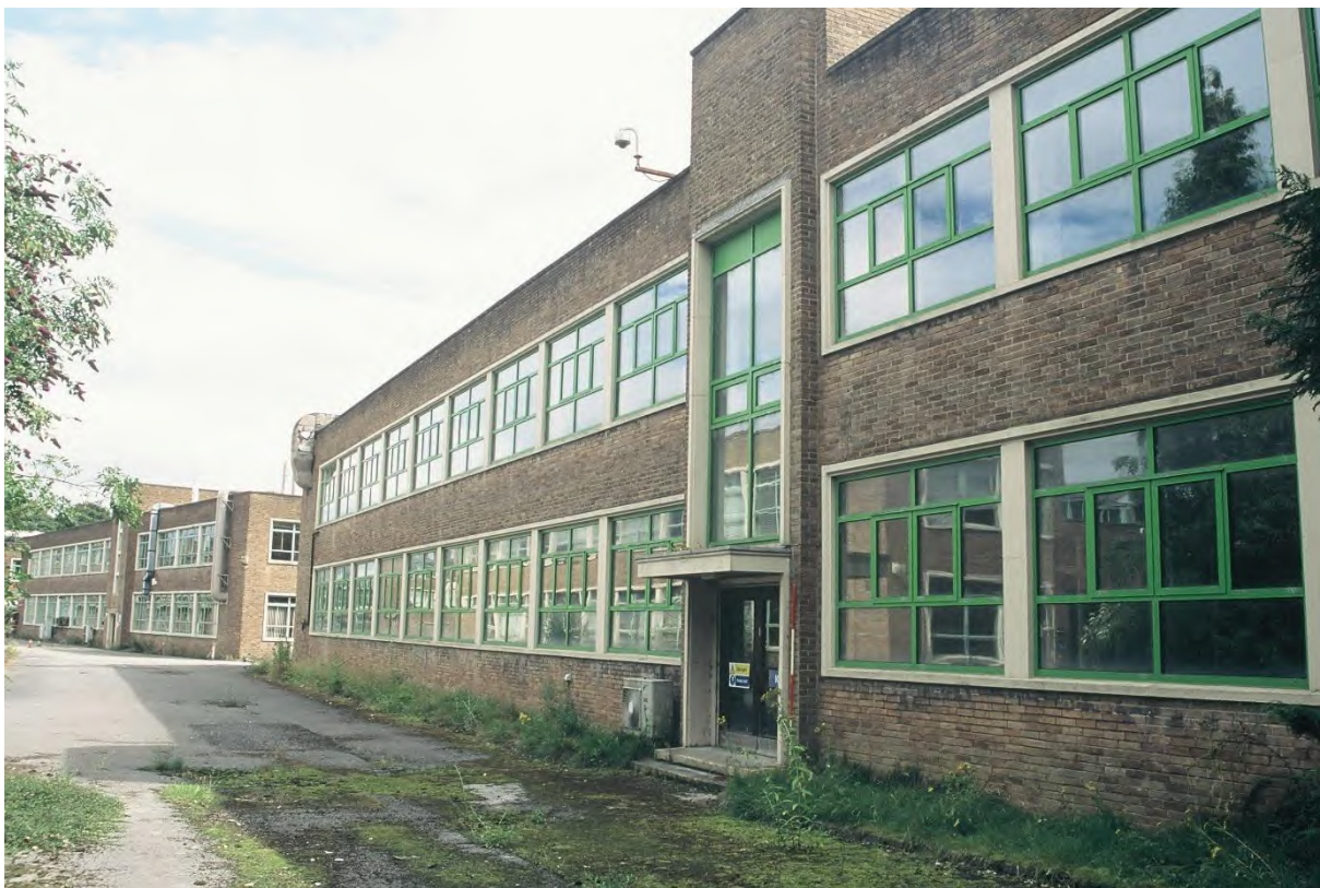
Plate 54. Block K: Exterior North Elevation (Swinden13_12). Facing East.
