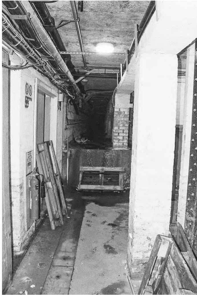
Plate 127. Block H: Interior Basement Duct (Swinden7_22). Facing North.
