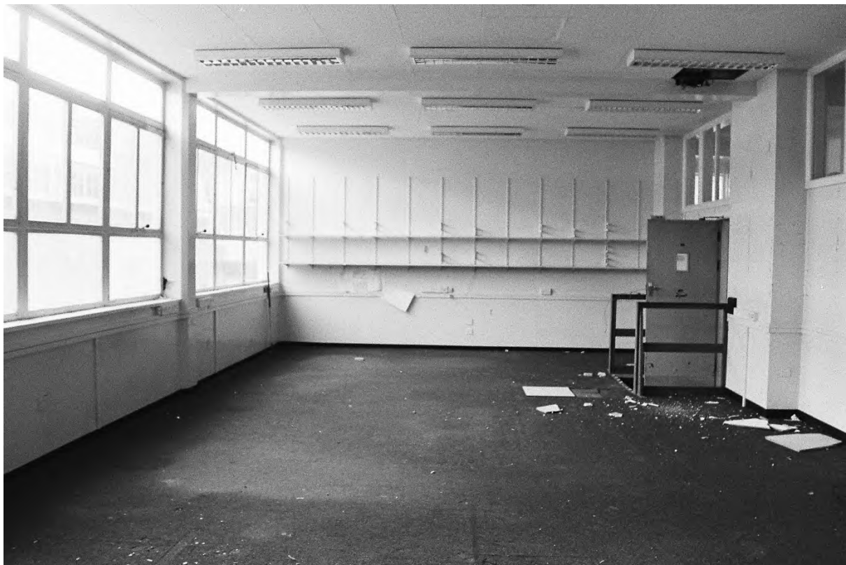
Plate 128. Block H: Interior Ground Floor Room H4 (Swinden2_28). Facing East.
