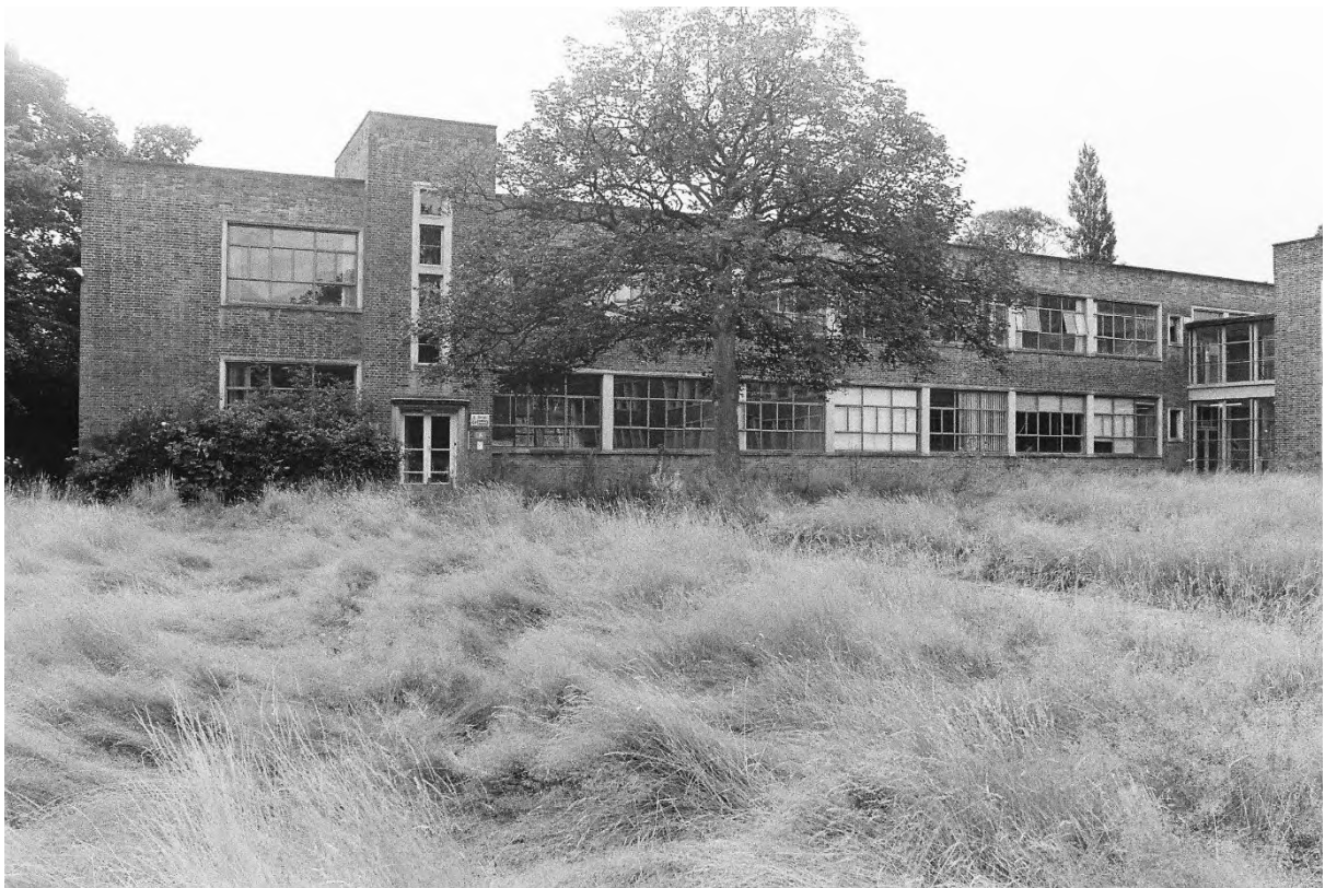
Plate 8. Block A: Exterior North Elevation (Swidon10_15). Facing South.
