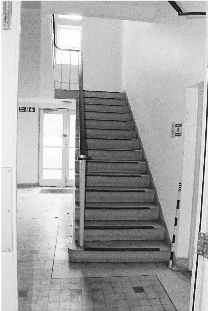
Plate 103. Block A: Interior Ground Floor Stairs (Swinden2_12) Facing North.
