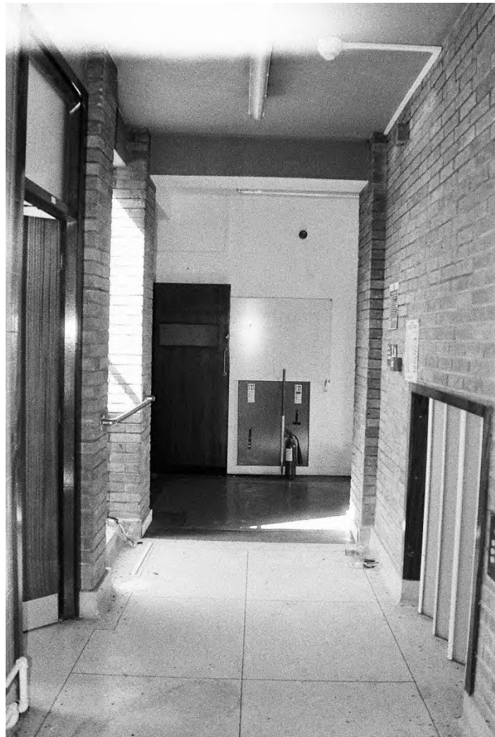
Plate 250. Block Q: Interior Second Floor Room Q18 (Swinden9_15). Facing North.
