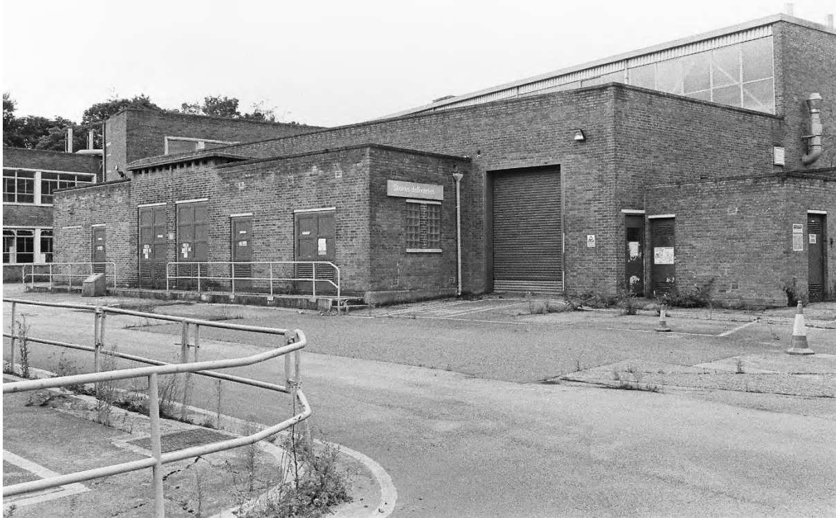
Plate 61. Blocks E & L: Exterior North & East Elevations (Swinden10_18). Facing South-west.
