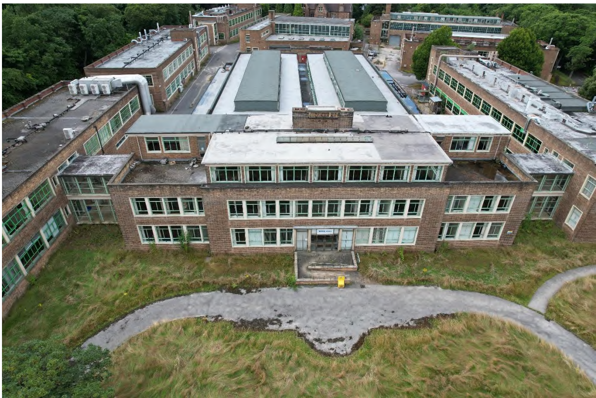
Plate 2. Block C from Drone (DJI_0078). Facing West.
