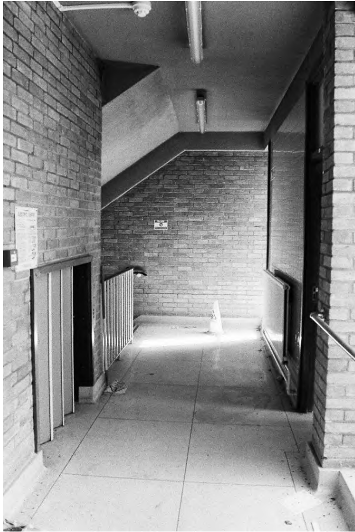
Plate 251. Block Q: Interior Second Floor Room Q18 (Swinden9_06). Facing South.
