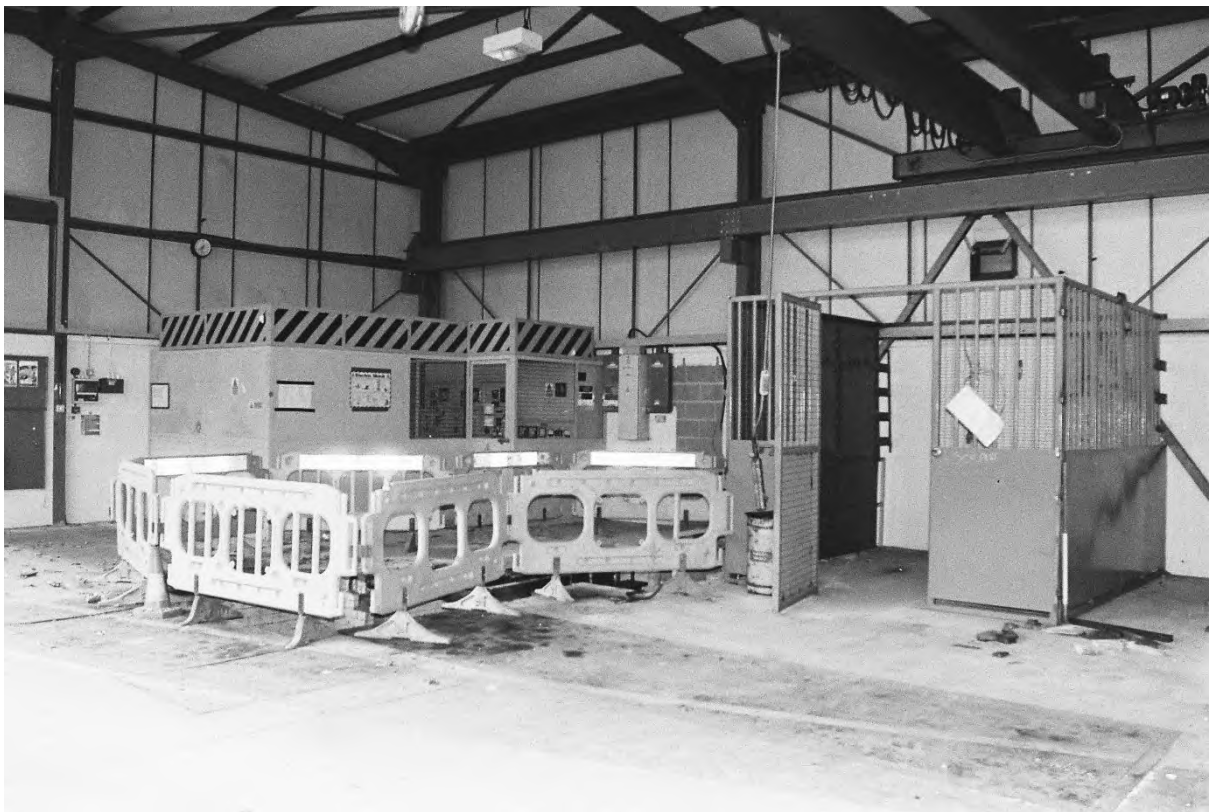
Plate 258. Block R: Interior (Swinden7_08). Facing South-west.
