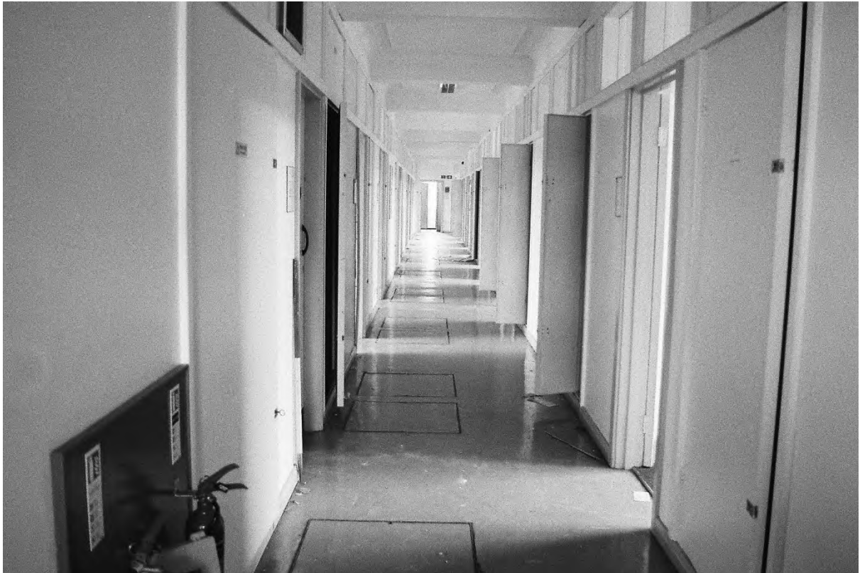
Plate 197. Block J: Interior First Floor Corridor J36 (Swinden7_12). Facing South.
