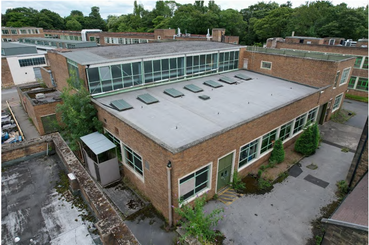
Plate 59. Block L from Drone (DJI_0162). Facing South-east.
