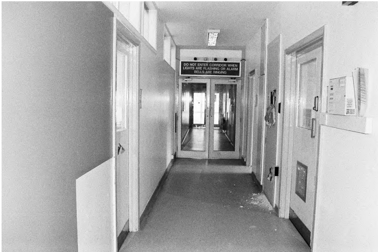
Plate 144. Block B: Interior Ground Floor Corridor (Swinden4_31). Facing West.
