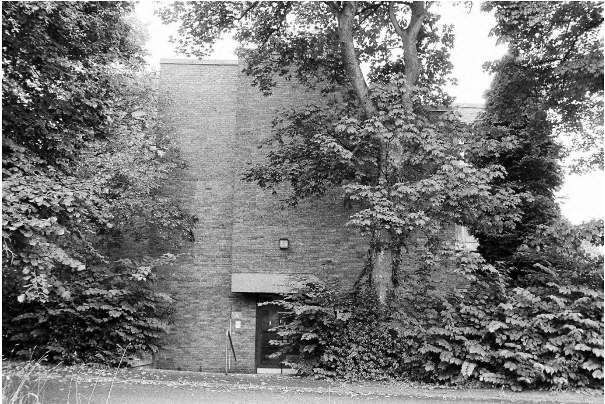
Plate 71. Block Q: Exterior South Elevation (Swinden11_30). Facing North.
