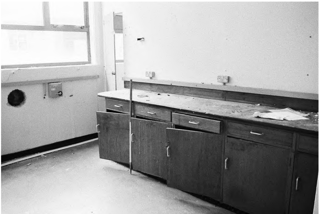
Plate 148. Block B: Interior Ground Floor Room B68 (Swinden4_20). Facing South.
