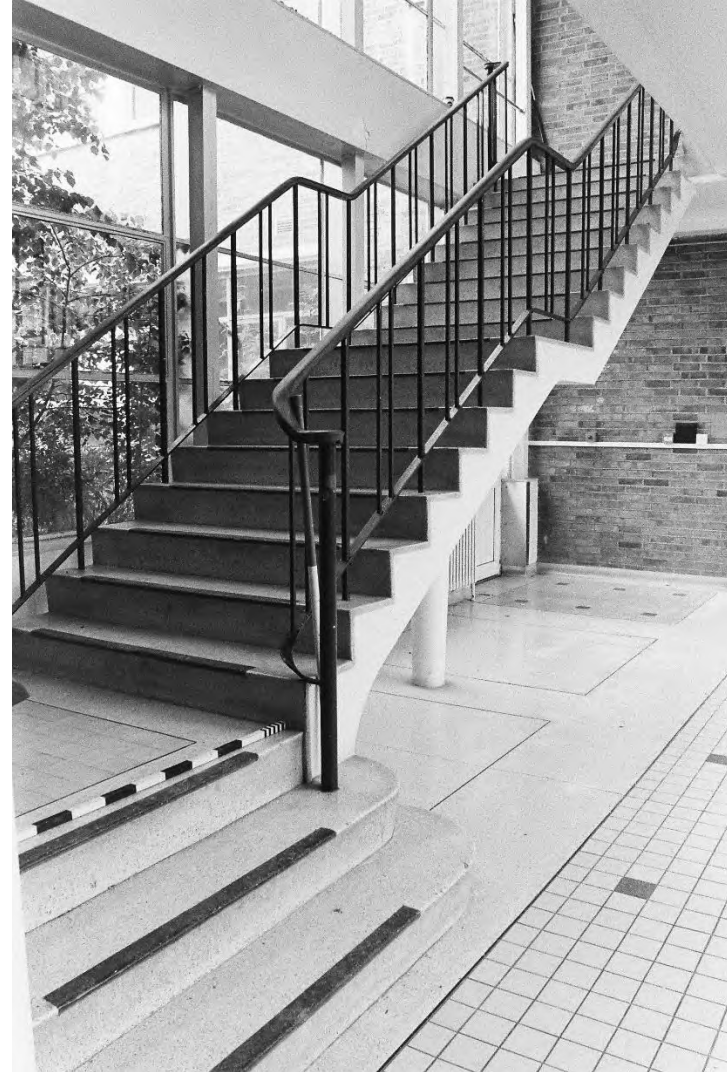
Plate 88. Ground Floor Stairs between Block C & B (Swinden11_23). Facing North-west.
