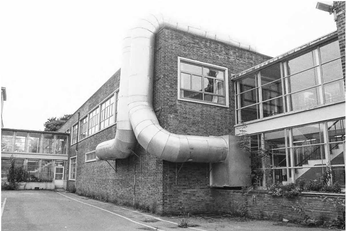
Plate 9. Block A: Exterior North Elevation (Swinden9_31). Facing East.
