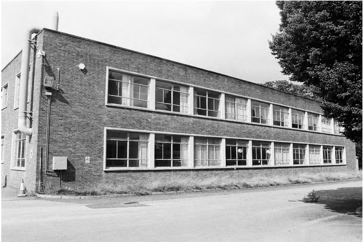
Plate 49. Block J: Exterior East & South Elevations (Swinden11_04). Facing North-west.
