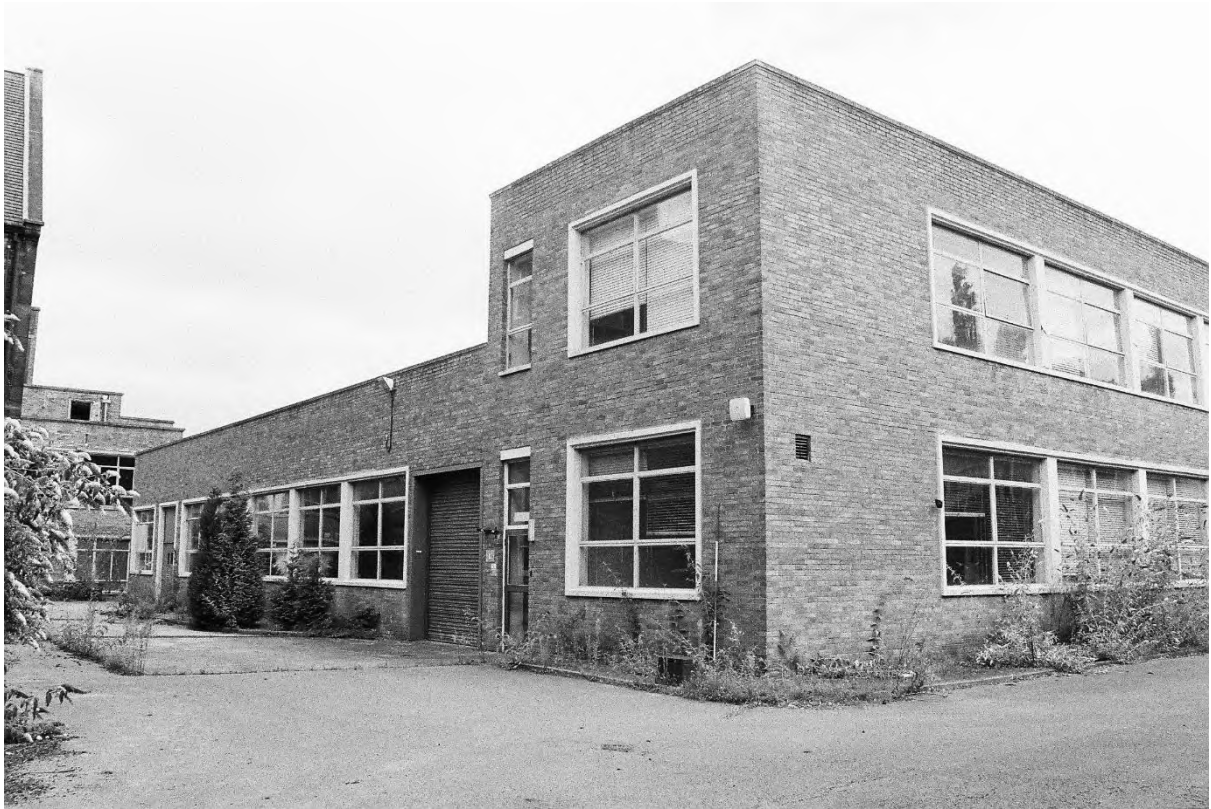
Plate 63. Block L: Exterior South & West Elevations (Swinden11_20). Facing North-east.
