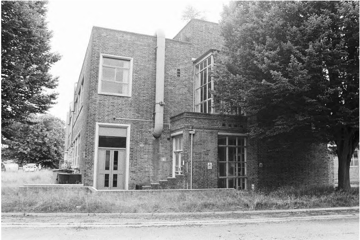
Plate 25. Block B: Exterior West Elevation (Swinden 10_06). Facing East.
