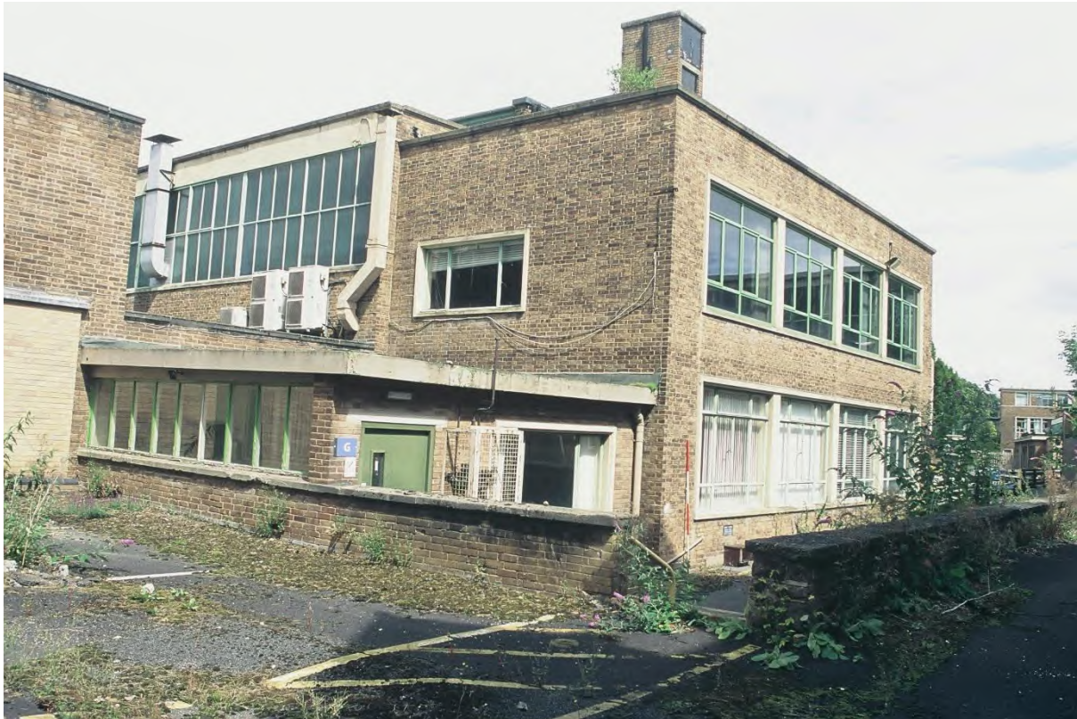
Plate 37. Block F: Exterior South & West Elevations (Swinden13_18). Facing North.
