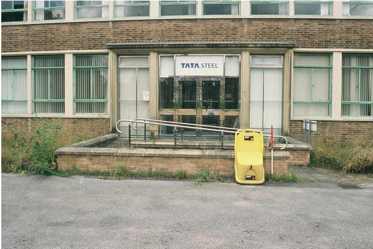
Plate 81. Block C: Entrance (Swinden5_36). Facing West.
