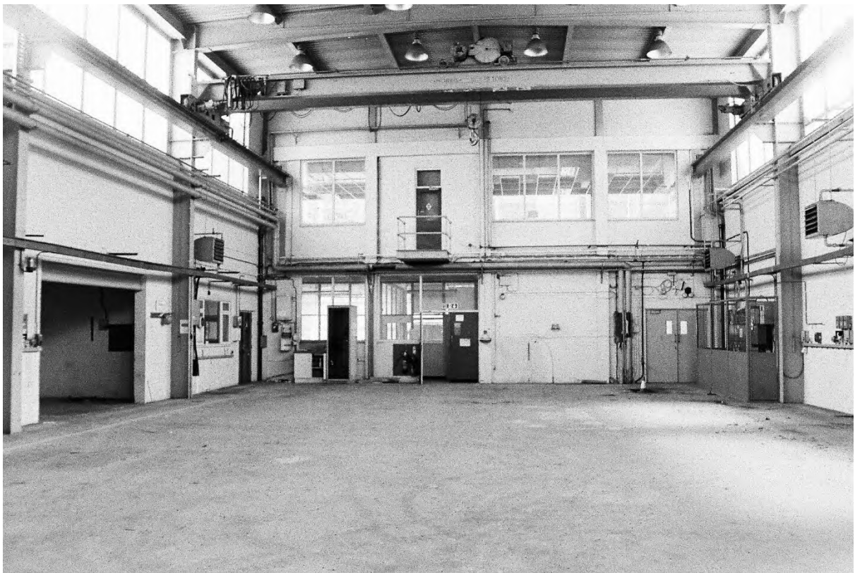
Plate 234. Block L: Interior Ground Floor Room L17 (Swinden8_26). Facing South.
