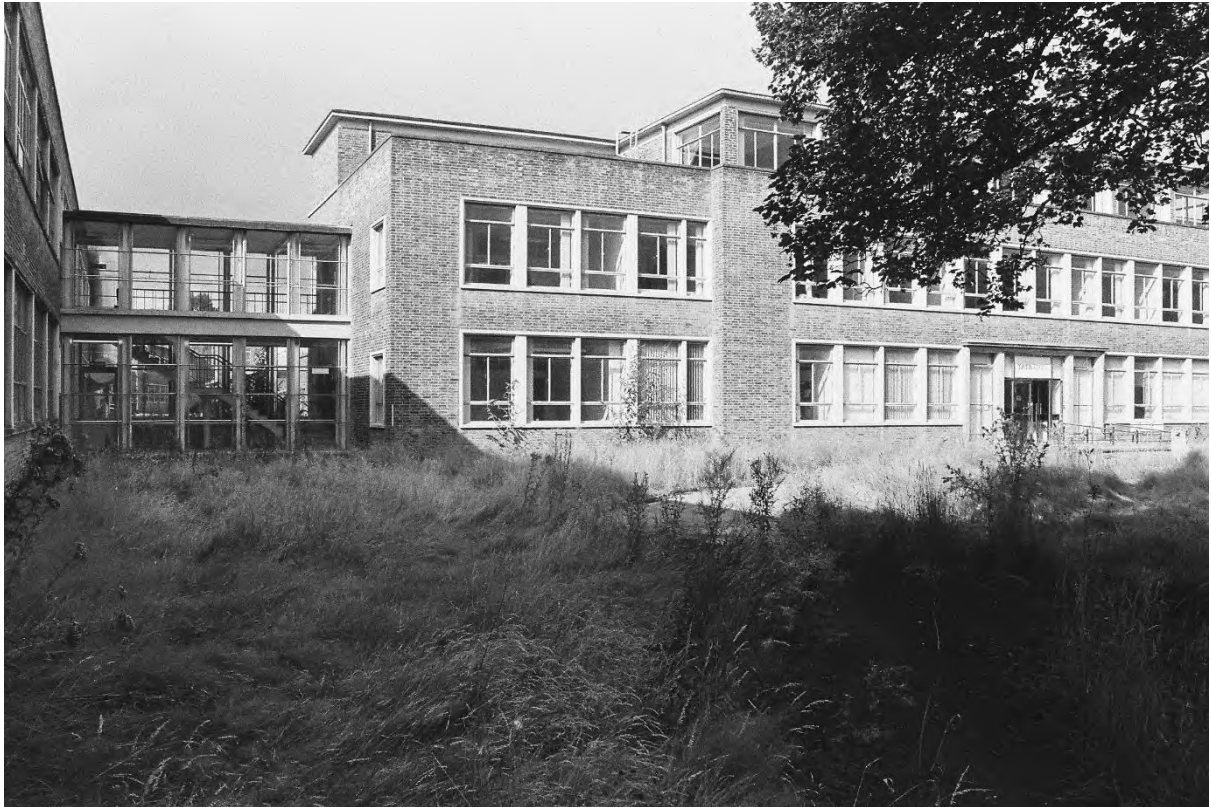
Plate 5. Block C: Exterior East Elevation (Swinden10_17). Facing West.
