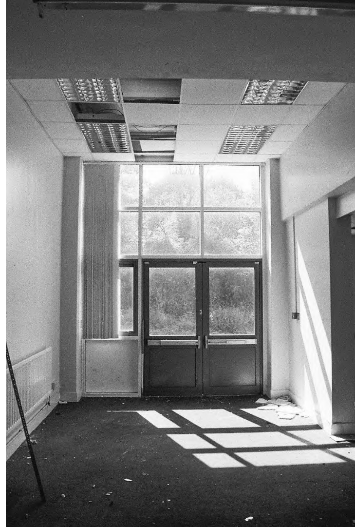
Plate 246. Block Q: Interior Ground Floor Room Q2 (Swinden9_14). Facing West.
