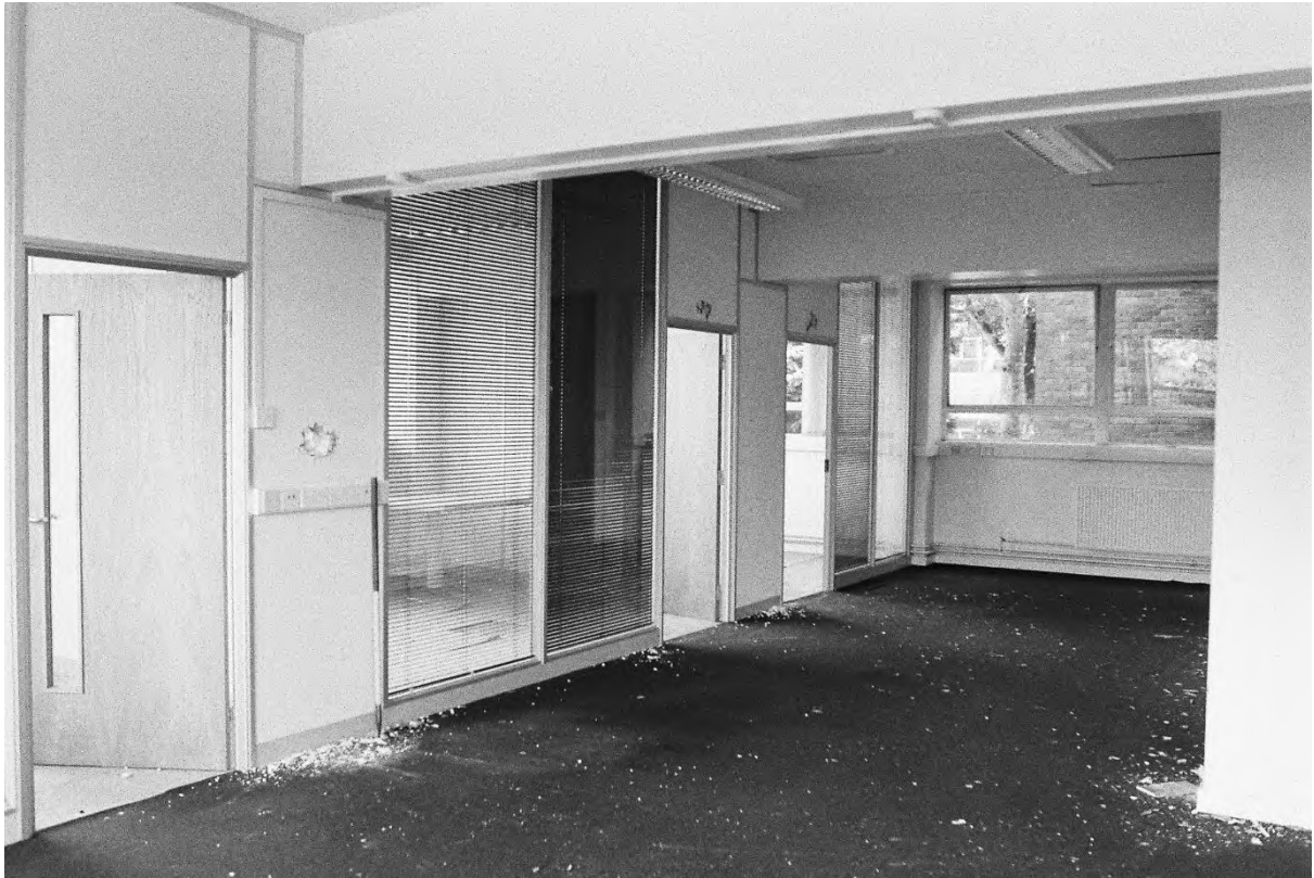
Plate 249. Block Q: Interior First Floor Room Q11/Q15 (Swinden9_09). Facing South.
