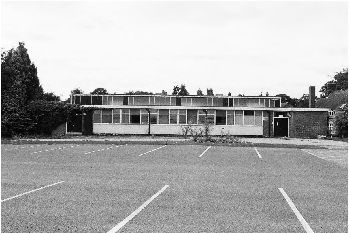
Plate 79. Canteen: Exterior East Elevation (Swinden11_33). Facing West.
