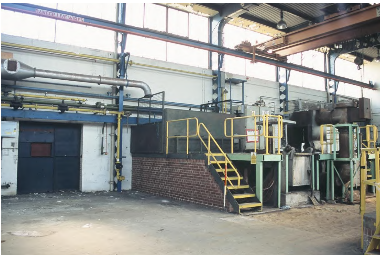
Plate 174. Block F: Interior Ground Floor Room F8 (Swinden12_04). Facing South-east.
