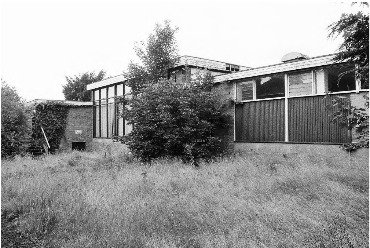
Plate 80. Canteen: Exterior South Elevation (Swinden11_34). Facing North-west.
