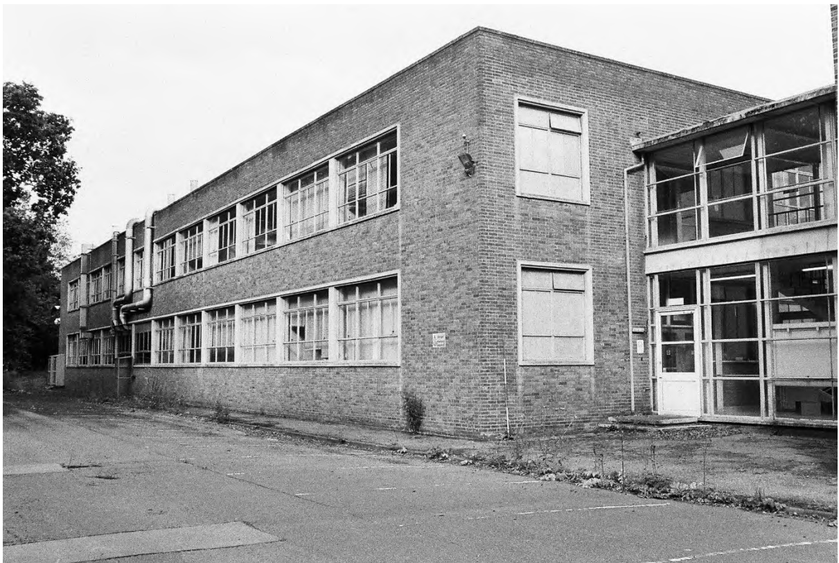
Plate 14. Block H: Exterior East & South Elevations (Swinden9_23). Facing South-west.
