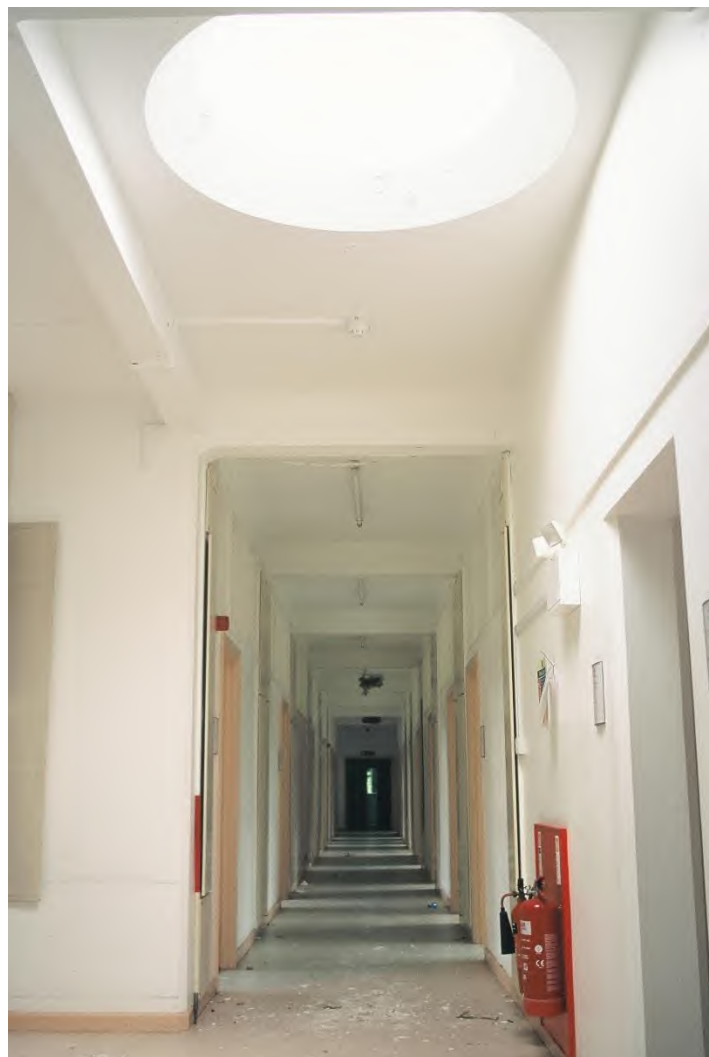
Plate 116. Block A: Interior First Floor Corridor & Skylight (Swinden5_02). Facing East.
