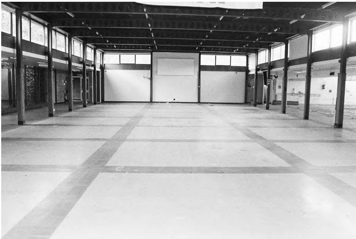
Plate 260. Canteen: Interior (Swinden6_07). Facing North.
