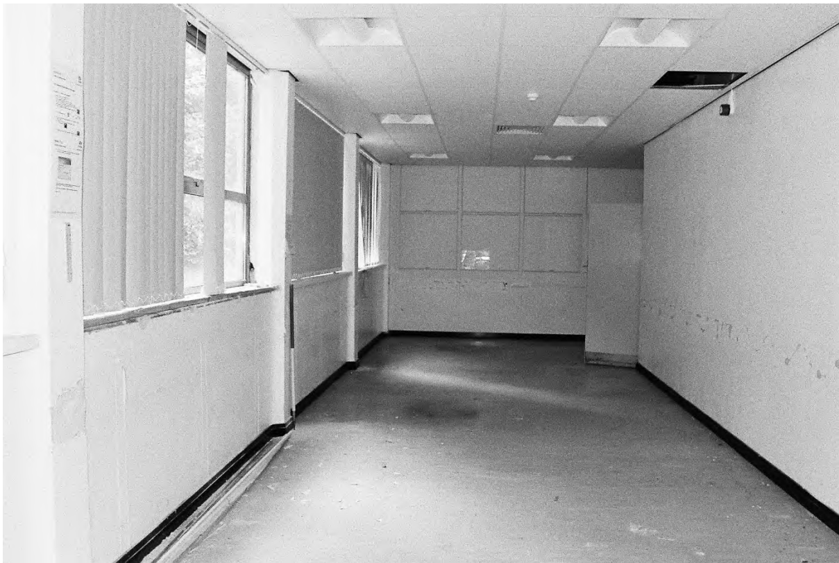
Plate 208. Block K: Interior Ground Floor Room K9 (Swinden8_06). Facing West.
