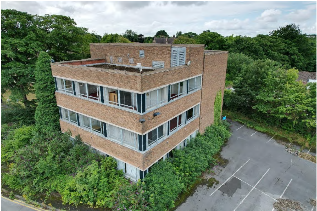
Plate 66. Block Q from the Drone (DJI_0051). Facing South-east.
