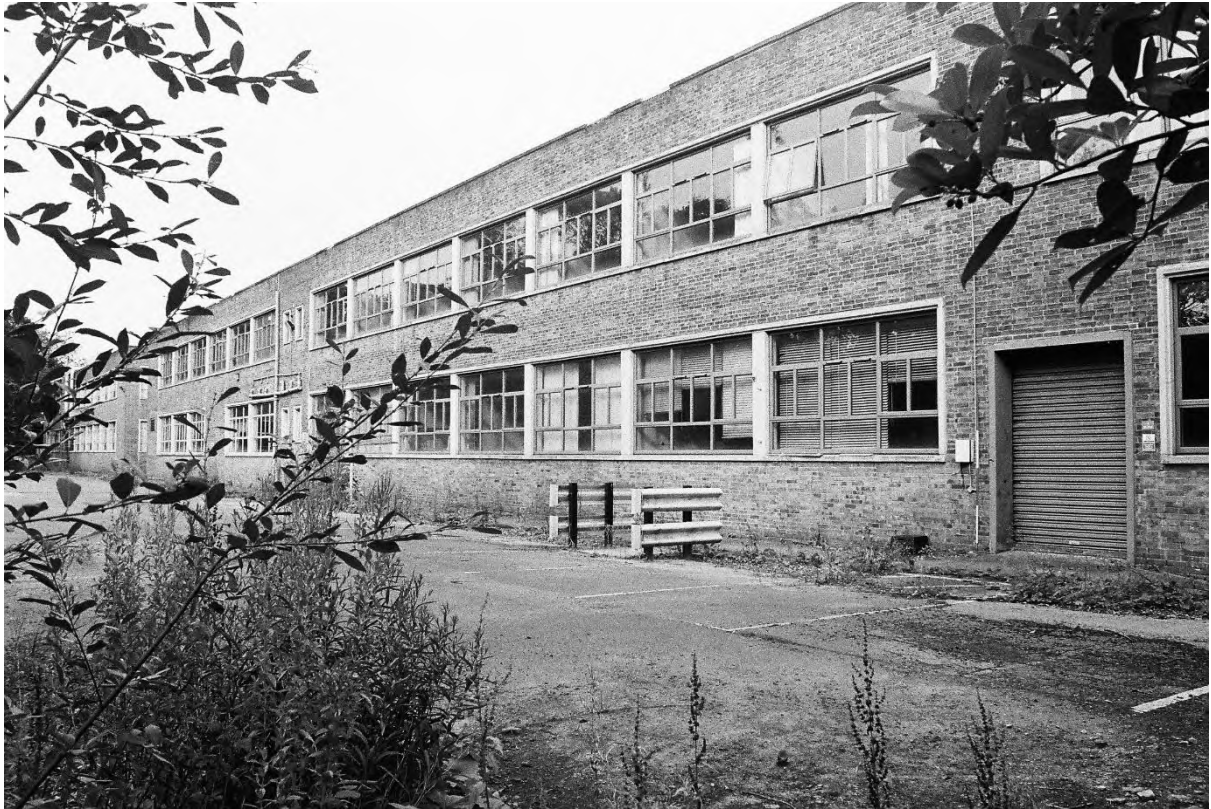
Plate 11. Block A: Exterior South Elevation (Swinden9_18). Facing North-west.
