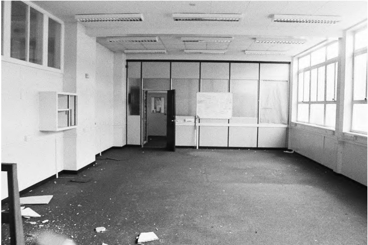
Plate 129. Block H: Interior Ground Floor Room H4 (Swinden2_29). Facing West.
