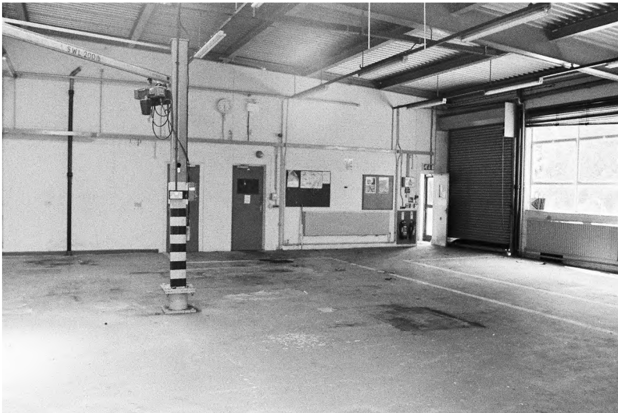
Plate 232. Block L: Interior Ground Floor Room L15 (Swinden8_23). Facing South.
