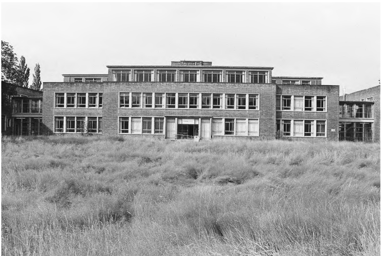
Plate 4. Block C: Exterior East Elevation (Swinden10_14). Facing West.
