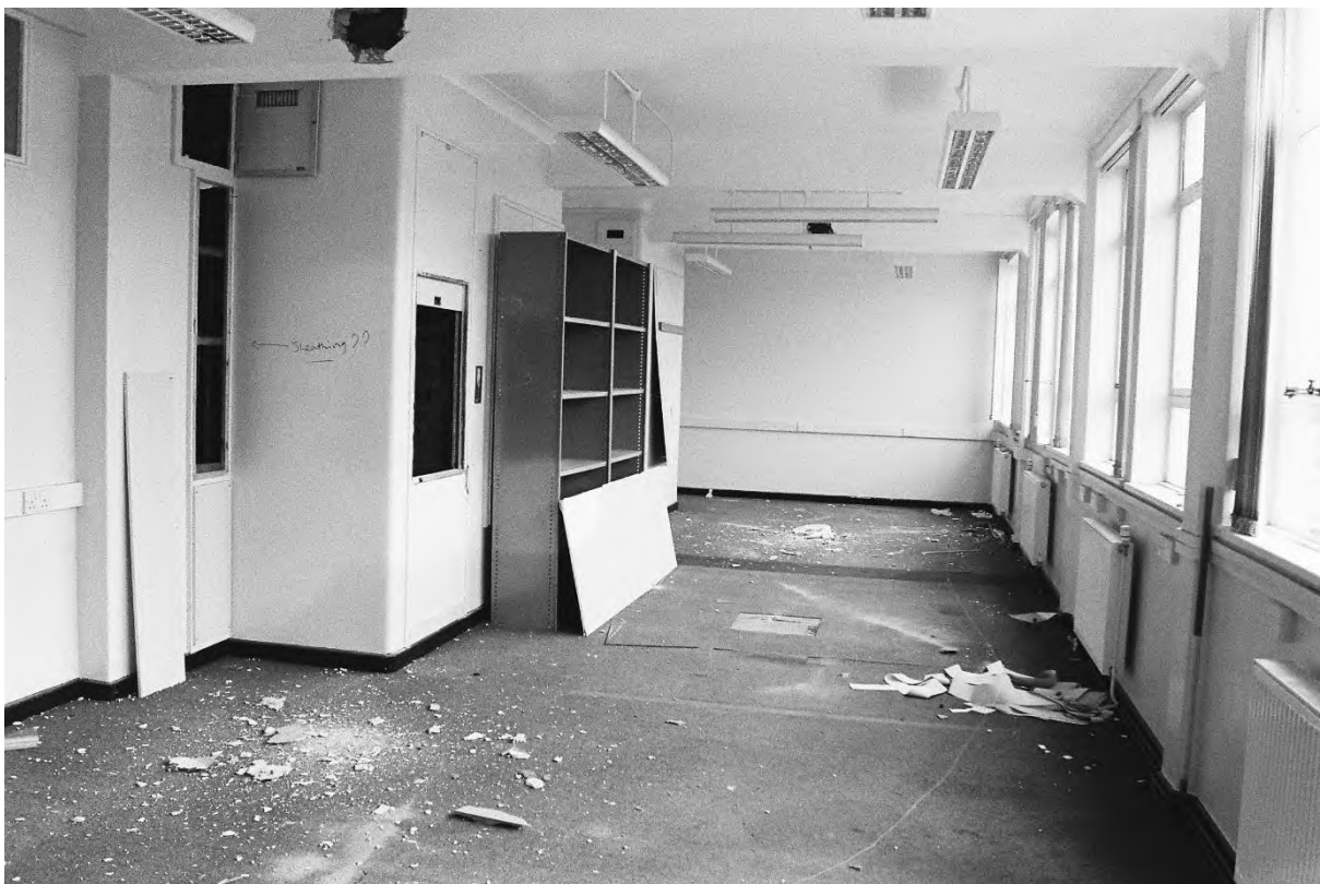
Plate 92. Block C: Interior First Floor Room C135/C137 (Swinden11_27). Facing South.
