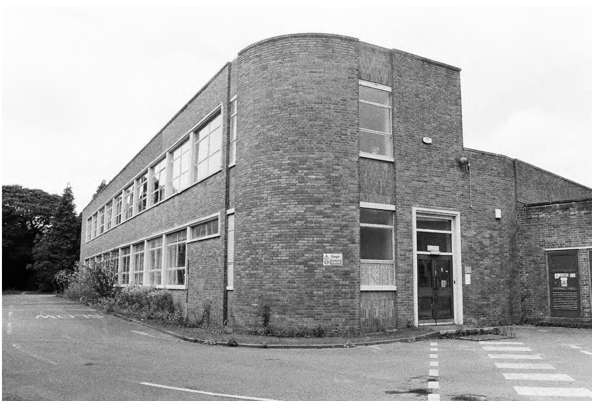
Plate 62. Block L: Exterior East & South Elevations (Swinden11_22). Facing West.
