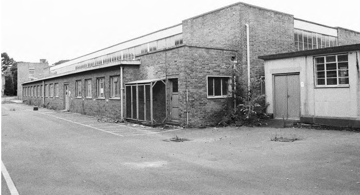
Plate 32. Block D: Exterior South Elevation (Swinden9_35). Facing South-west.
