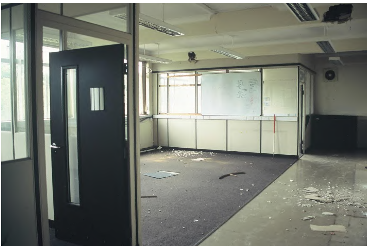
Plate 98. Block C: Interior Ground Floor Room C150/150A/150D (Swinden15_18). Facing South-east.
