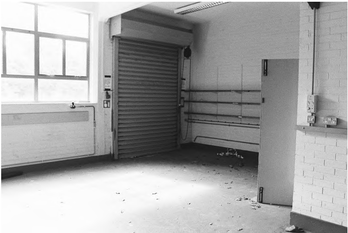
Plate 106. Block A: Interior Ground Floor Room A1 (Swinden2_09). Facing South-west.
