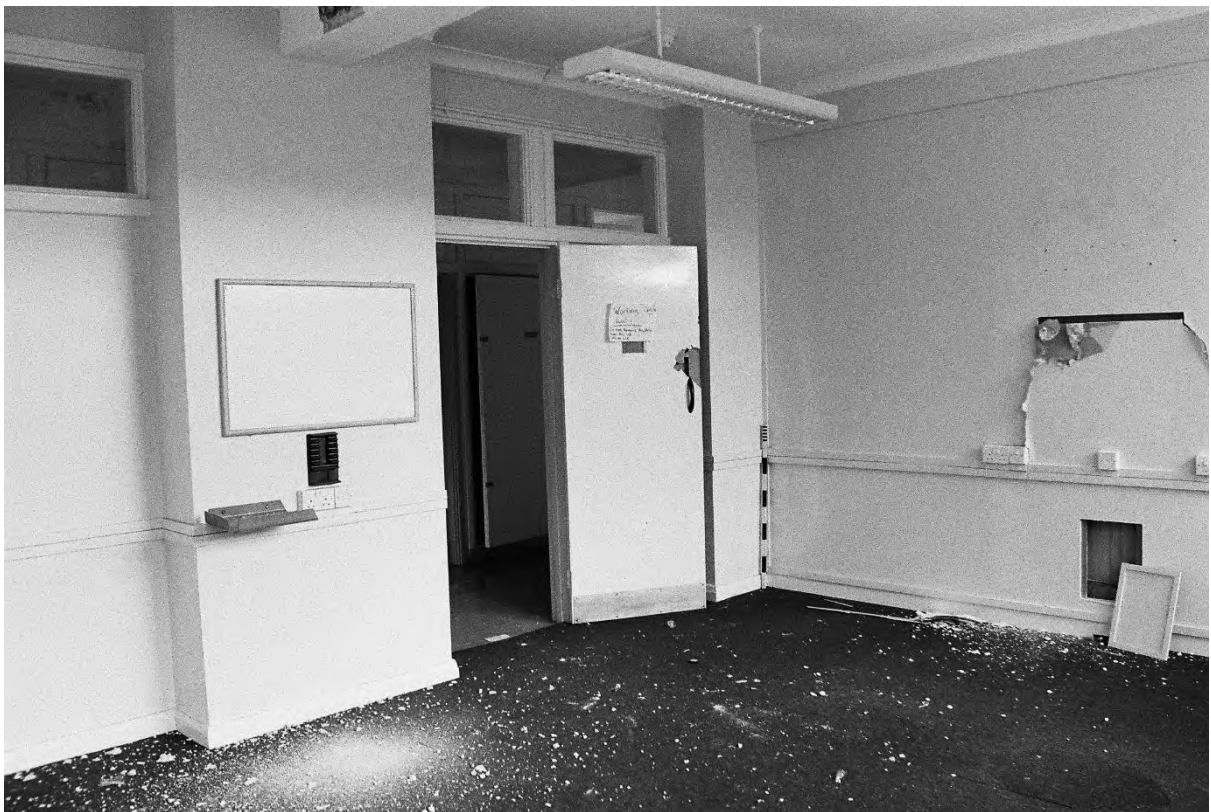
Plate 200. Block J: Interior First Floor Room J33/J33A (Swinden7_11). Facing South-east.
