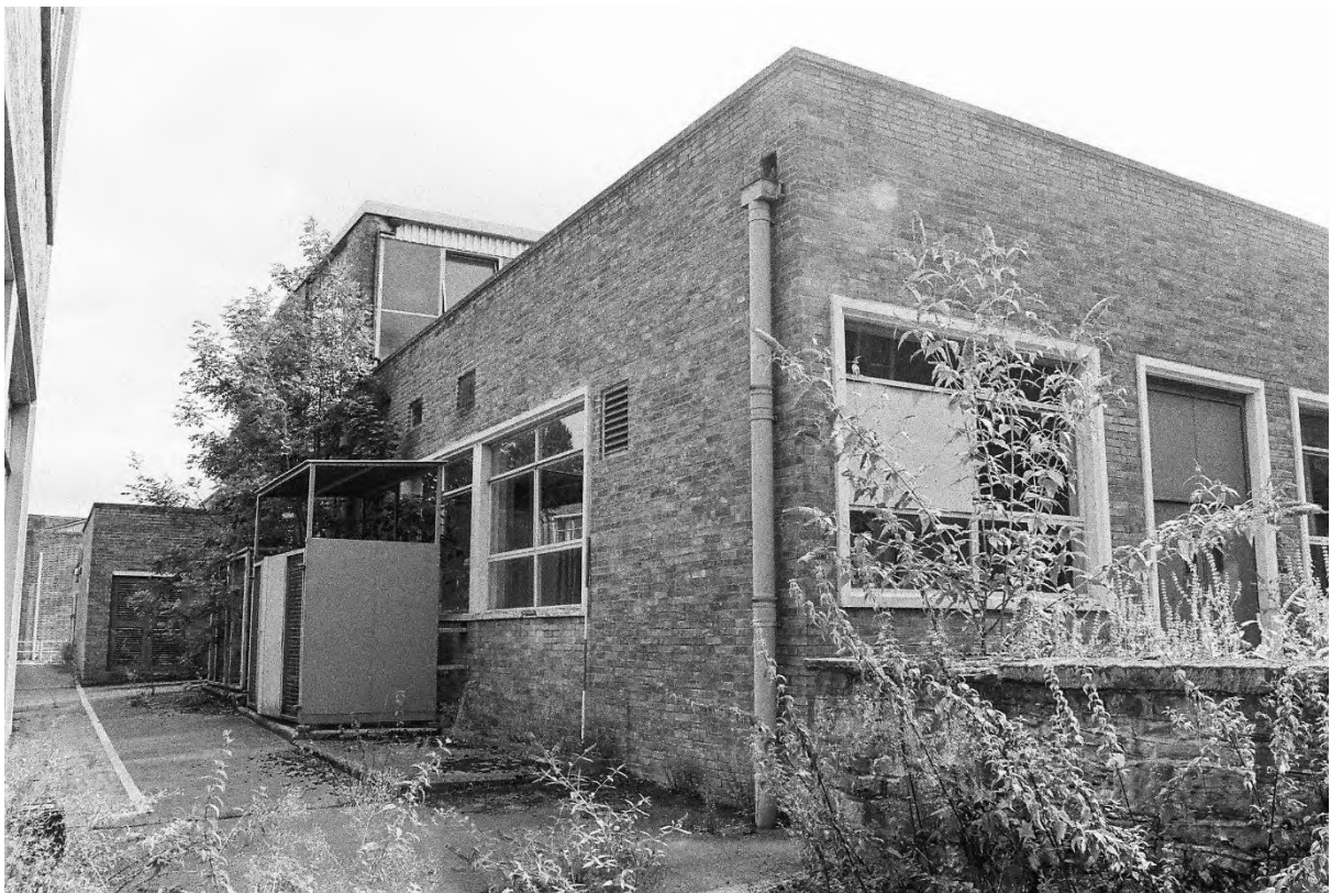
Plate 64. Block L: Exterior West & North Elevations (Swinden11_24). Facing East.
