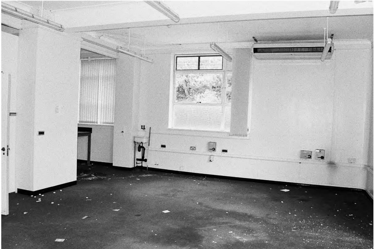
Plate 225. Block K: Interior First Floor Room K42/K44 (Swinden8_09). Facing South-west.
