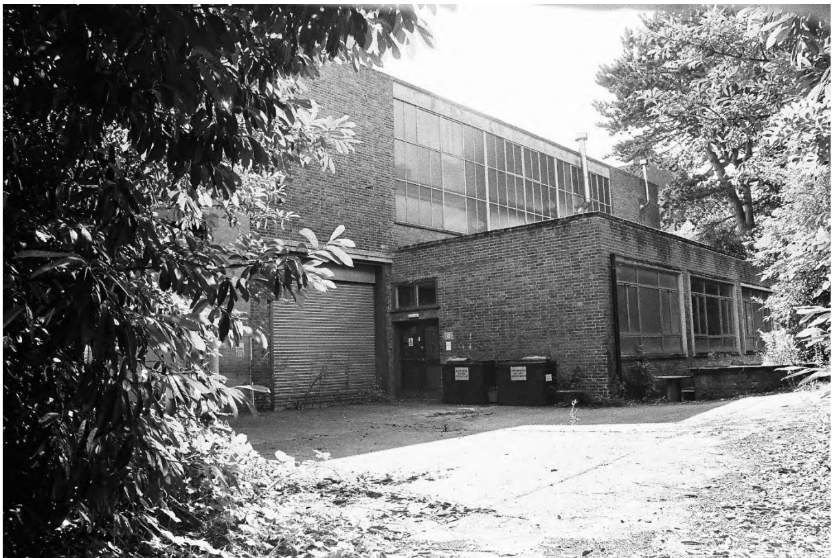
Plate 44. Block G: Exterior West Elevation (Swinden10_31). Facing South-east.
