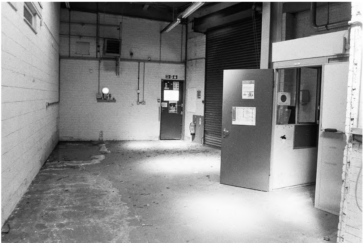
Plate 236. Block L: Interior Ground Floor Room L18A (Swinden8_29). Facing North.
