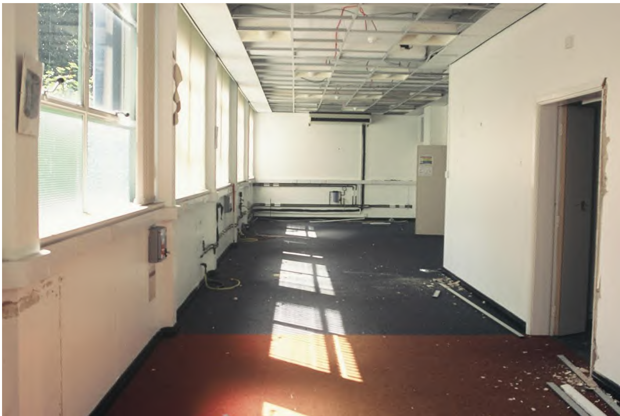
Plate 220. Block K: Interior First Floor Room K29/K37 (Swinden12_25). Facing West.
