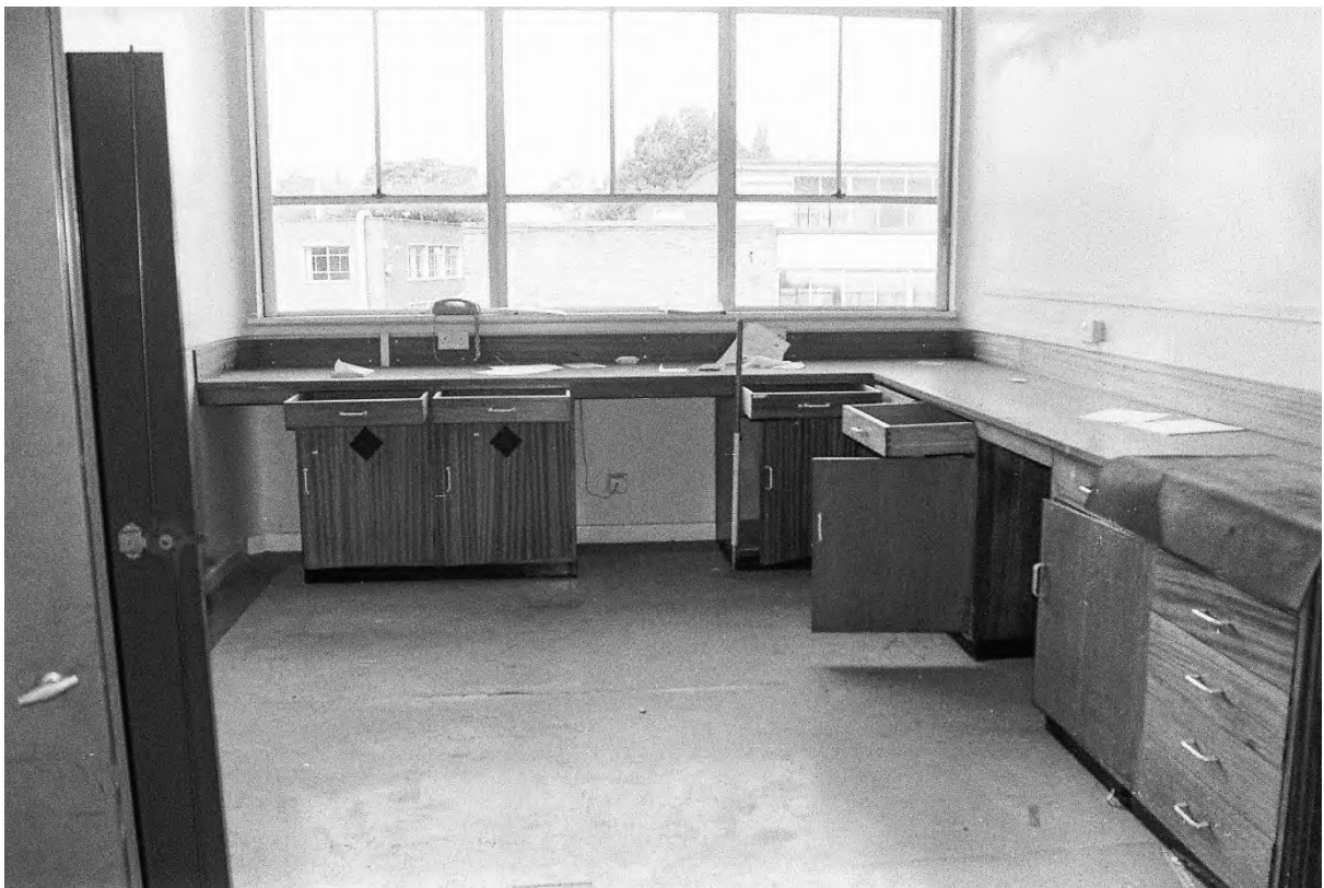
Plate 138. Block H: Interior First Floor Room H28 (Swinden3_25). Facing North.
