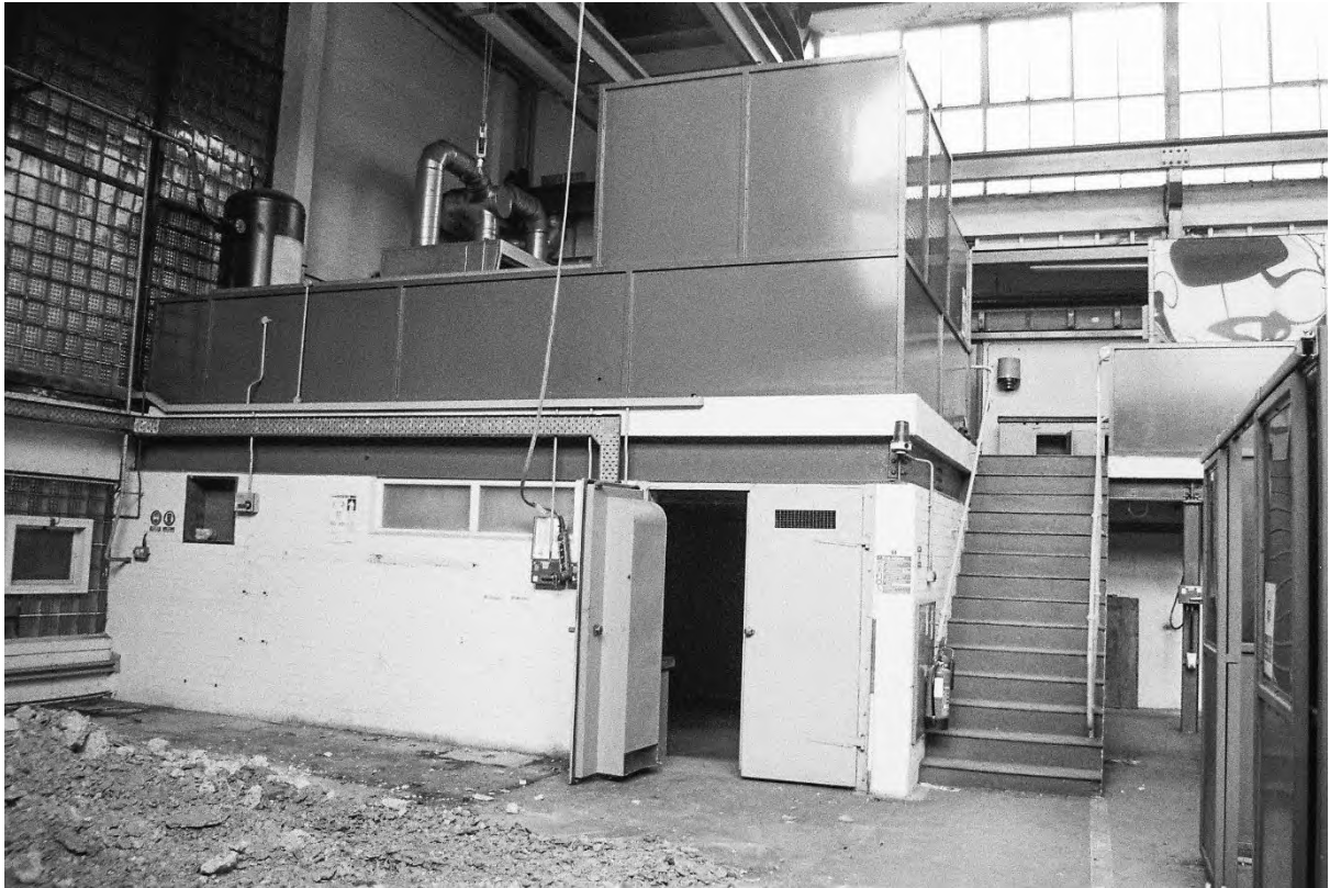
Plate 183. Block G: Interior Mezzanine & Room G2 (Swinden6_31). Facing North-east.
