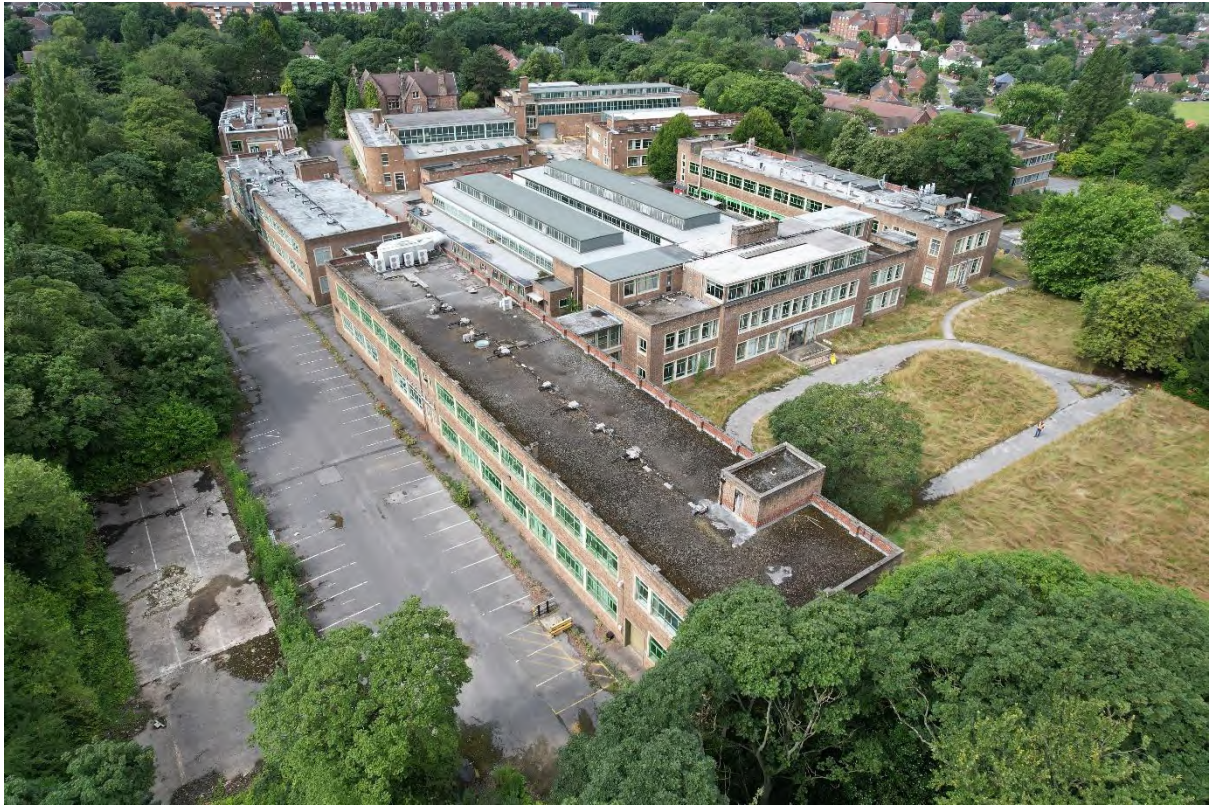
Plate 1. Swinden Technology Centre from Drone (DJI_0090). Facing North-west.
