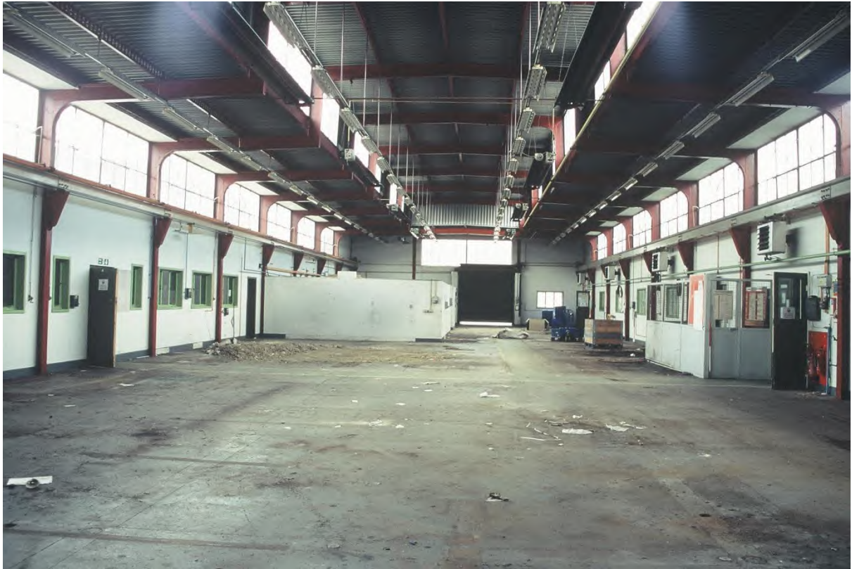
Plate 167. Block D: Interior Room D176/D179 (Swinden5_29). Facing West.
