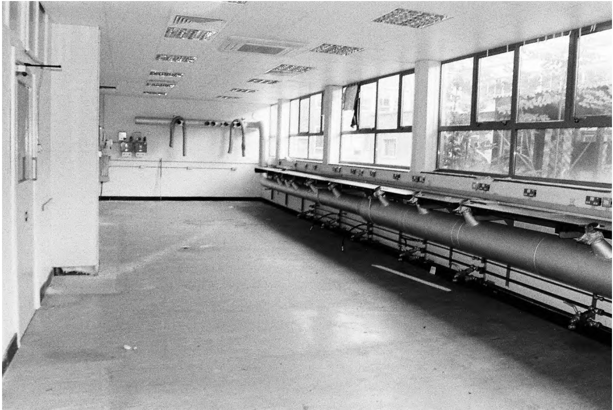
Plate 151. Block B: Interior Ground Floor Room B78/B79 (Swinden4_26). Facing West.
