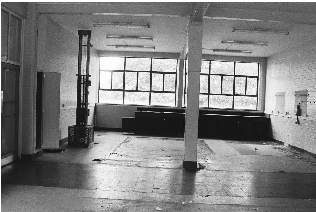
Plate 108. Block A: Interior Ground Floor Room A2 (Swinden2_05). Facing North.
