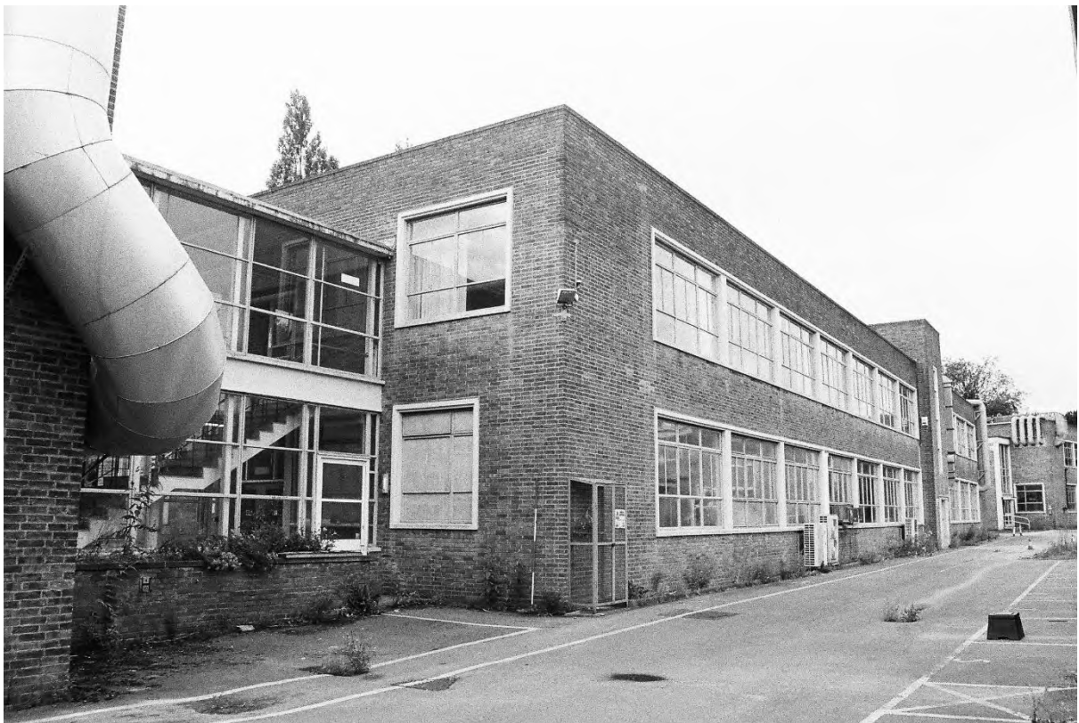
Plate 18. Block H: Exterior North Elevation (Swinden9_29). Facing South-west.
