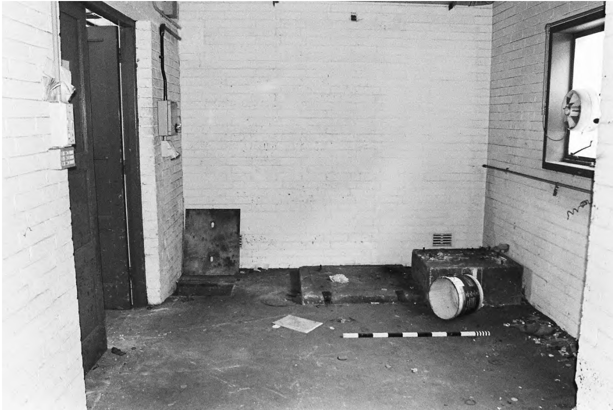
Plate 165. Block D: Interior Room D216 (Swinden1_16). Facing West.
