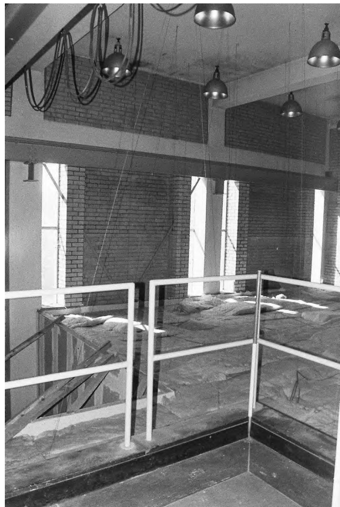
Plate 254. Block Q: Interior Second Floor Room Q11 (Swinden9_02). Facing North-west.
