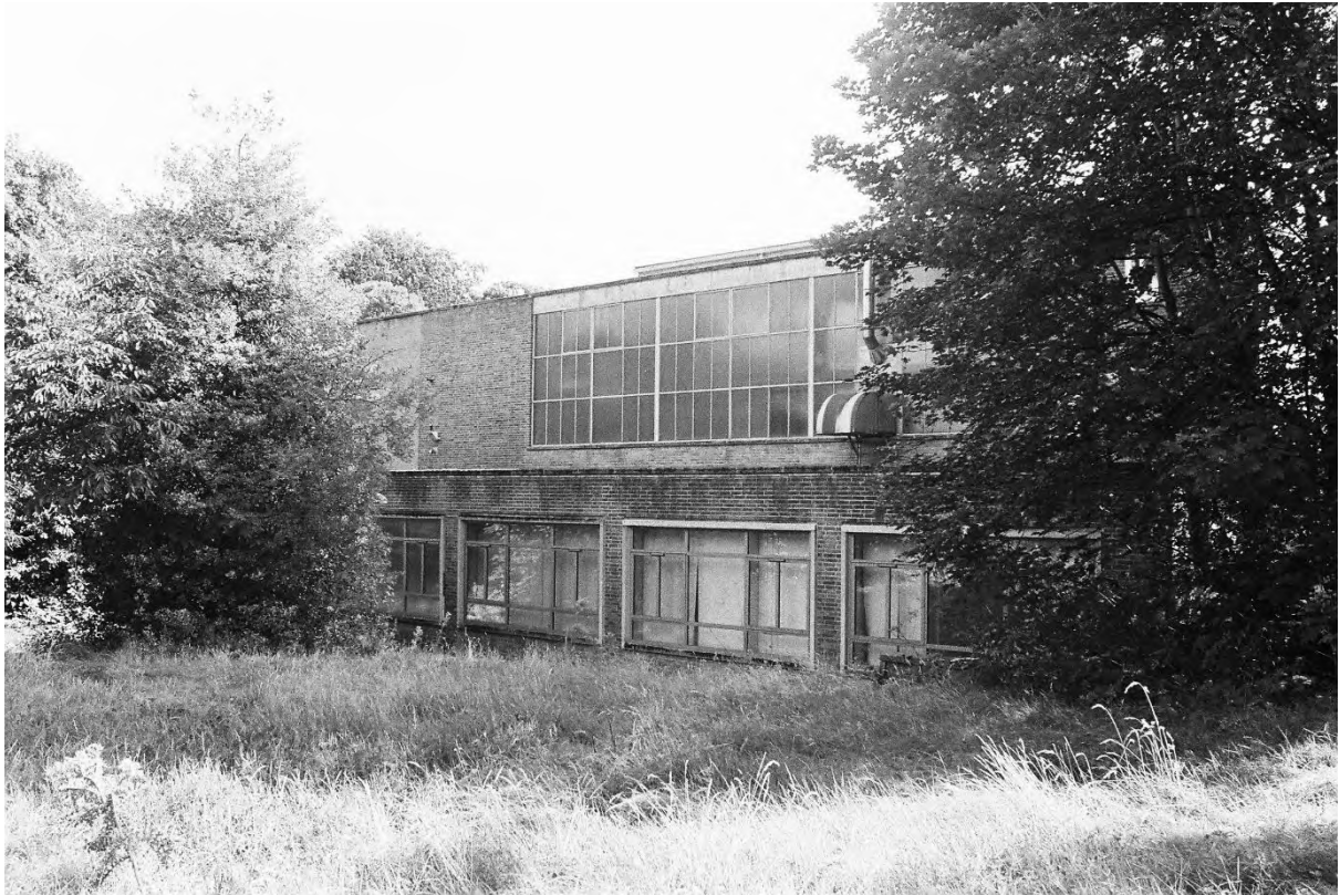
Plate 43. Block G: Exterior West Elevation (Swinden10_30). Facing North-east.
