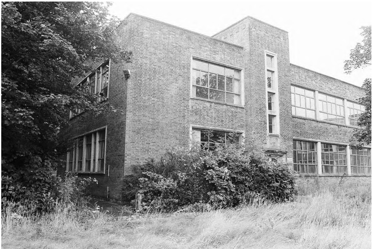
Plate 10. Block A: Exterior North and East Elevations (Swinden9_16). Facing South-west.
