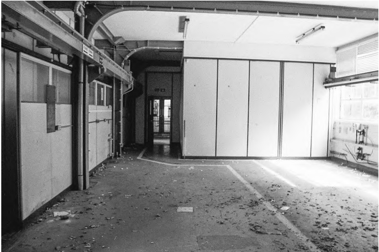
Plate 133. Block H: Interior Ground Floor Room H12 (Swinden3_07). Facing East.
