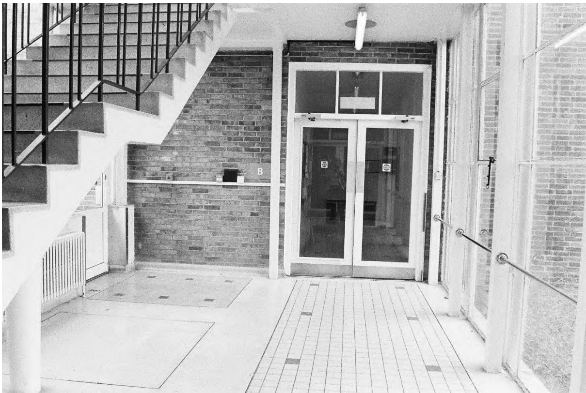
Plate 142. Block B Ground Floor Entrance from Block C (Swinden4_10). Facing North.
