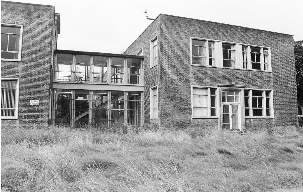
Plate 21. Block B: Exterior East Elevation (Swinden10.12). Facing West.
