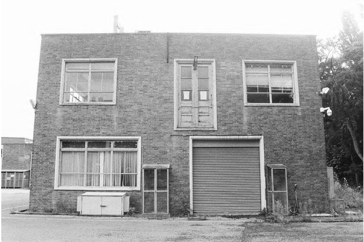
Plate 16. Block H: Exterior West Elevation (Swinden9_25). Facing East.
