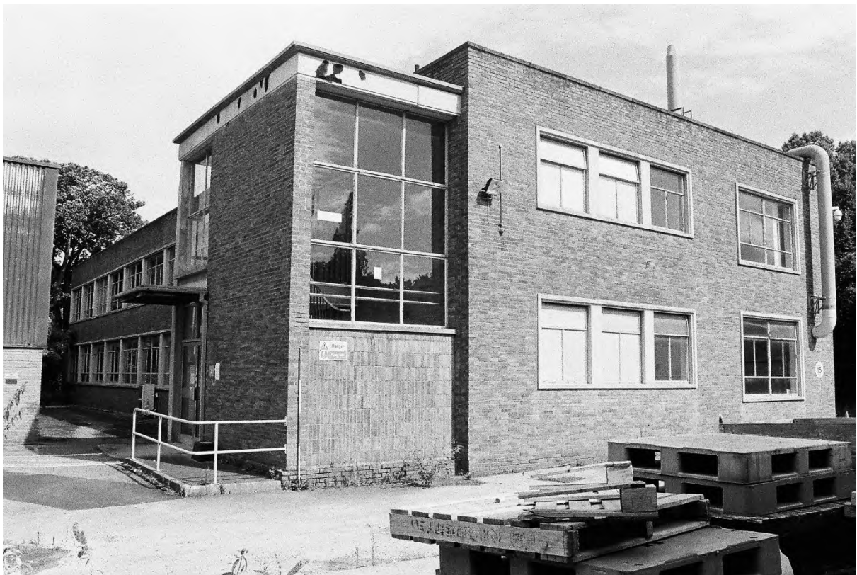
Plate 50. Block J: Exterior South & West Elevations (Swinden11_06). Facing North.
