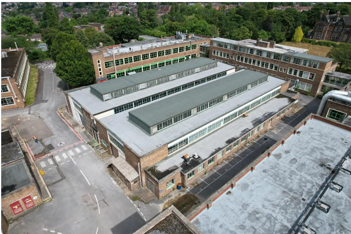
Plate 28. Block D from Drone (DJI_0134). Facing North-east.
