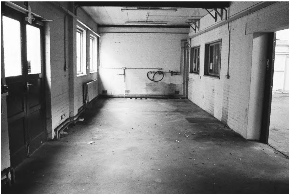
Plate 166. Block D: Interior Room D211 (Swinden1_18). Facing East.
