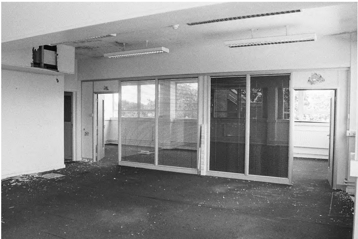
Plate 252. Block Q: Interior Second Floor Room Q19/Q19A (Swinden9_04). Facing North.
