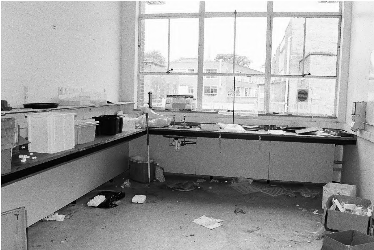
Plate 131. Block H: Interior Ground Floor Room H10 (Swinden2_34). Facing North.
