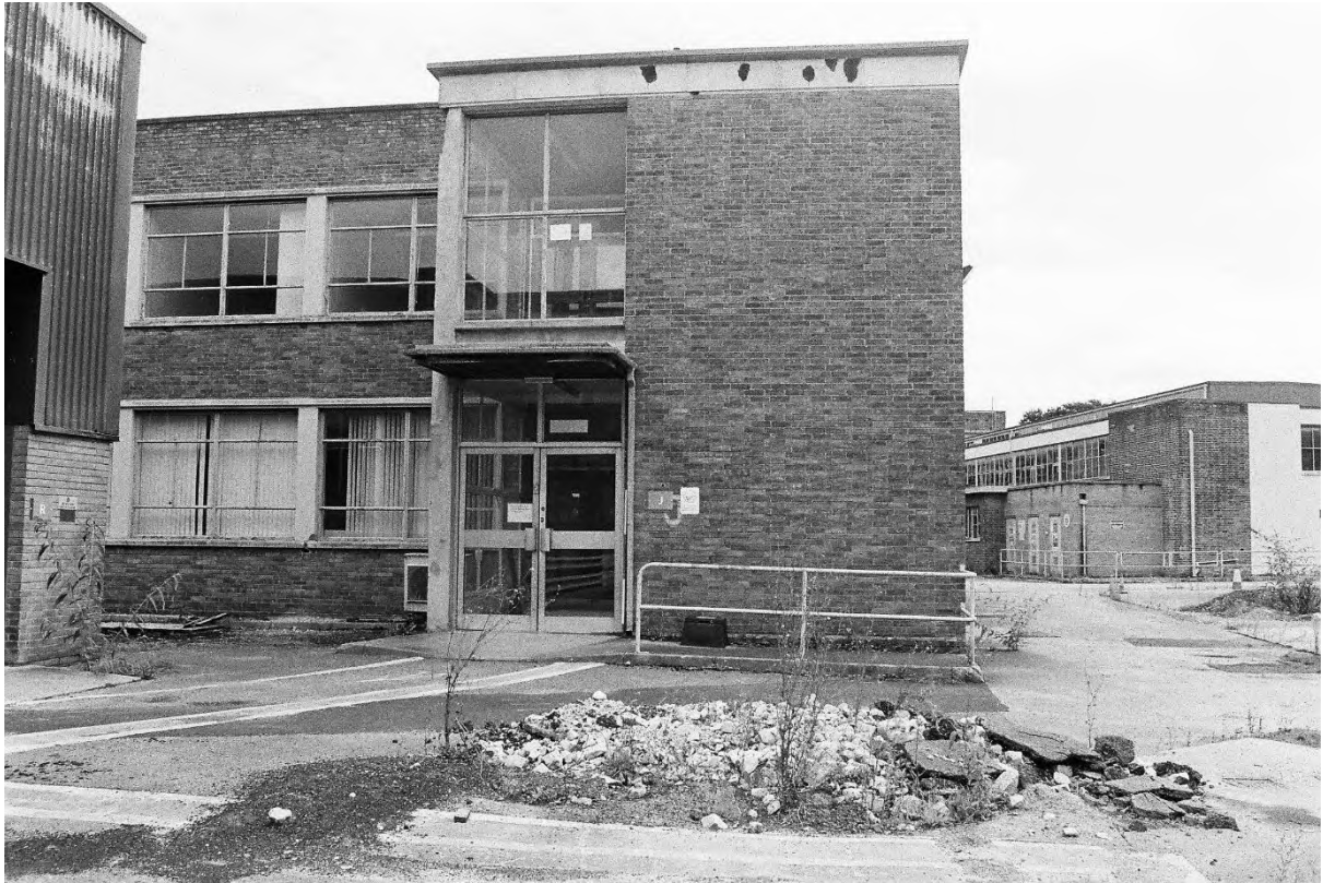
Plate 51. Block J: Exterior West Elevation (Swinden11_07). Facing East.
