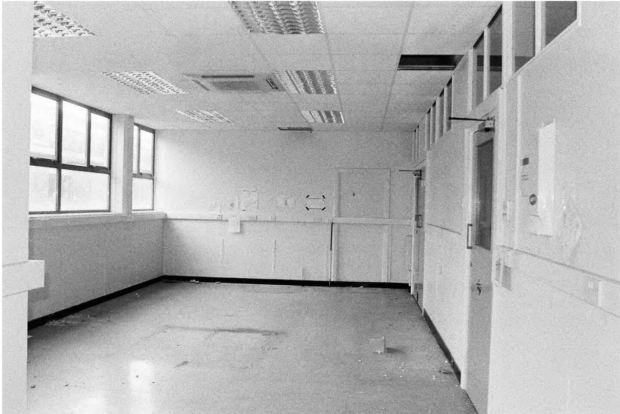
Plate 149. Block B: Interior Ground Floor Room B68A (Swinden4_23). Facing West.
