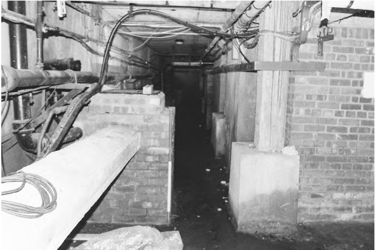
Plate 201. Block K: Interior Basement Duct (Swinden7_26). Facing West.
