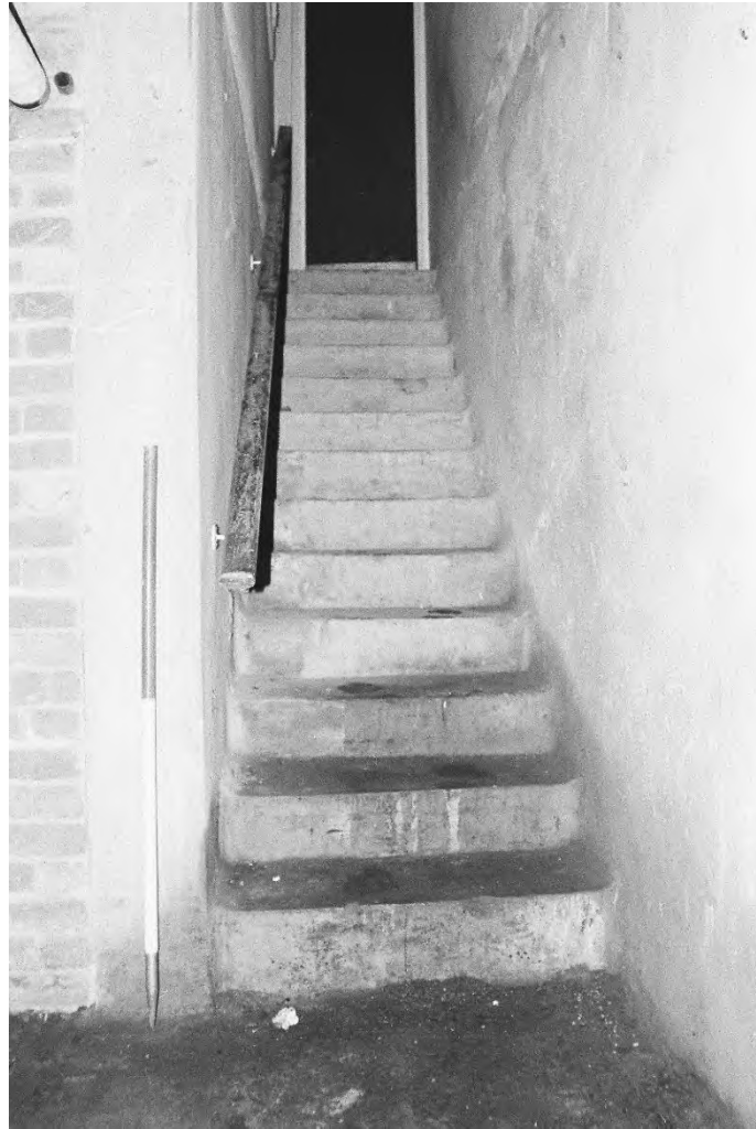
Plate 203. Block K: Interior Basement Stairs (Swinden7_28). Facing North.
