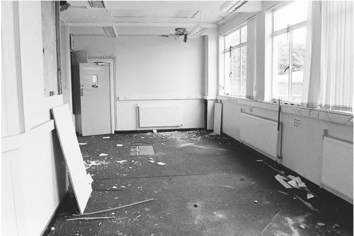
Plate 99. Block C: Interior Second Floor Room C156 (Swinden11_35). Facing South.
