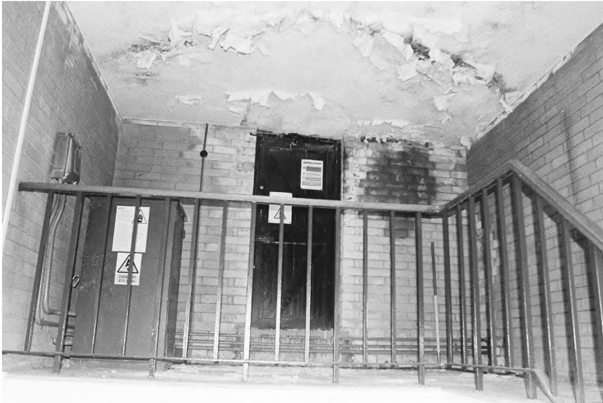
Plate 141. Block H: Interior Roof Access (Swinden3_28). Facing South.
