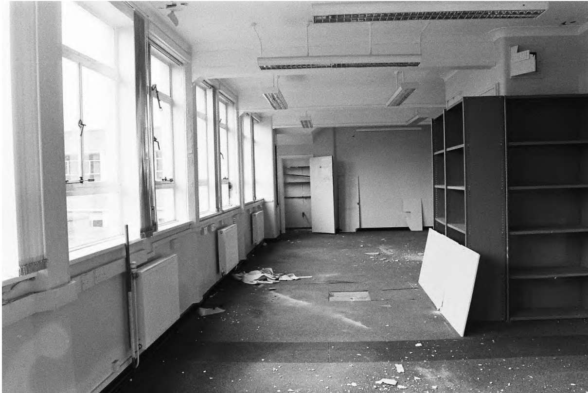
Plate 93. Block C: Interior First Floor Room C135/C137 (Swinden11_28). Facing North.
