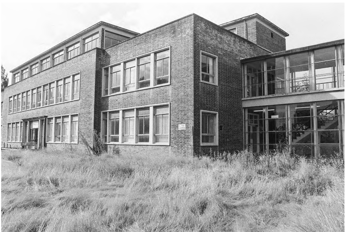
Plate 6. Block C: Exterior East Elevation (Swinden10_13). Facing South-west.
