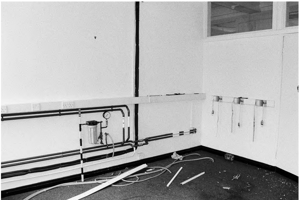
Plate 222. Block K: Interior First Floor Room K37(Swinden8_12). Facing North-west.
