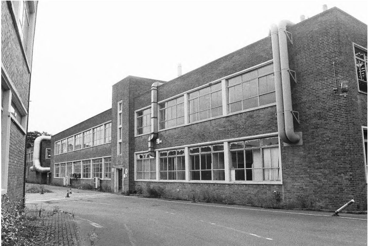
Plate 17. Block H: Exterior North Elevation (Swinden9_27). Facing North-east.
