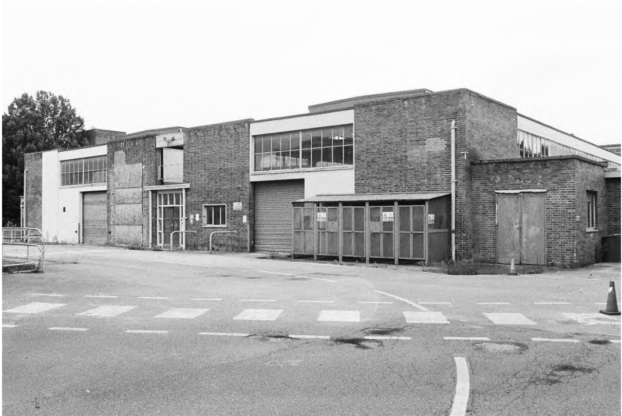
Plate 29. Block D: Exterior West Elevation (Swinden9_37). Facing North-east.
