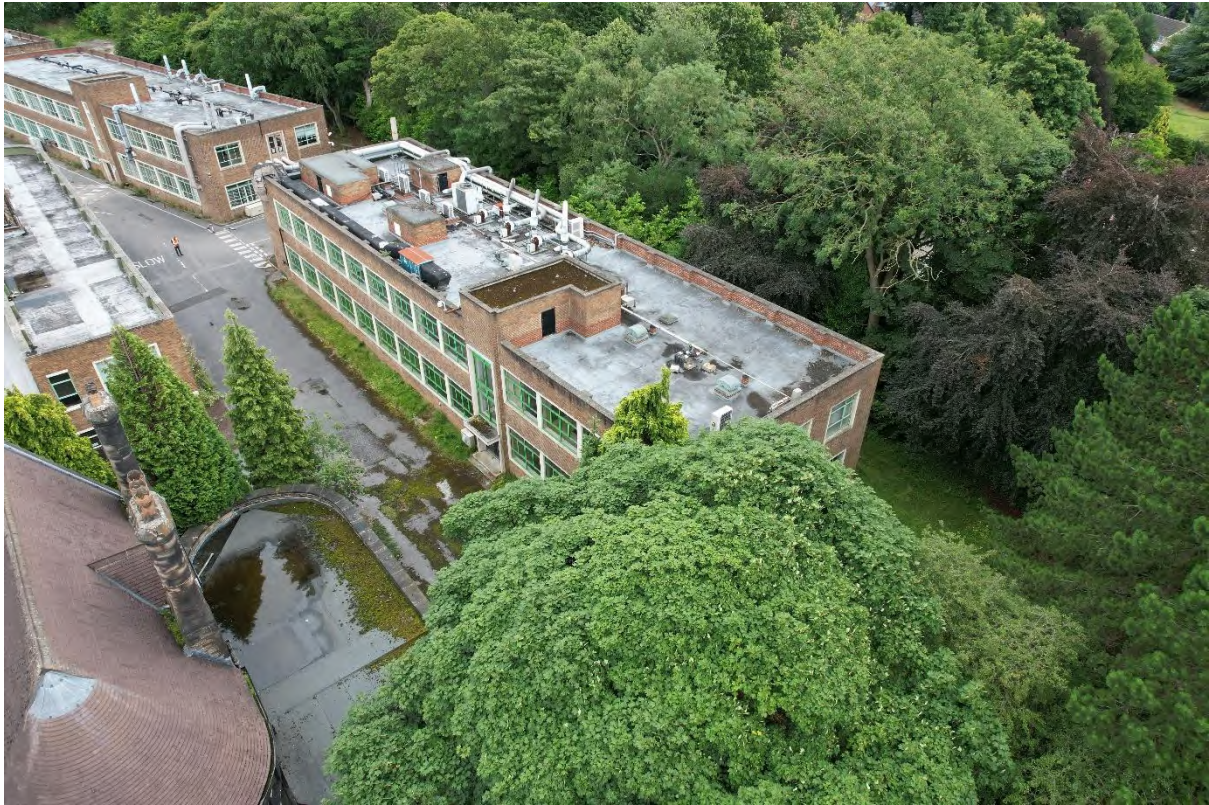
Plate 53. Block K from Drone (DJI_0172). Facing East.
