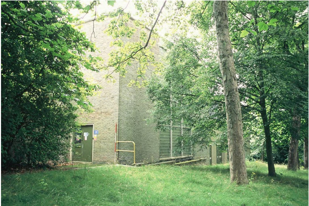
Plate 39. Block F: Exterior East and North Elevations (Swinden13_26). Facing West.
