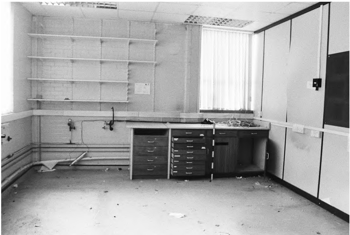
Plate 134. Block H: Interior Ground Floor Room H12D (Swinden3_09). Facing North.
