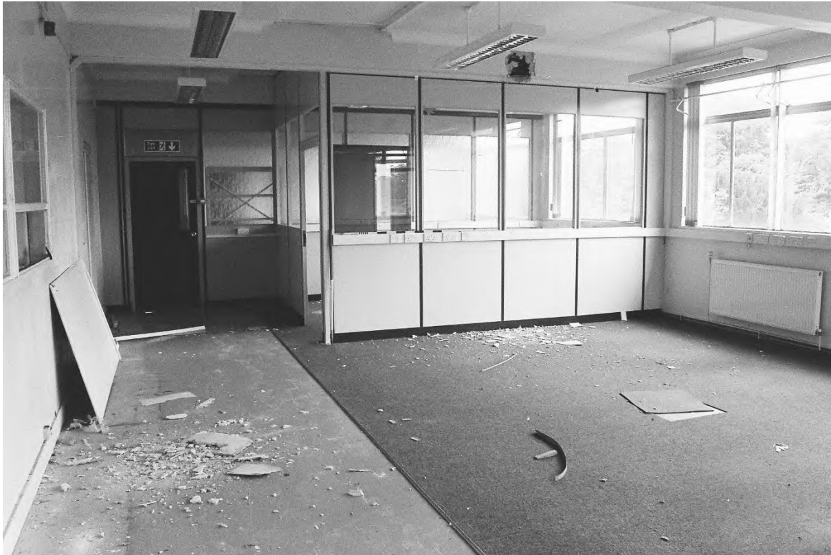
Plate 97. Block C: Interior Ground Floor Room C150/150D (Swinden11_37). Facing North.
