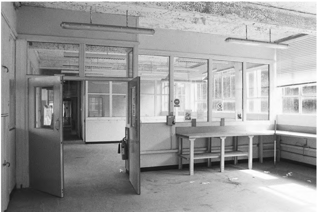
Plate 140. Block H: Interior First Floor Room H40 (Swinden3_20) Facing East.
