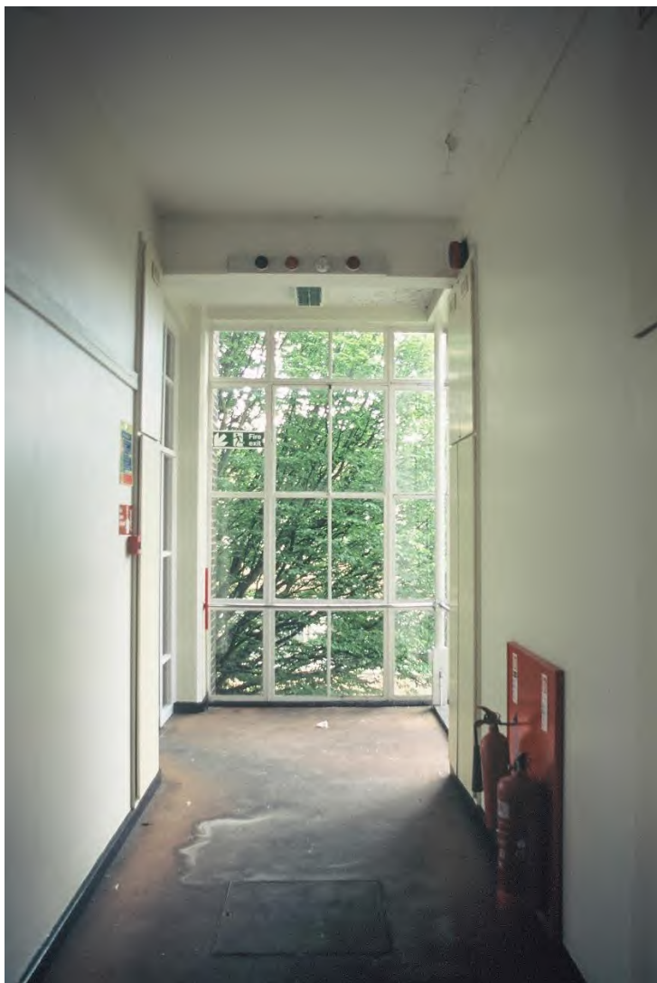
Plate 153. Block B: Interior First Floor Corridor (Swinden5_21). Facing South.
