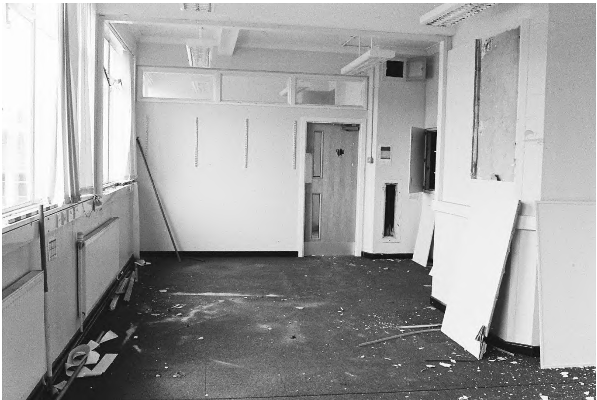
Plate 100. Block C: Interior Second Floor Room C156 (Swinden11_36). Facing North.
