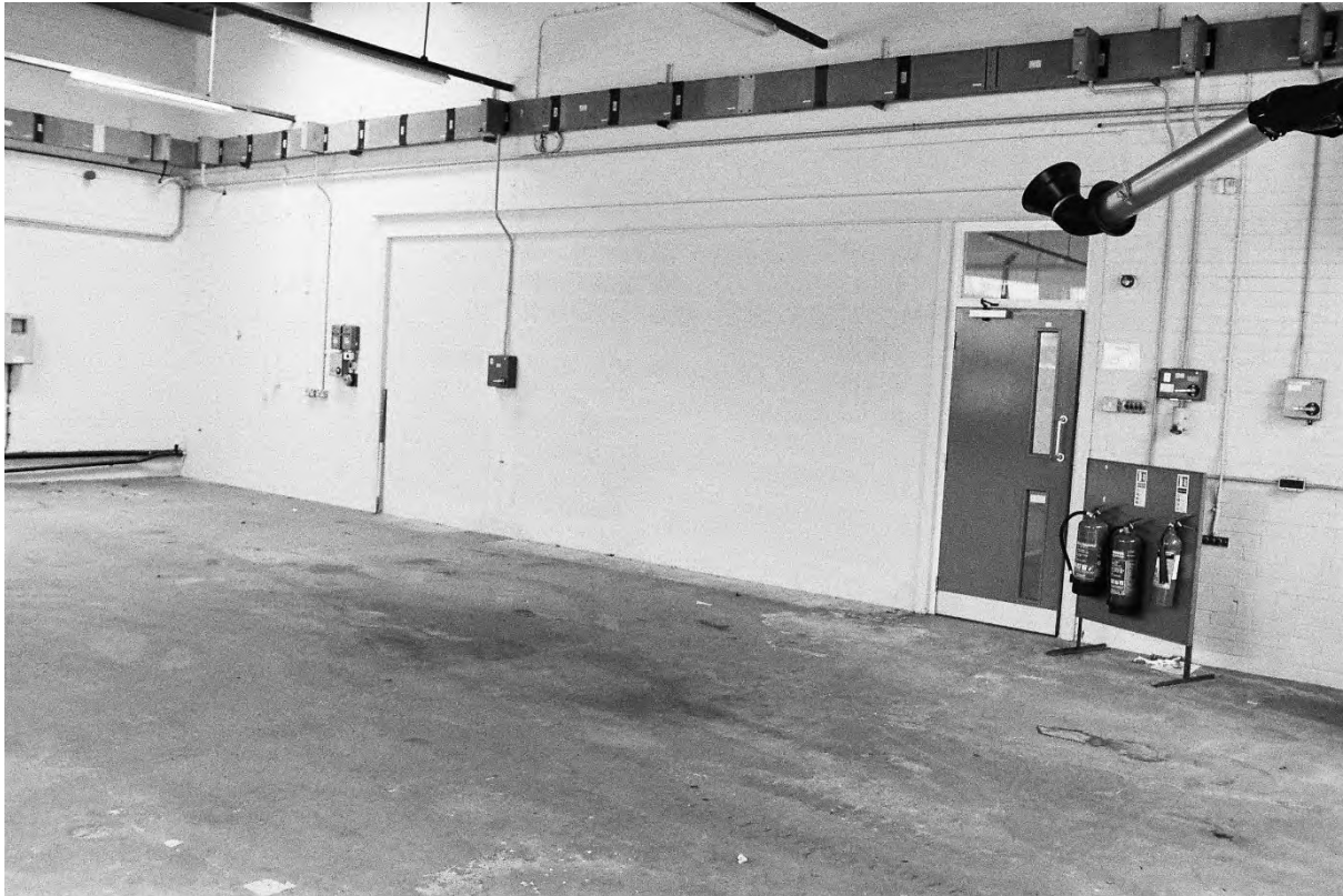
Plate 229. Block L: Interior Ground Floor Room L16 (Swinden8_20). Facing South-east.
