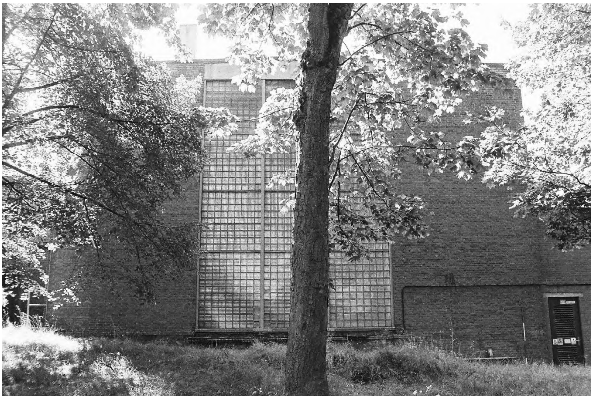
Plate 40. Block F: Exterior North Elevation (Swinden10_35). Facing South.
