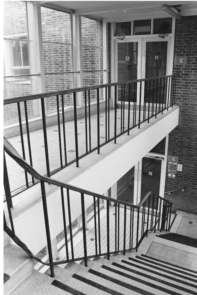
Plate 96. Blocks B & C: Interior First Floor Stairs (Swinden11/24). Facing North-west.
