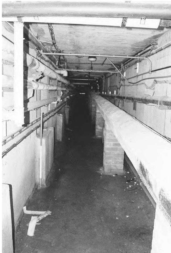
Plate 202. Block K: Interior Basement Duct (Swinden7_27). Facing East.
