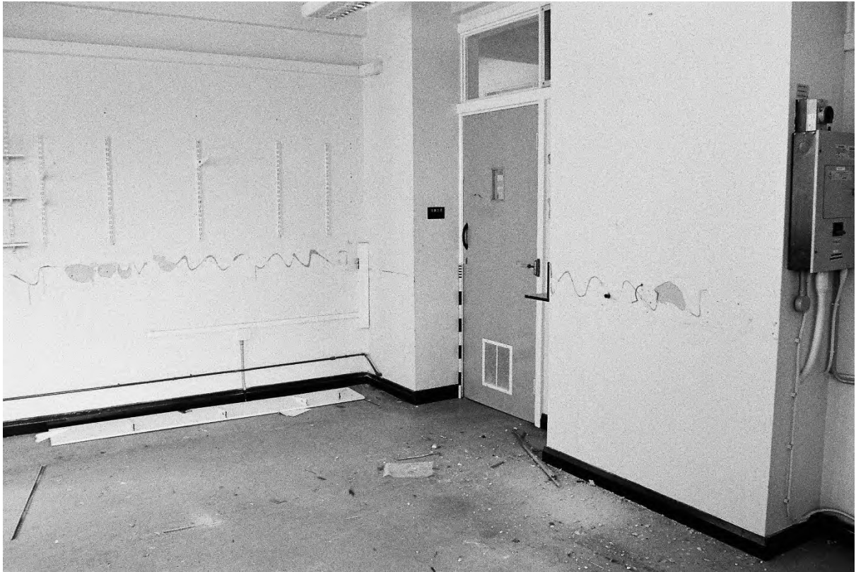
Plate 199. Block J: Interior First Floor J34 (Swinden7_10). Facing South-west.
