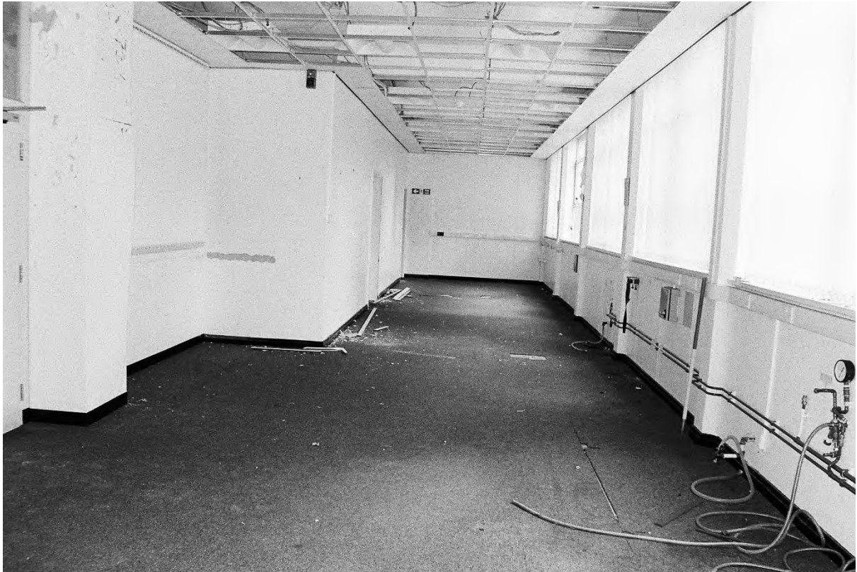
Plate 221. Block K: Interior First Floor Room K29/K37 (Swinden8_11). Facing East.
