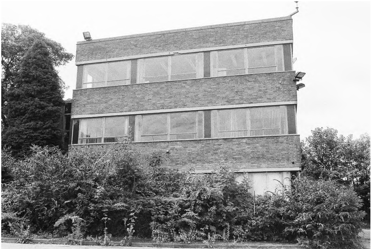
Plate 69. Block Q: External East Elevation (Swinden11_28). Facing West.
