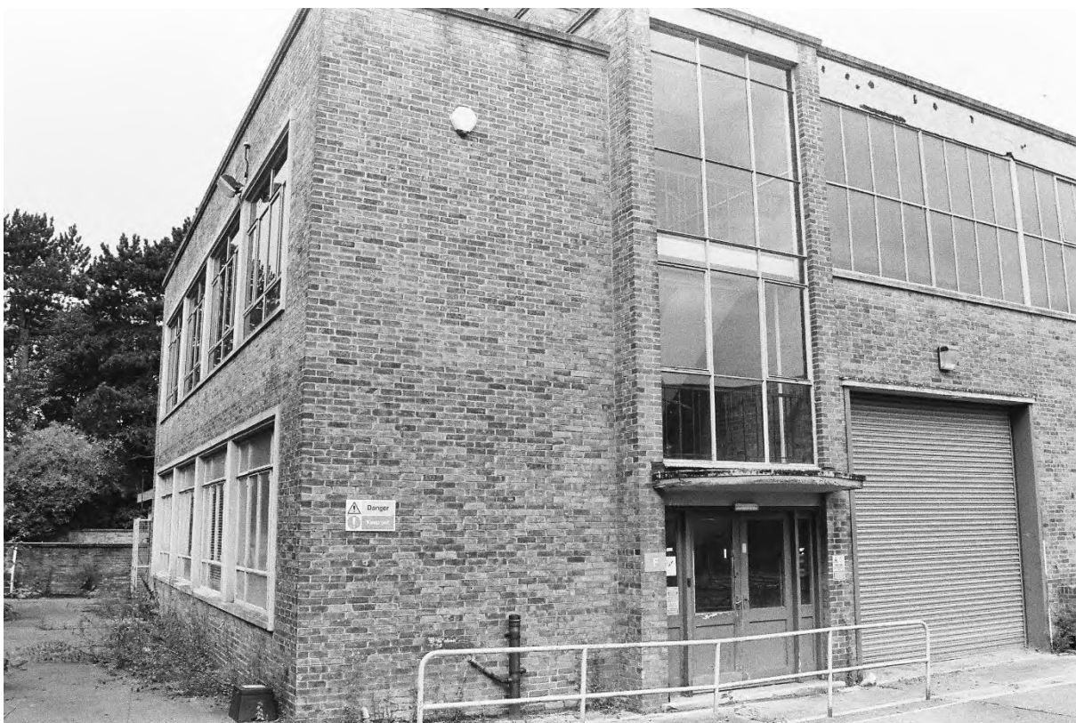
Plate 38. Block F: Exterior East & South Elevations (Swinden10_25). Facing West.
