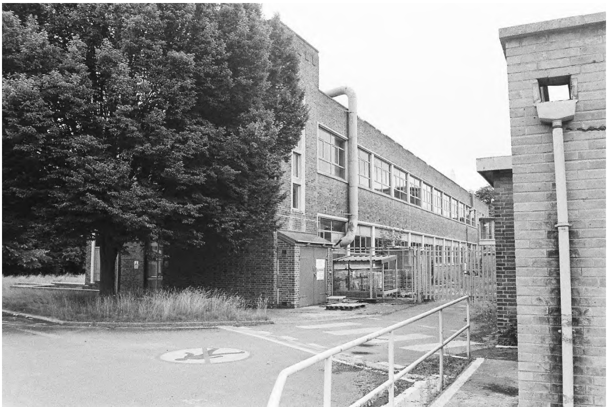
Plate 26. Block B: Exterior South Elevation (Swinden10_05). Facing North-east.
