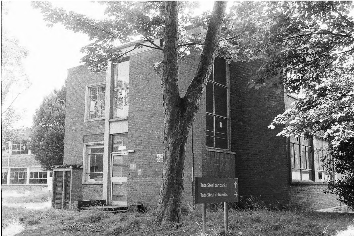
Plate 47. Block J: Exterior North & West Elevations (Swinden11_02). Facing South-east.
