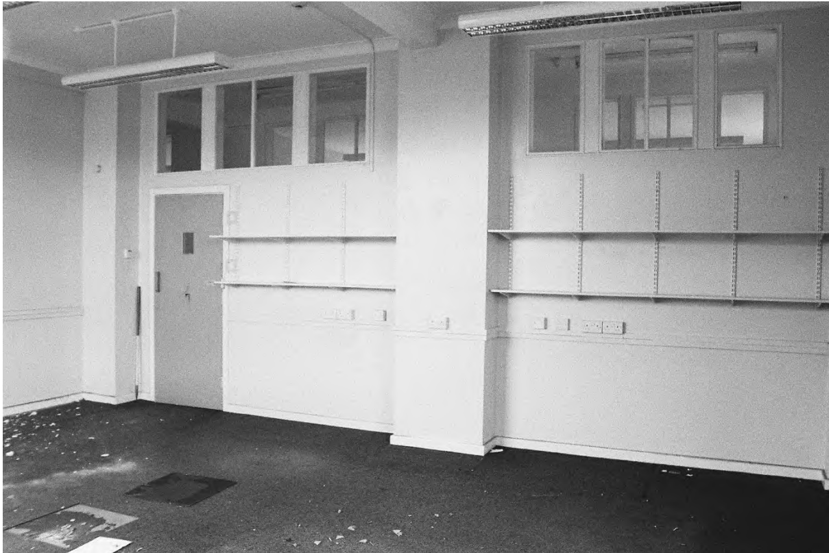
Plate 121. Block A: Interior First Floor Room A54 (Swinden2_24). Facing South-east.
