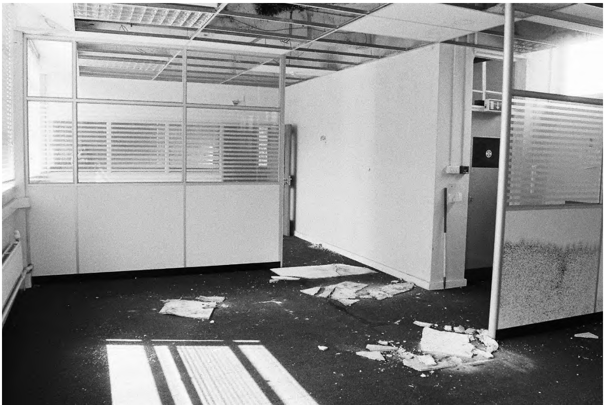
Plate 242. Block L: Interior First Floor Room L28 (Swinden8_18). Facing West.
