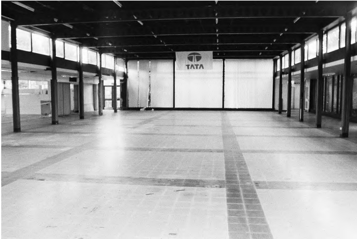
Plate 259. Canteen: Interior (Swinden6_05). Facing South.
