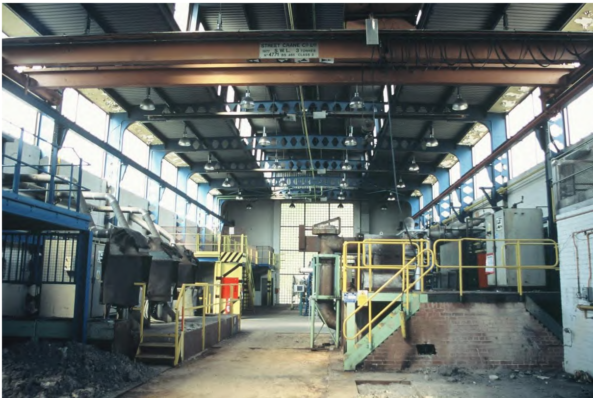
Plate 172. Block F: Interior Ground Floor Room F8/F10 (Swinden12_01). Facing North.
