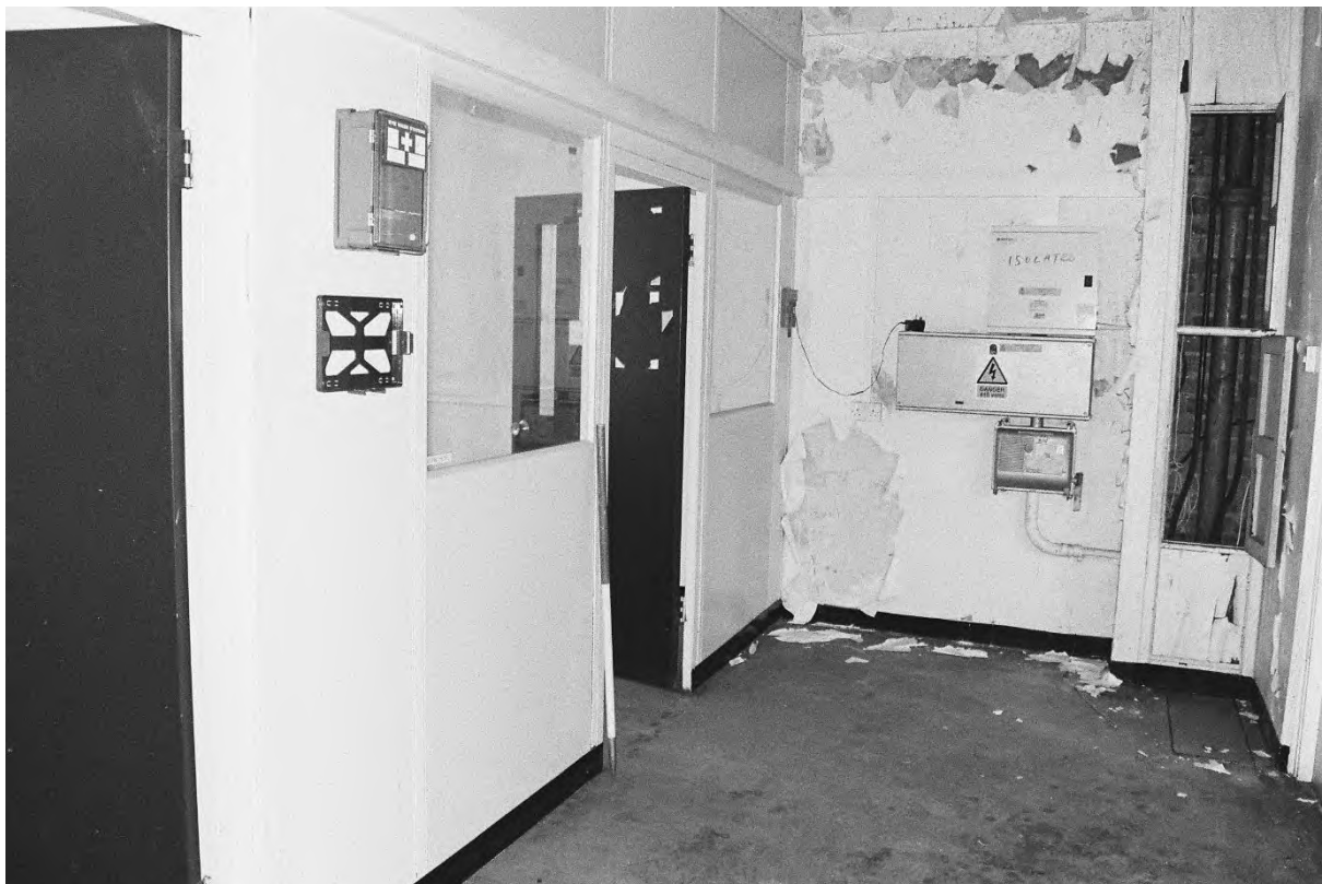
Plate 176. Block F: Interior Ground Floor Room F7 (Swinden6_19). Facing South-west.
