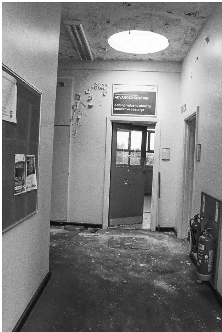
Plate 152. Block B: Interior First Floor Corridor & Skylight (Swinden3_30). Facing North.
