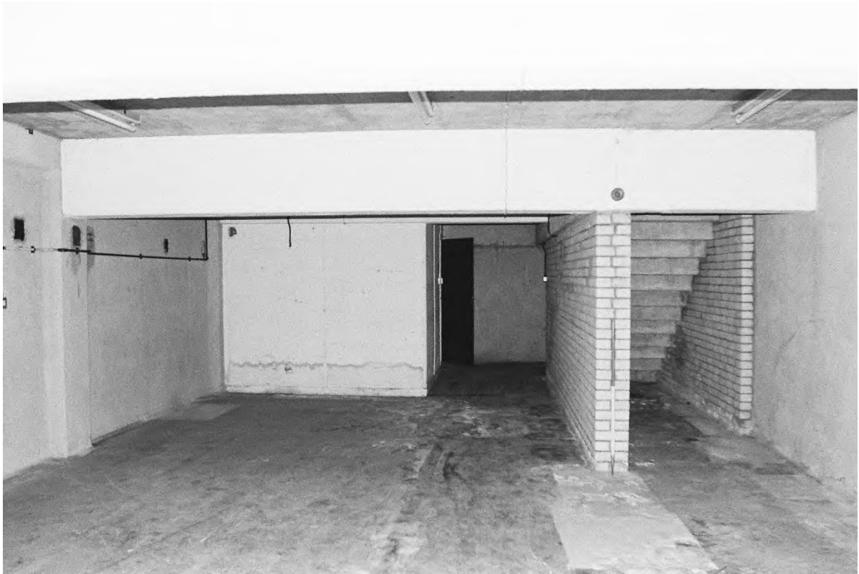
Plate 227. Block L: Interior Basement Room L31 (Swinden8_34). Facing West.
