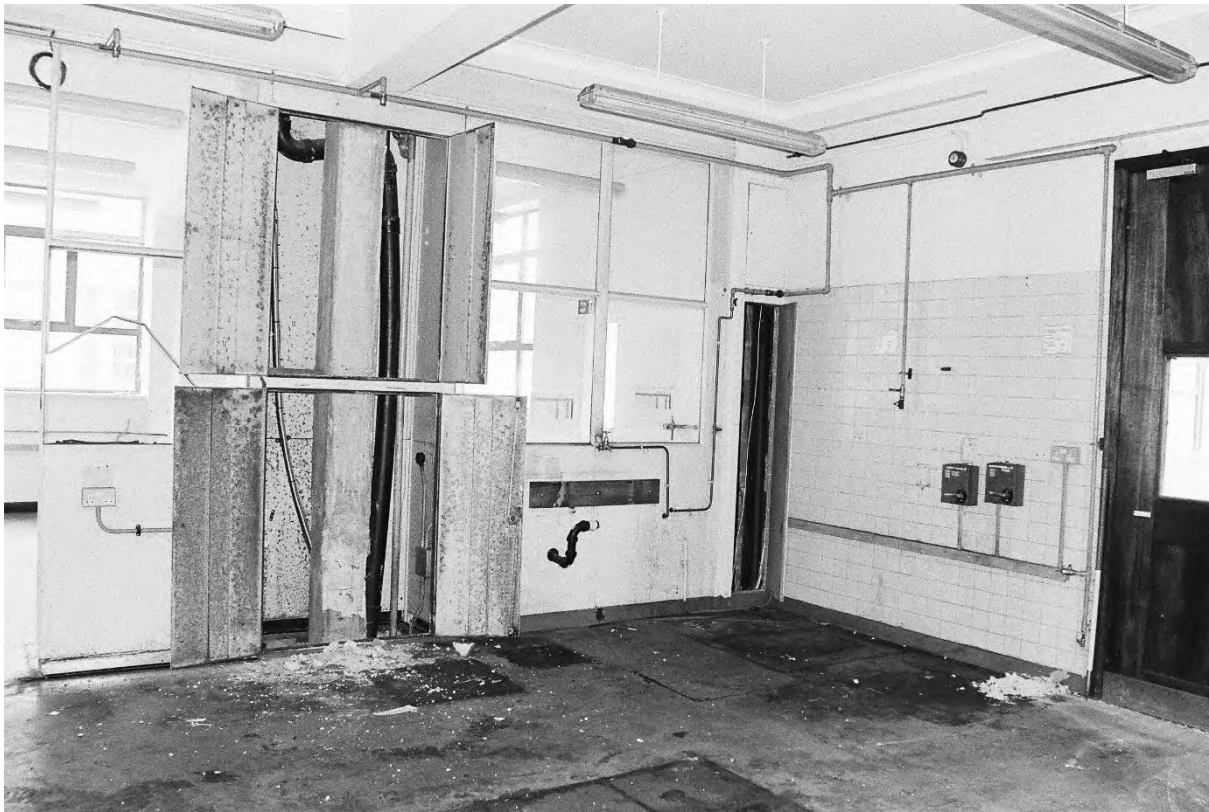
Plate 207. Block K: Interior Ground Floor Room K1 (Swinden8_04). Facing North-east.
