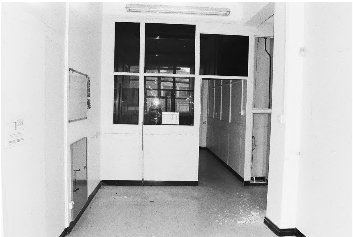
Plate 212. Block K: Interior Ground Floor Corridor & Room K9 (Swinden8_02). Facing South.
