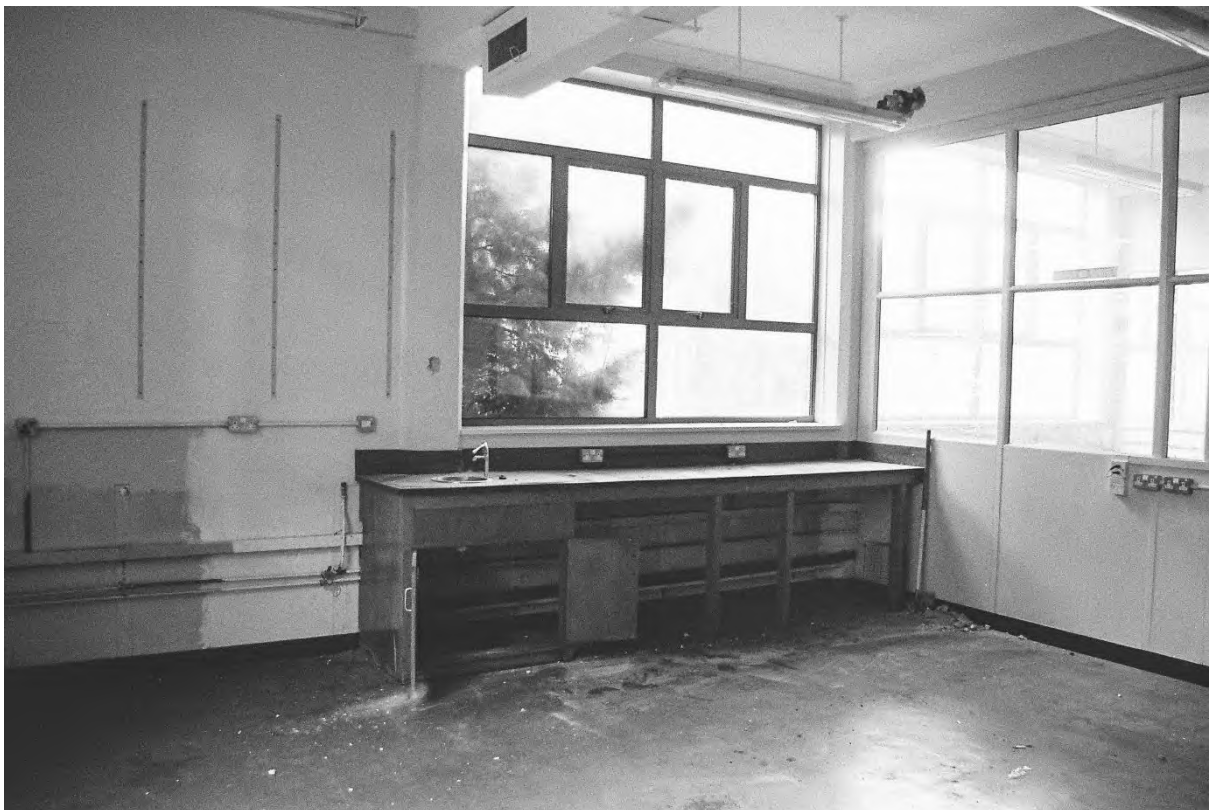
Plate 216. Block K: Interior Ground Floor Room K18 (Swinden7_31). Facing North-east.
