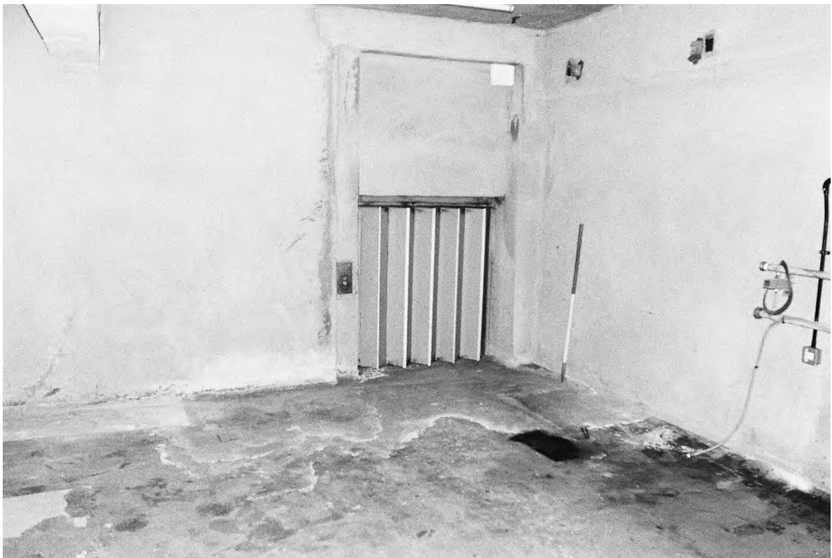
Plate 226. Block L: Interior Basement Room L31 Goods Elevator (Swinden8_33). Facing North.
