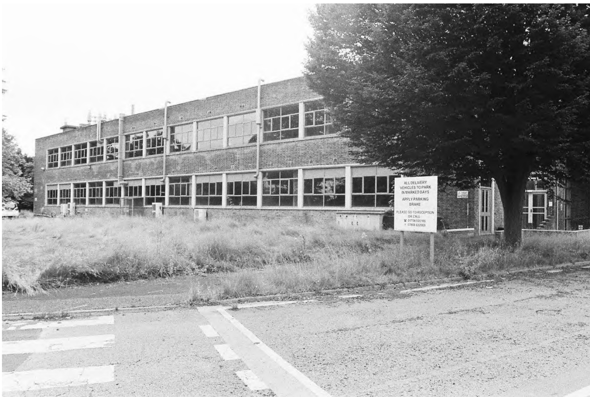
Plate 20. Block B: Exterior North Elevation (Swinden10_07). Facing South-east.
