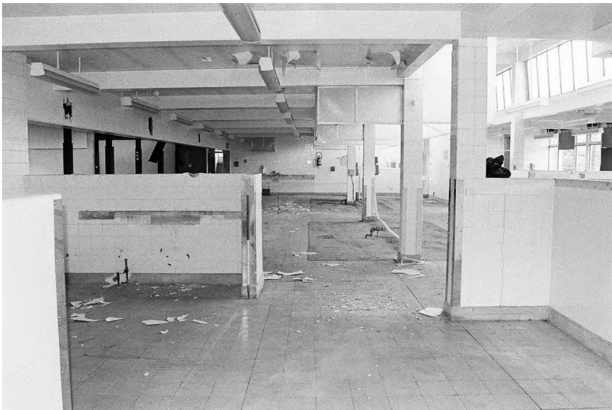
Plate 262. Canteen: Interior (Swinden6_08). Facing North.
