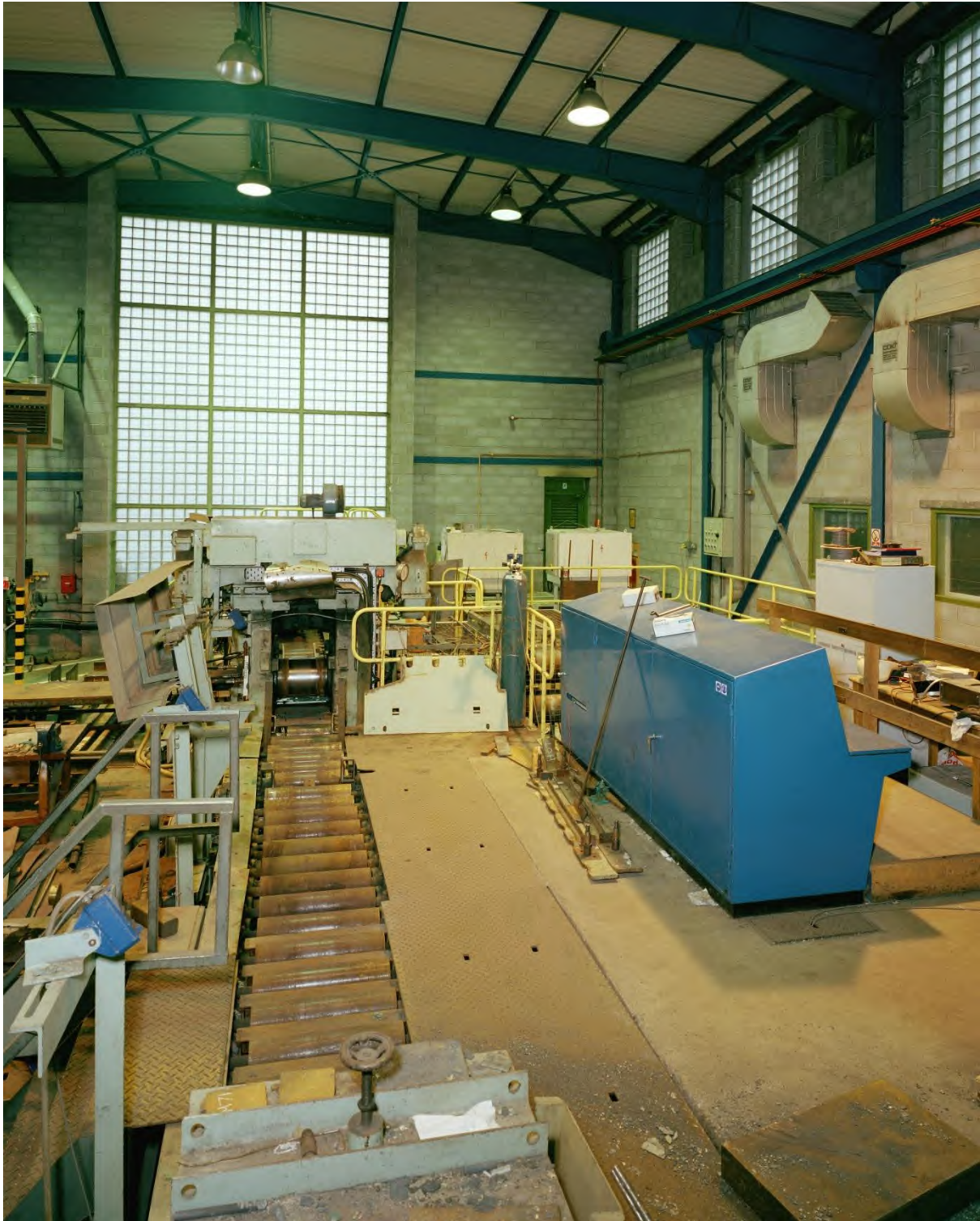
AA040592 G Block extension - experimental rolling mill (copyright Historic England Archive 2002)
