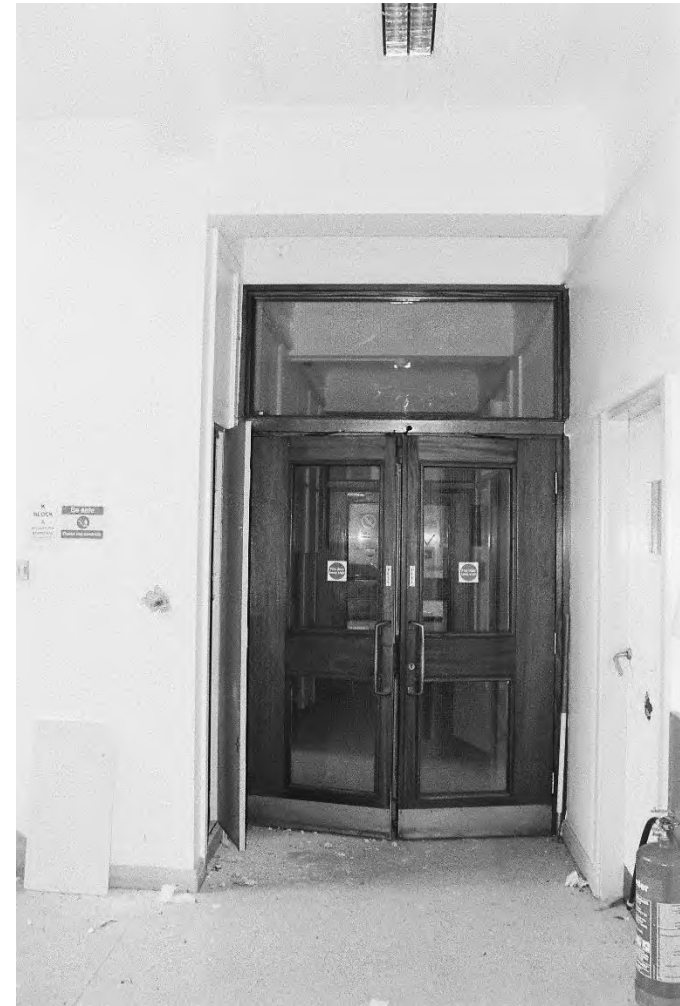
Plate 206. Block K: Interior Ground Floor Corridor (Swinden7_33). Facing East.
