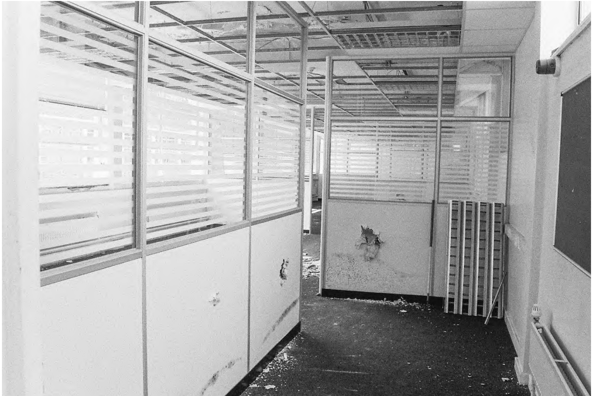
Plate 241. Block L: Interior First Floor (Swinden8_17). Facing West.
