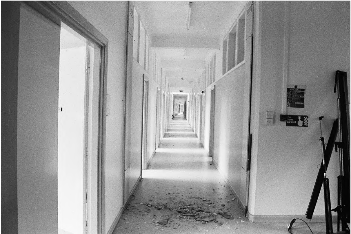
Plate 115. Block A: Interior First Floor Corridor (Swinden2_14). Facing West.
