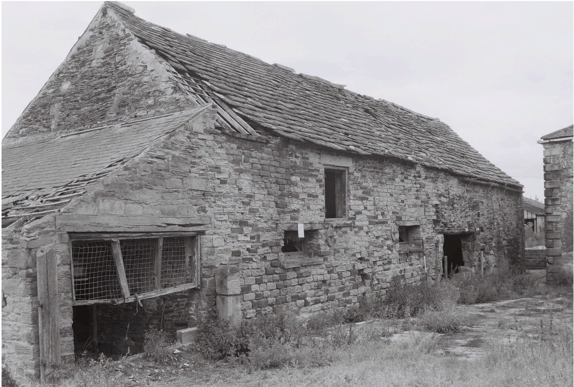
Plate15. South Barn: South Elevation. Facing North-east.
