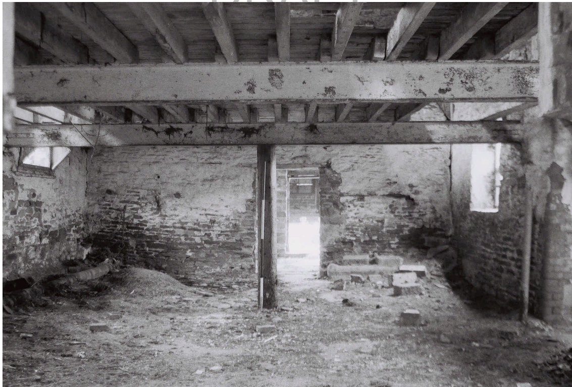
Plate 20. South Barn: Interior. Facing East.
