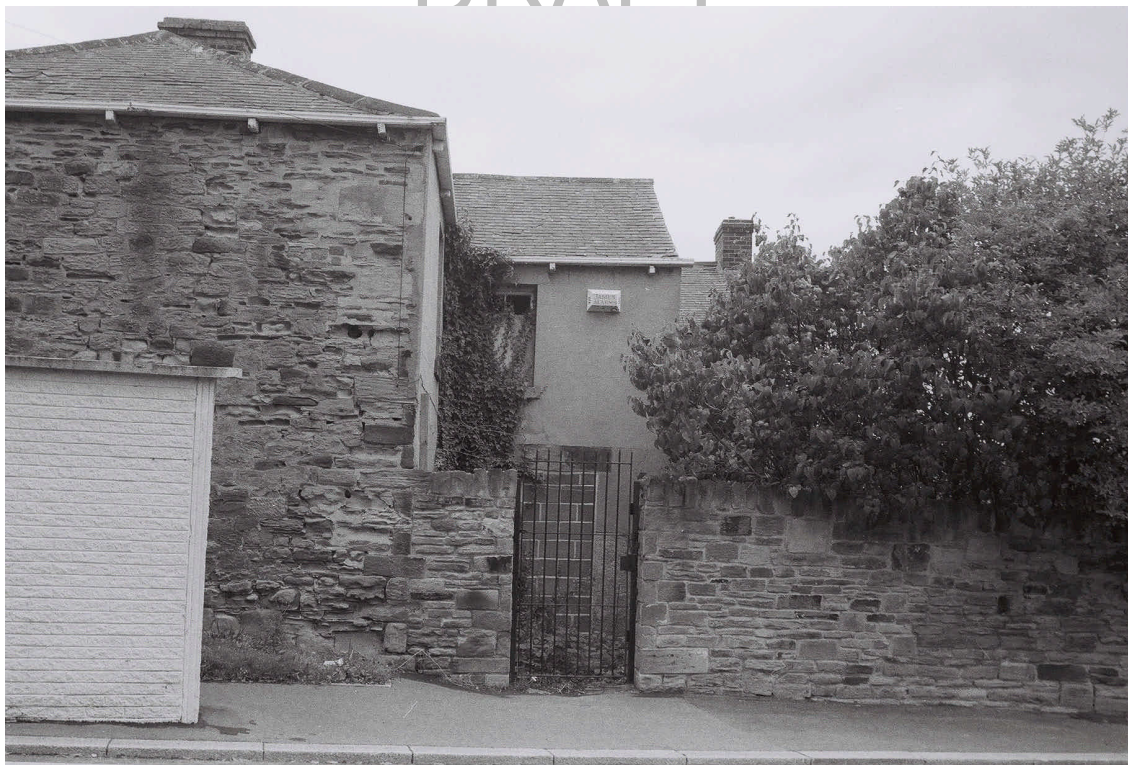
Plate 6. Manor House: South Elevation. Facing North.
