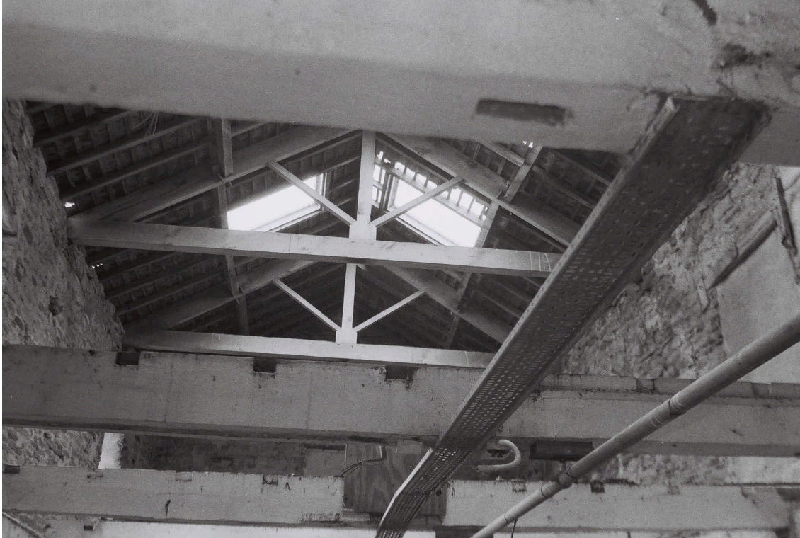
Plate 41. East Barn: Interior. Facing South.
