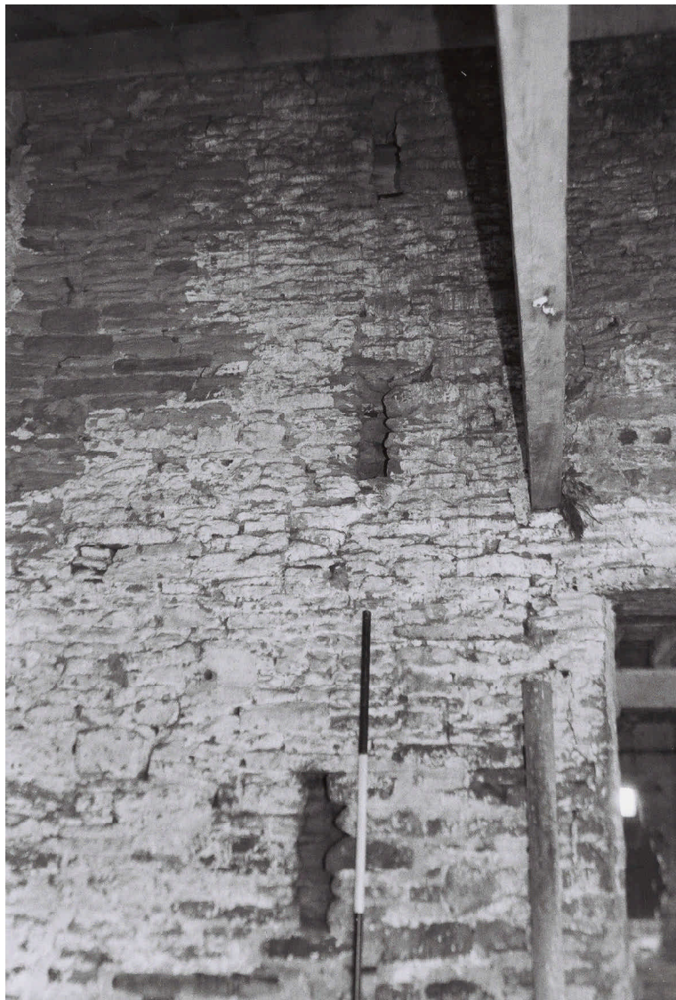
Plate 22. South Barn: Interior. Facing East.
