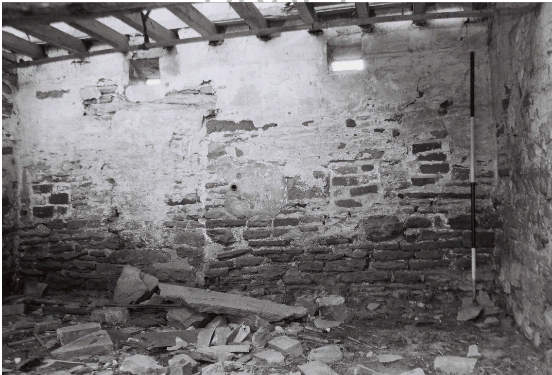
Plate 30. East Barn: Interior. Facing West.
