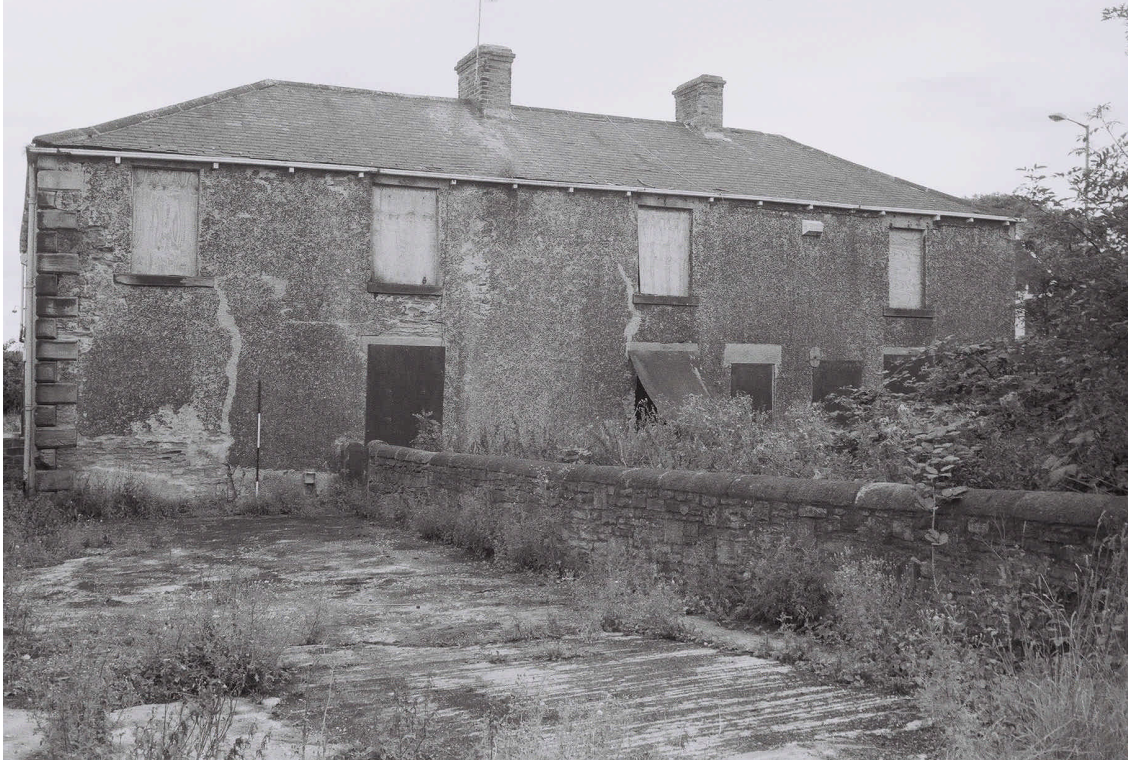
Plate 7. Manor House: West Elevation. Facing East.
