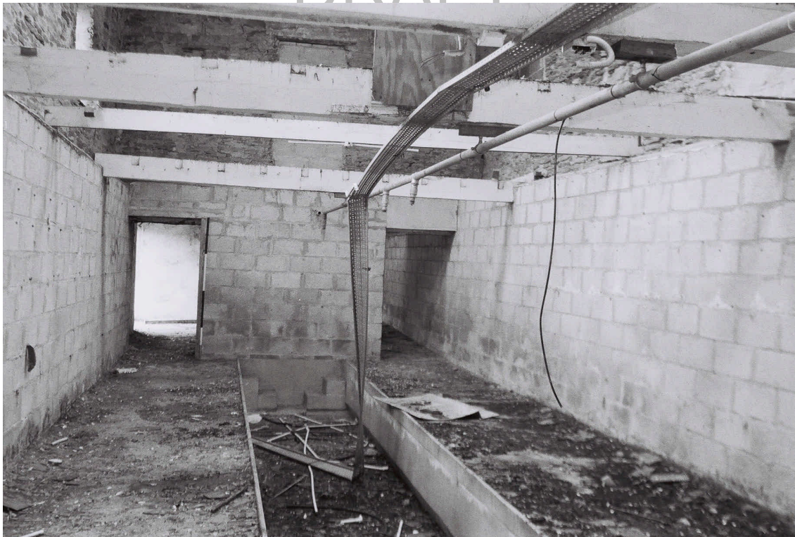
Plate 40. East Barn: Interior. Facing South.
