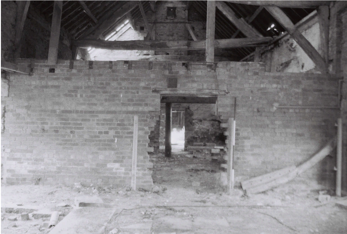
Plate 19. South Barn: Interior. Facing West.
