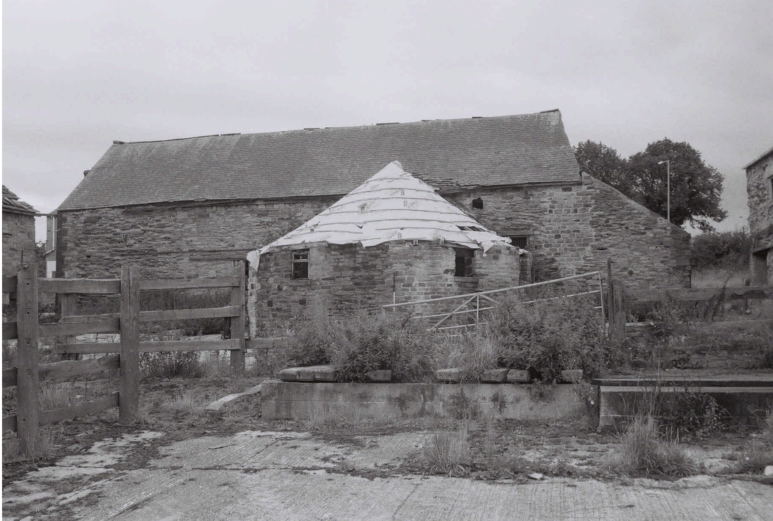
Plate 11. South Barn and Horse Engine House: North Elevation. Facing South.
