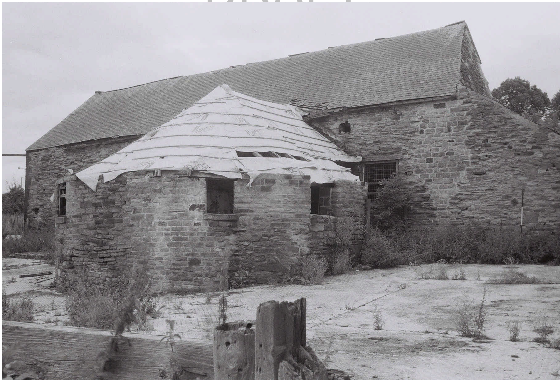
Plate 12. South Barn and Horse Engine House: North Elevation. Facing South-east.
