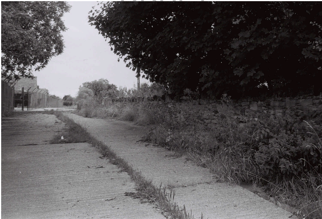
Plate 4. Wall to Cinderbridge Plantation. Facing West.
