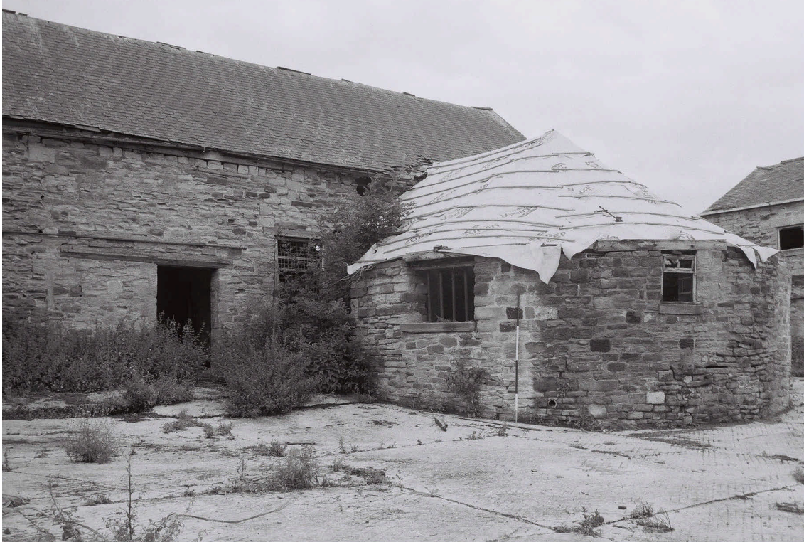
Plate 13. South Barn and Horse Engine House: North Elevation. Facing Southwest.
