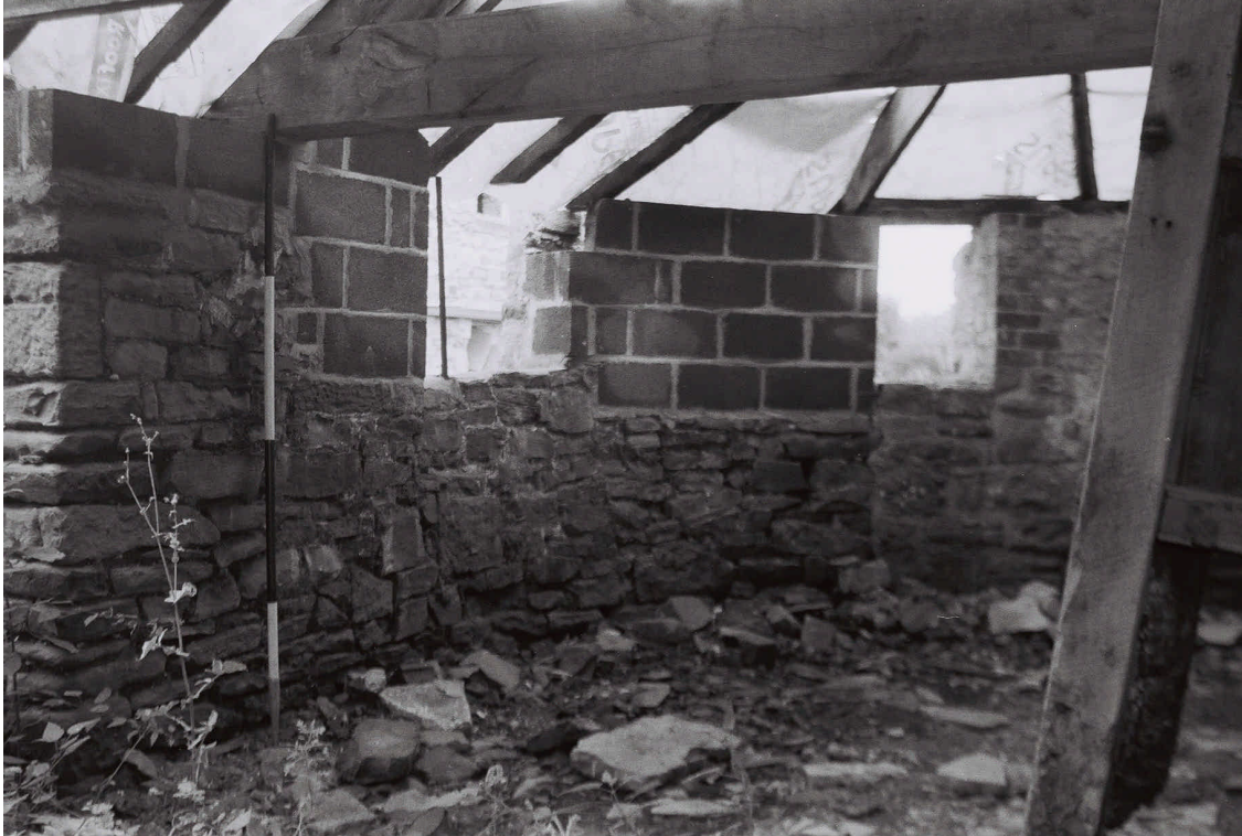
Plate 23. Horse Engine House: Interior. Facing North.
