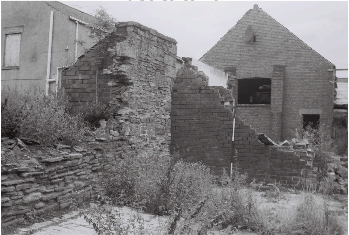
Plate 14. South Barn: East Elevation. Facing West.
