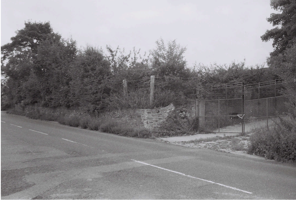
Plate 1. Boundary Wall on Church Street. Facing North-west.
