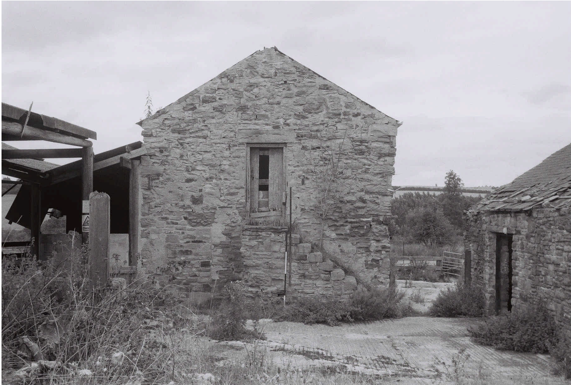
Plate 37. West Barn: South Elevation. Facing North.
