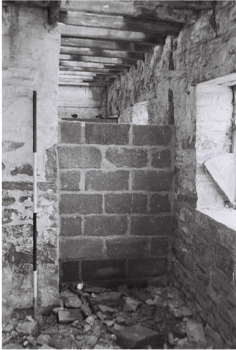
Plate 31. East Barn: Interior. Facing South.
