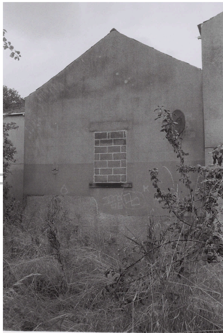
Plate 10. Manor House. East Elevation. Facing West.
