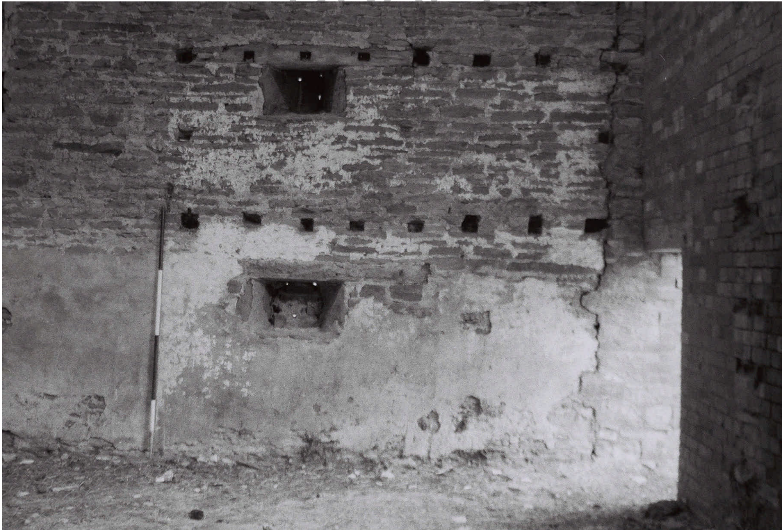
Plate 18. South Barn: Interior. Facing North.
