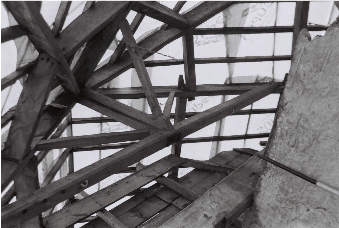
Plate 25. Horse Engine House: Interior. Facing South-west.
