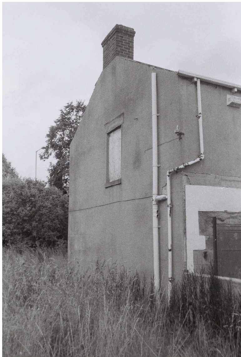
Plate 9. Manor House. East Elevation. Facing West.
