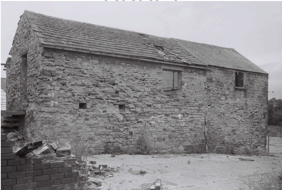
Plate 28. East Barn: East Elevation. Facing West.
