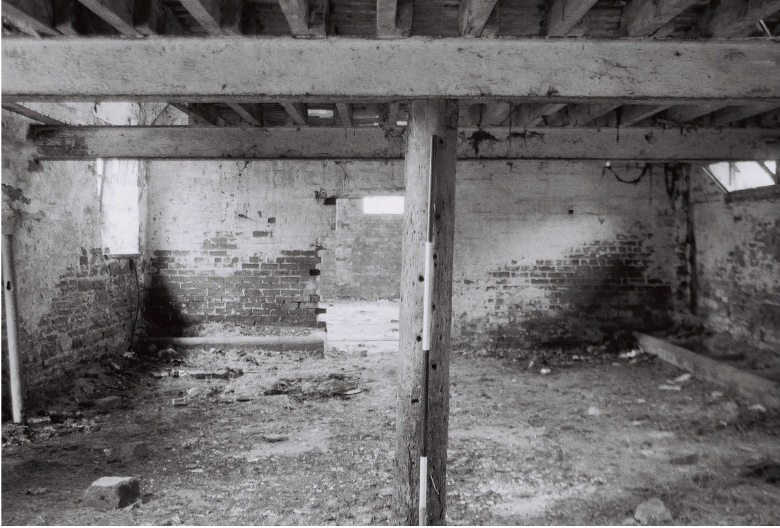
Plate 21. South Barn: Interior. Facing West.
