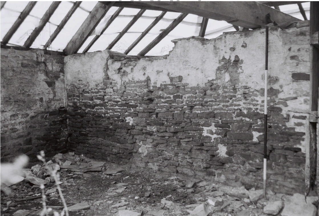
Plate 24. Horse Engine House: Interior. Facing North.
