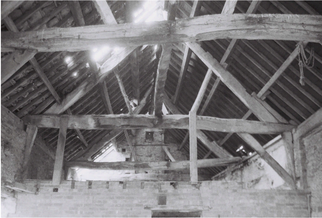
Plate 17. South Barn: Interior. Facing West.
