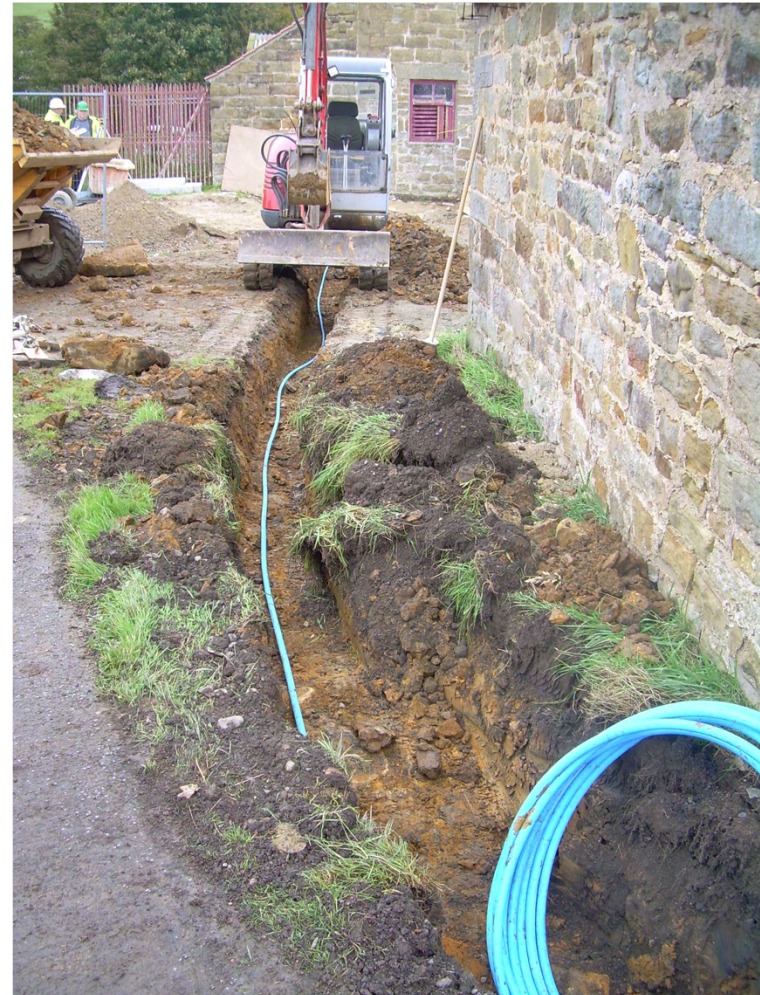
Plate 6. Trench for water pipe. facing North.
