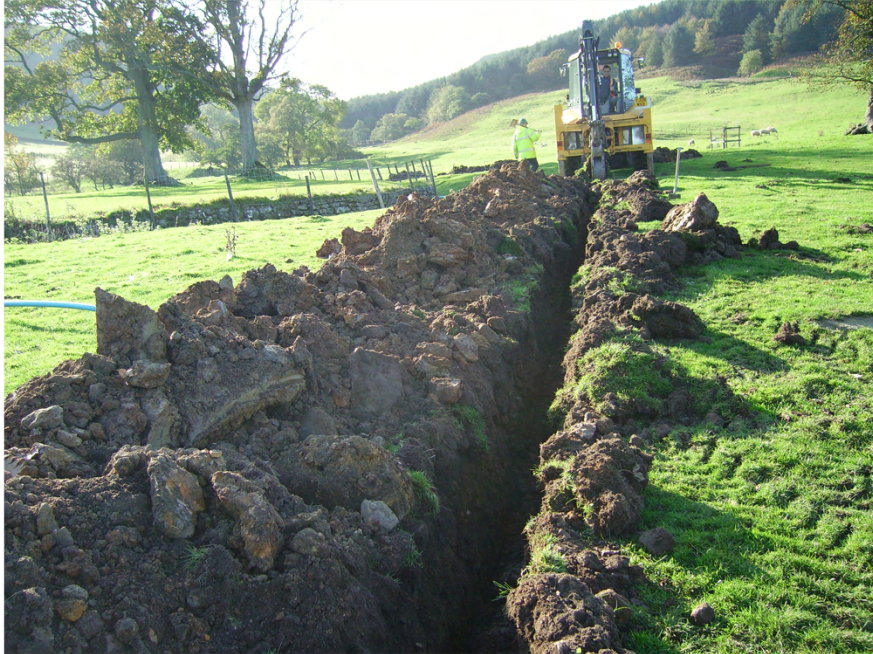
Plate 7. Trench through Field 0062. Facing South-west.
