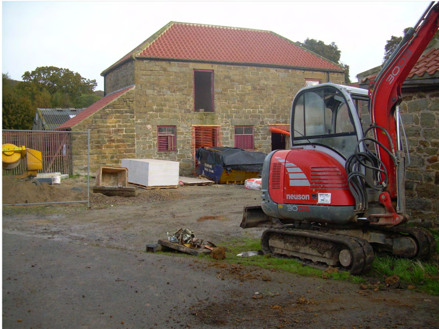
Plate 3. View of Barn. Facing North-east.
