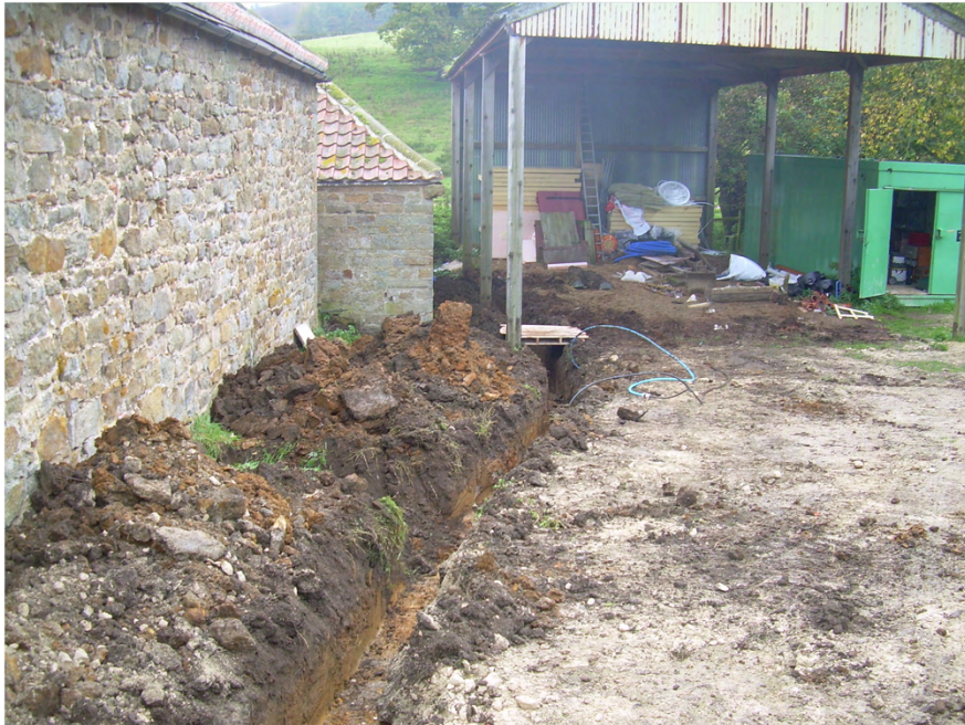
Plate 5. Trench for water pipe. Facing West.
