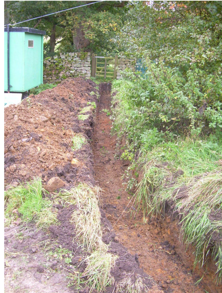
Plate 4. View of water pipe trench. Facing South.
