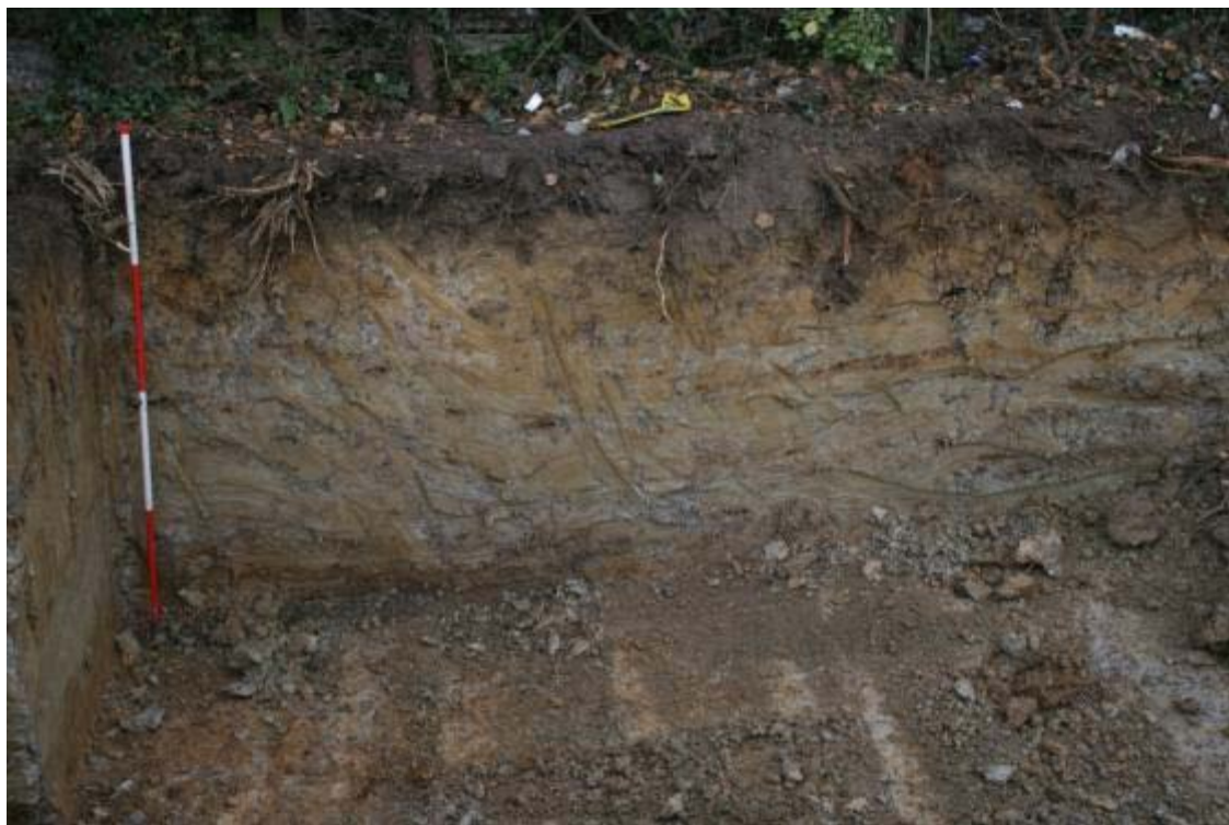
Fig. 7: Land at Burtenshaw Lane, Market Street, Hailsham: Photograph of road and water storage facility excavation
