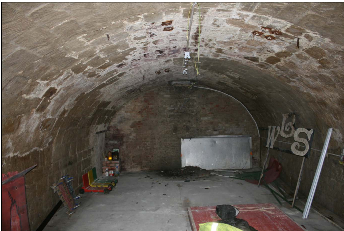
Fig. 20: 190 High Street, Lewes: Cellar/Basement
