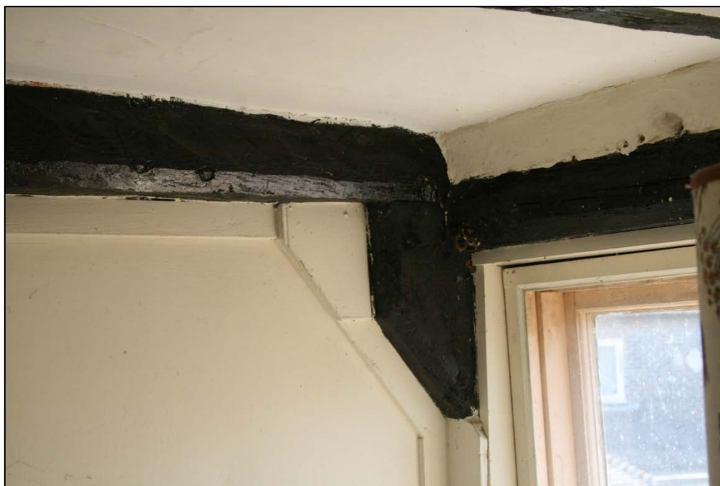
Fig. 10: Crown Cottages: Exposed beam and wall plate on the landing
