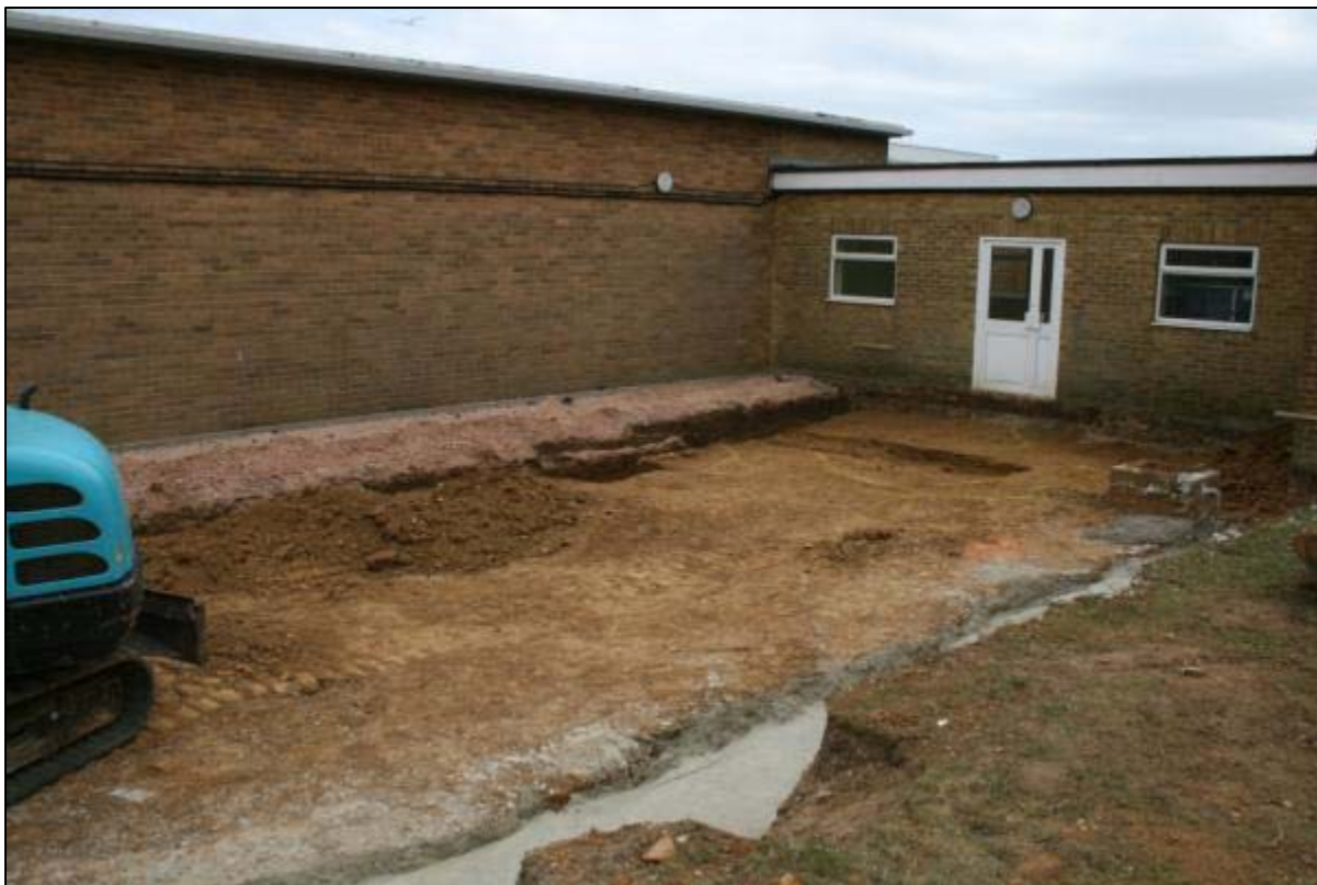
Fig. 14: Tideway School, Newhaven: General view of south end of site
