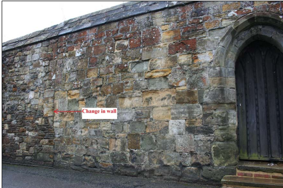
Fig. 7: Upper Lake Zebra Crossing: Photograph showing the change in precinct wall construction
