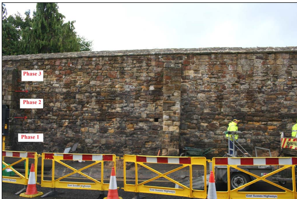
Fig. 8: Upper Lake Zebra Crossing: Photograph showing the different phases of precinct wall construction
