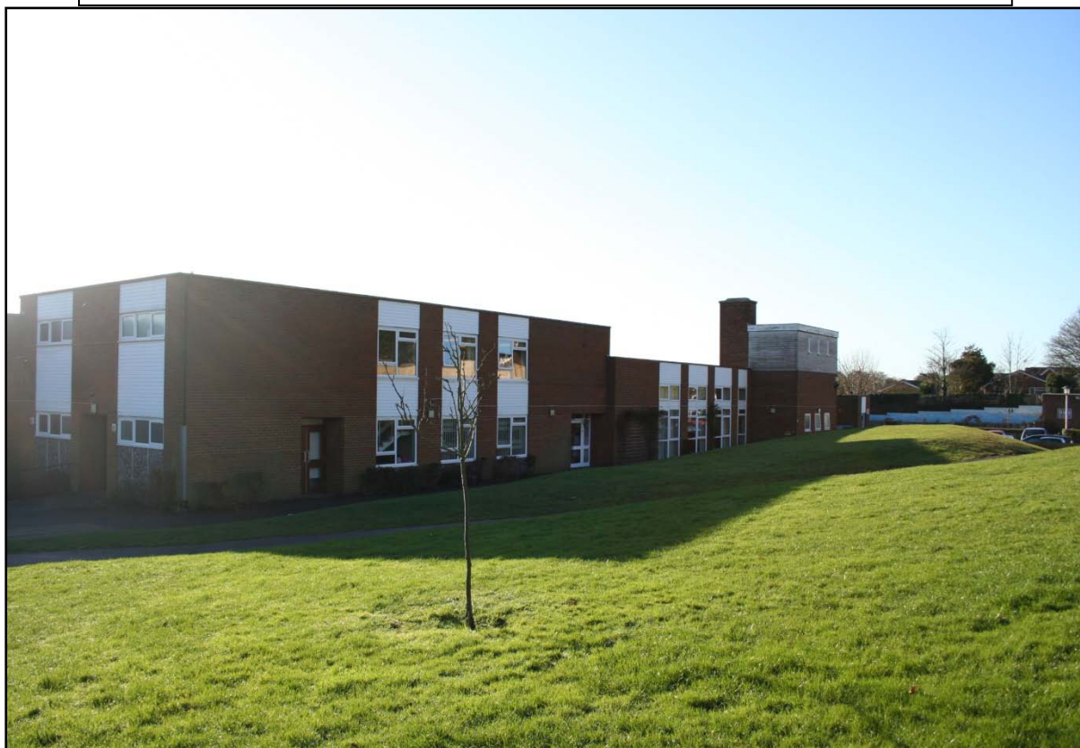
Fig. 14: Cradle Hill School, Seaford: Site of proposed extension on north side
