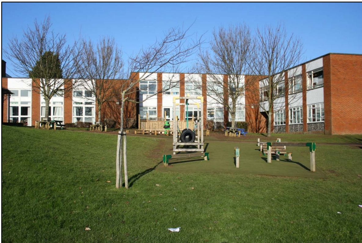
Fig. 13: Cradle Hill School, Seaford: Site of proposed extension on south side
