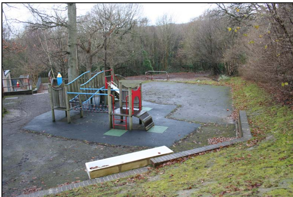
Fig. 12: Churchwood School: NW side of school showing the terracing into the slope at different levels
