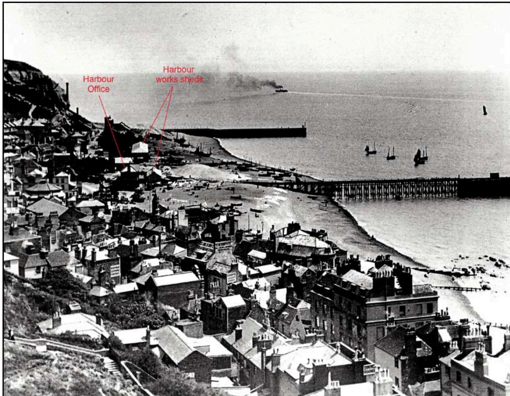
Fig. 24: The Stade: 1897/8 showing the harbour arm under construction 000.62.79 Courtesy of Hastings Museum and Art Gallery
