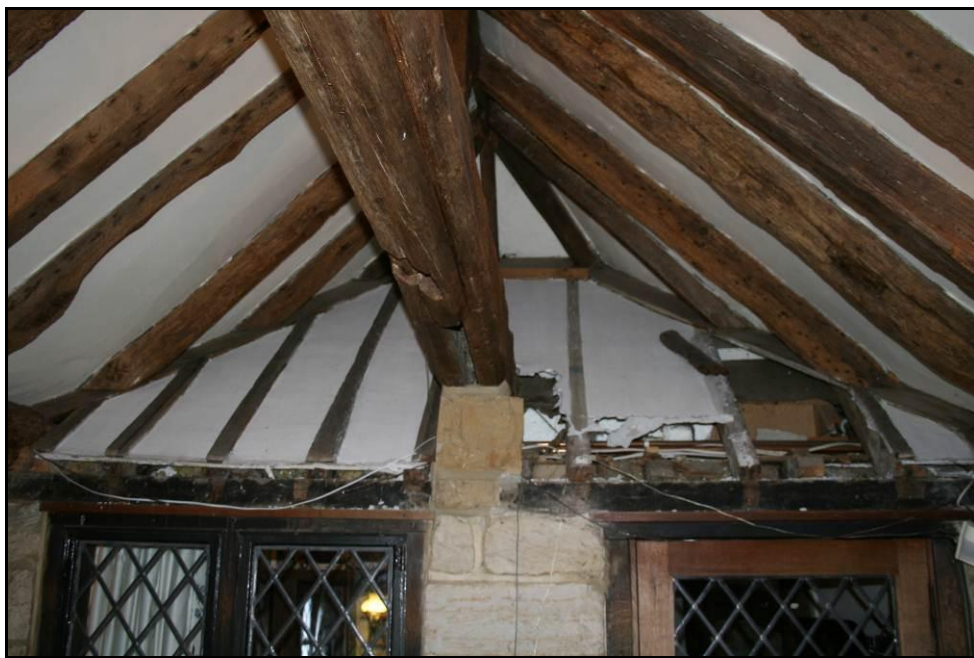
Fig. 8: Parrock Brook, Hartfield: Reused timbers in existing extension
