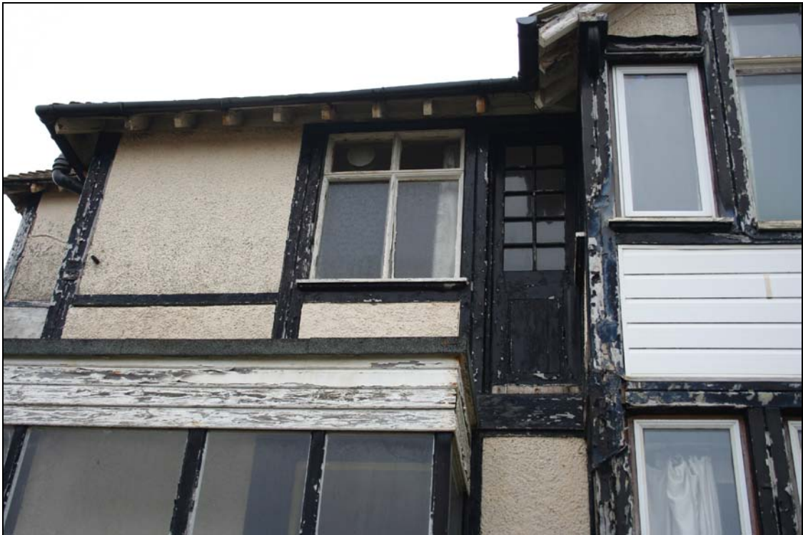
Fig. 17: 1 Cricketfield Road, Seaford: External view of balcony area
