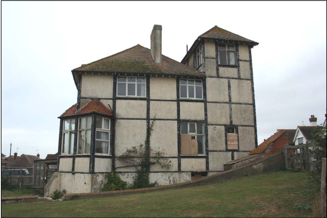
Fig. 11: 1 Cricketfield Road, Seaford: View of the house from the east
