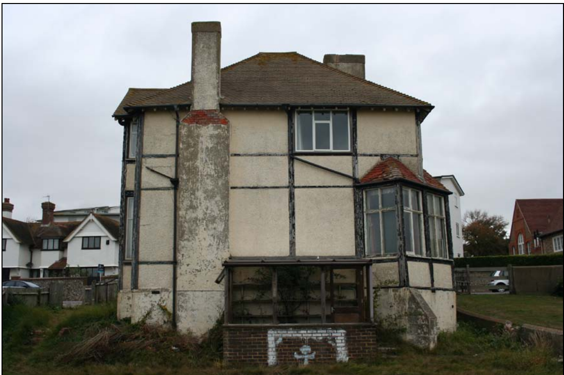
Fig. 14: 1 Cricketfield Road, Seaford: View of the house from the south
