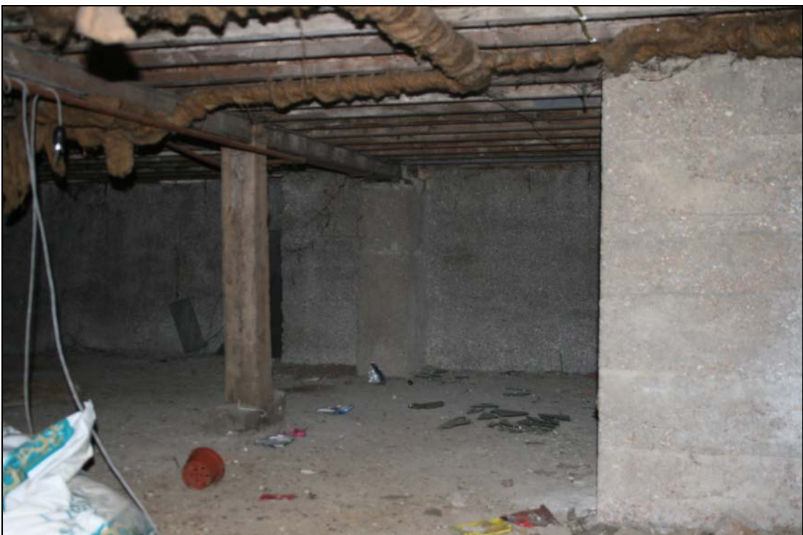
Fig. 18: 1 Cricketfield Road, Seaford: The basement
