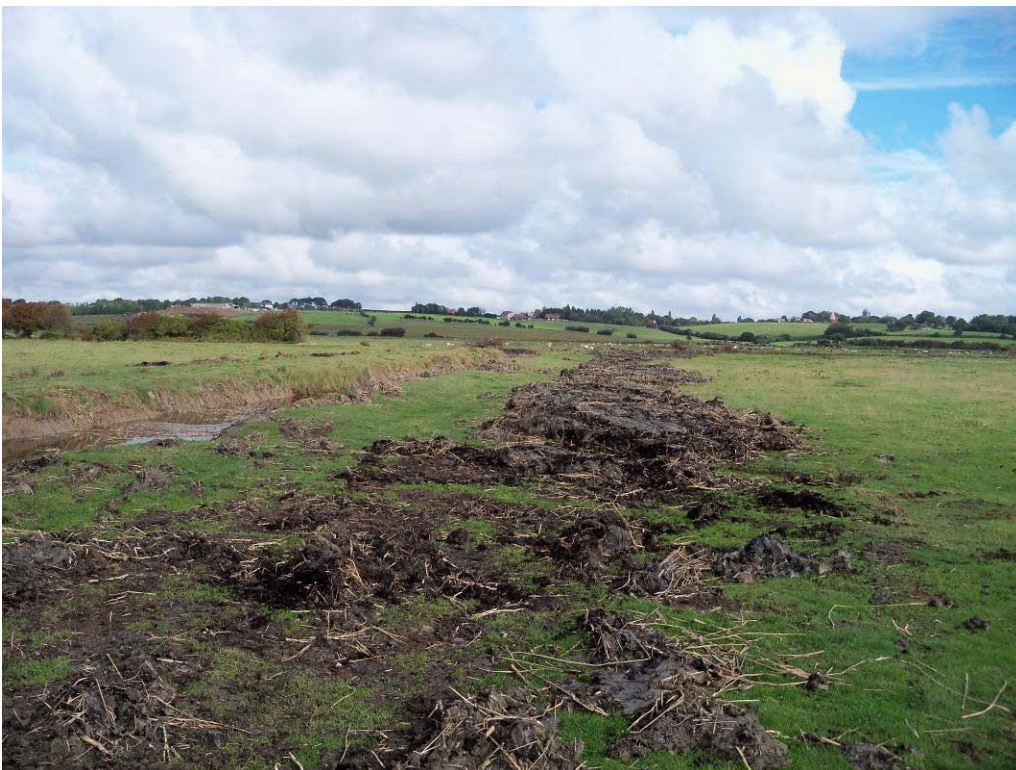
Plate 2. Up Cast Spoil from Drainage Channel P.1 to P.2
